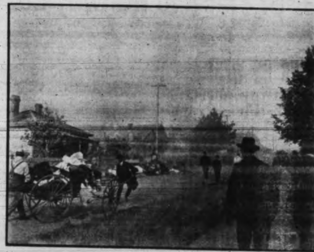
LOOKING UP PRINCESS AVENUE. HOUSES ON THE NORTH SIDE IN FLAMES.
