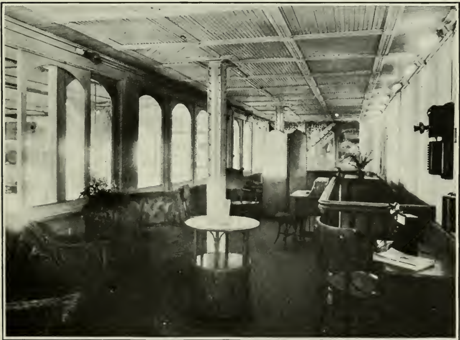
FIG. 2.—REST ROOM PROVIDED BY A CITY MARKET IN WASHINGTON, D. C.
