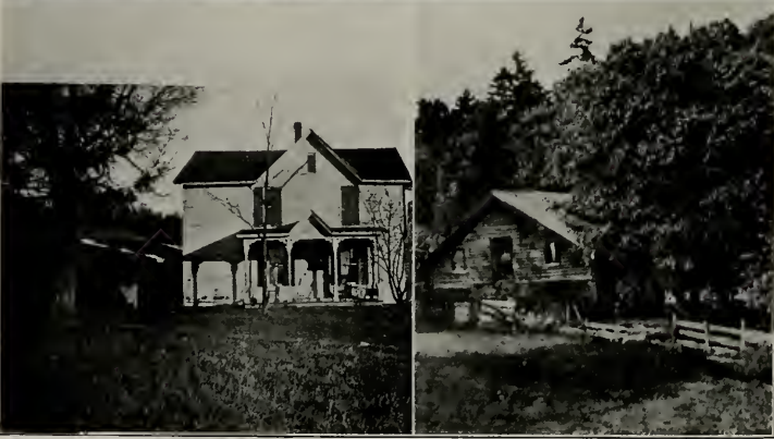
REAR VIEW OF OLD MILL HOUSE (BUILT IN 1810)
