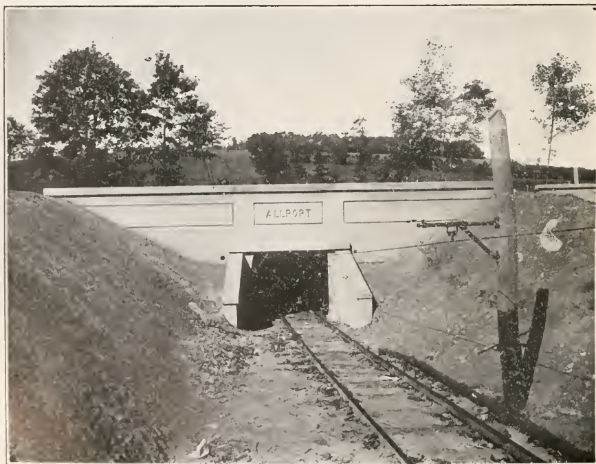
PLATE IV. ENTRANCE TO ALLPORT MINE. ALL CONCRETE. NO TIMBERS TO CATCH FIRE AND SPREAD THROUGHOUT THE MINE
