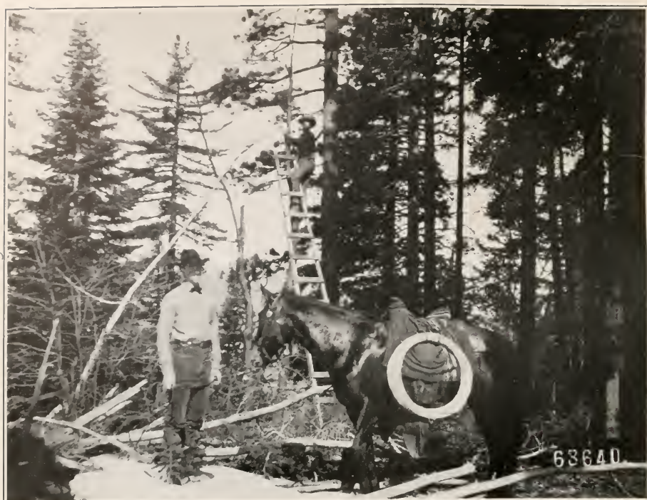
RANGERS CONSTRUCTING TELEPHONE LINES, PLUMAS NATIONAL FOREST, CALIFORNIA
