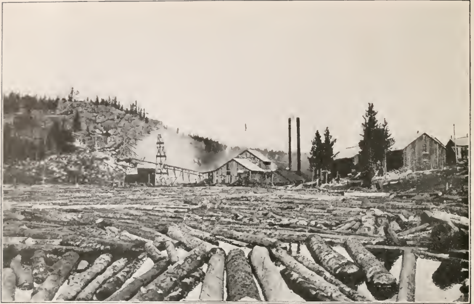
No. 5. THE LOG POND OF A SMALL SAWMILL, LOCATED WITHIN THE BOUNDARIES OF THE FOREST. TIES, SMALL LOGS AND LARGE SLABBED LOGS ARE FLUMED TO THE LARGER MILL IN THE VALLEY.
