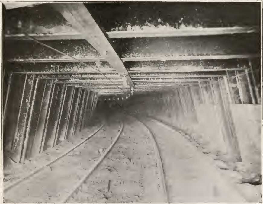
PLATE II. STEEL GAUGEWAY SUPPORTS IN EUREKA MINE. THE VERY LATEST, ALL STEEL.
