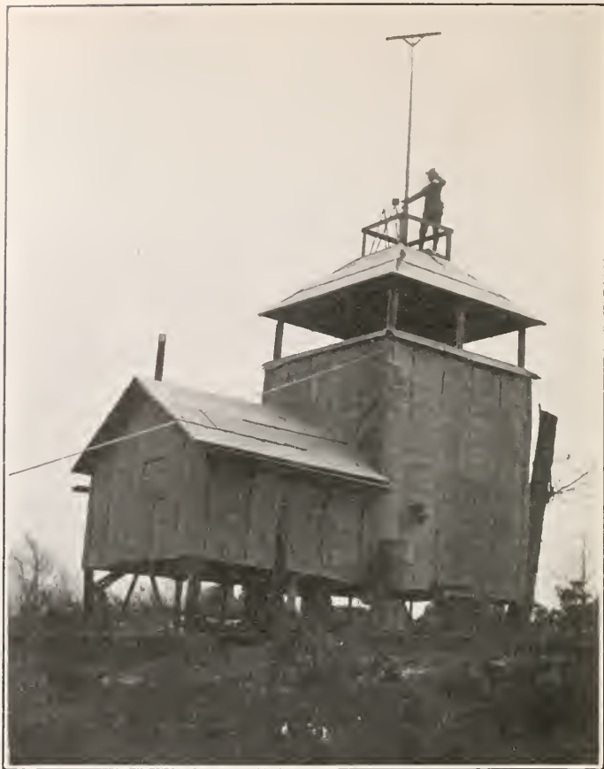
FOREST OFFICER SIGNAL- LING TWENTY MILES BY HELIOGRAPH FROM RANGE FINDER STATION. NIGHT SIGNALS ARE MADE BY POWERFUL ACETYLENE LIGHTS WITH REFLECTOR
