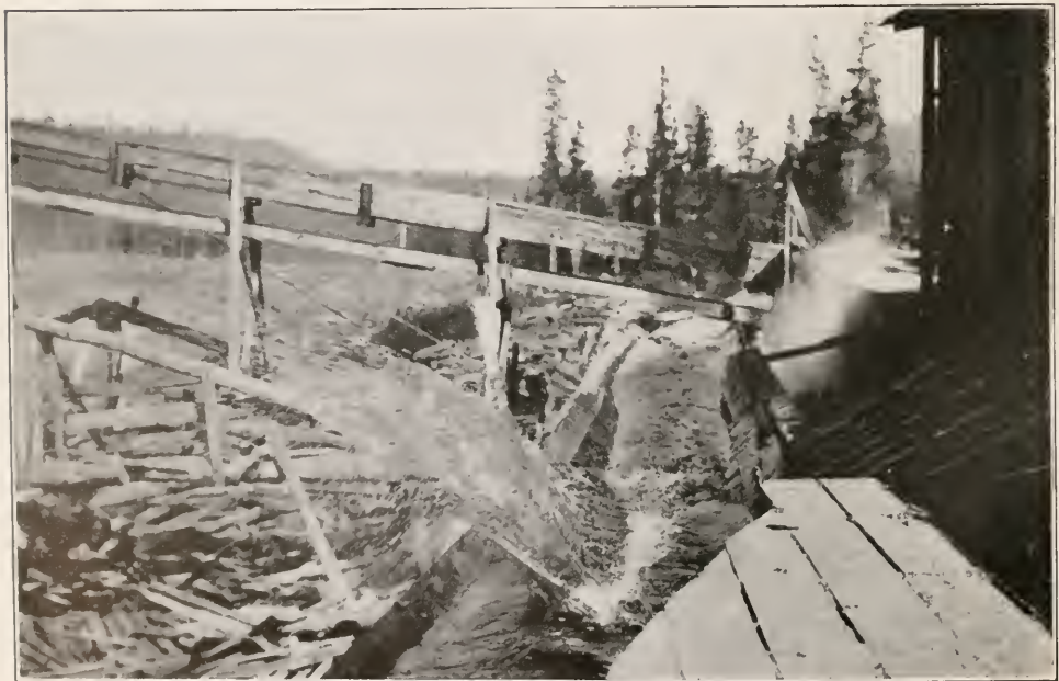
No. 6. THE SPLASH FROM A RAILROAD TIE THAT HAS JUST BEEN THROWN OFF THE CARRIAGE OF THE SMALL SAWMILL, INTO THE FLUME.
