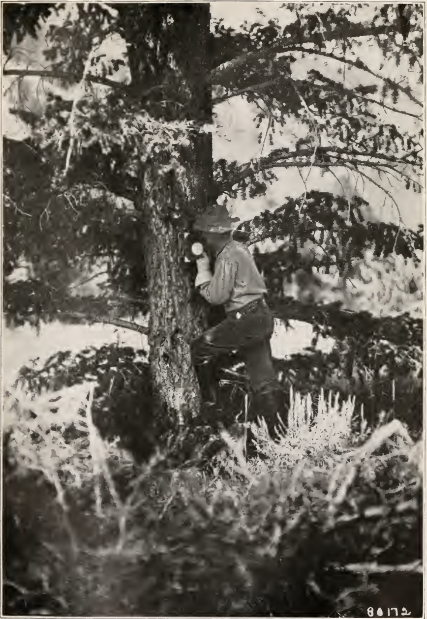
TESTING TELEPHONE LINE AFTER CONSTRUCTING IT
