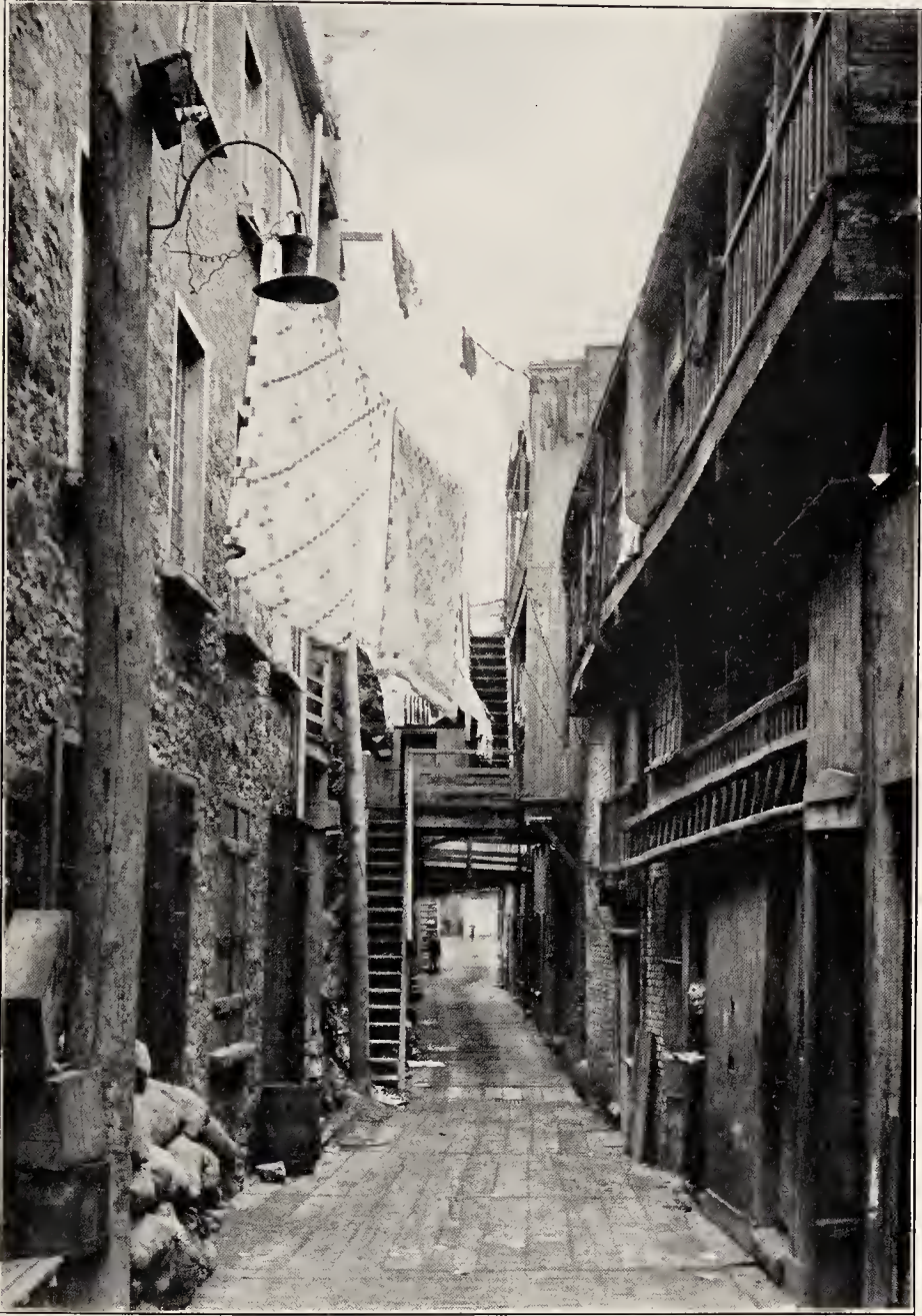
In the old Lower Town are all sorts of narrow streets that may end in the rock cliff, a flight of stairs, or an elevator. Many of them are paved with planks.
