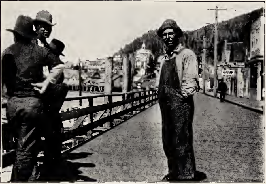
Prince Rupert has miles of streets made of planks, upheld by trestle work, or resting on the rock underlying the city. Most of the streets and building sites were blasted by dynamite from the sides of the mountains.
