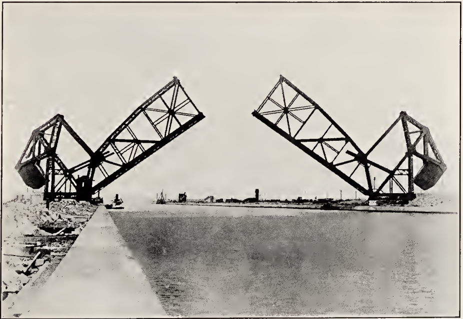
The longest bascule bridge in the world is operated by the Canadian Pacific Railway at Sault Ste. Marie. Each section is 169 feet long, and is raised by electric power to permit vessels to pass through the canal.
