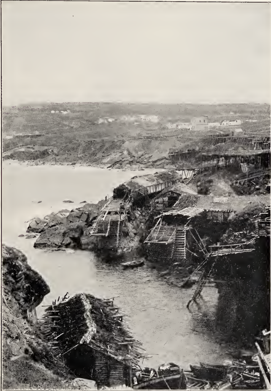
Wherever there is a slight indentation on the high rock-faced coast you will find a fishing village with its landing stages and drying "flakes," built of spruce poles and boughs, clinging to the steep shore.
