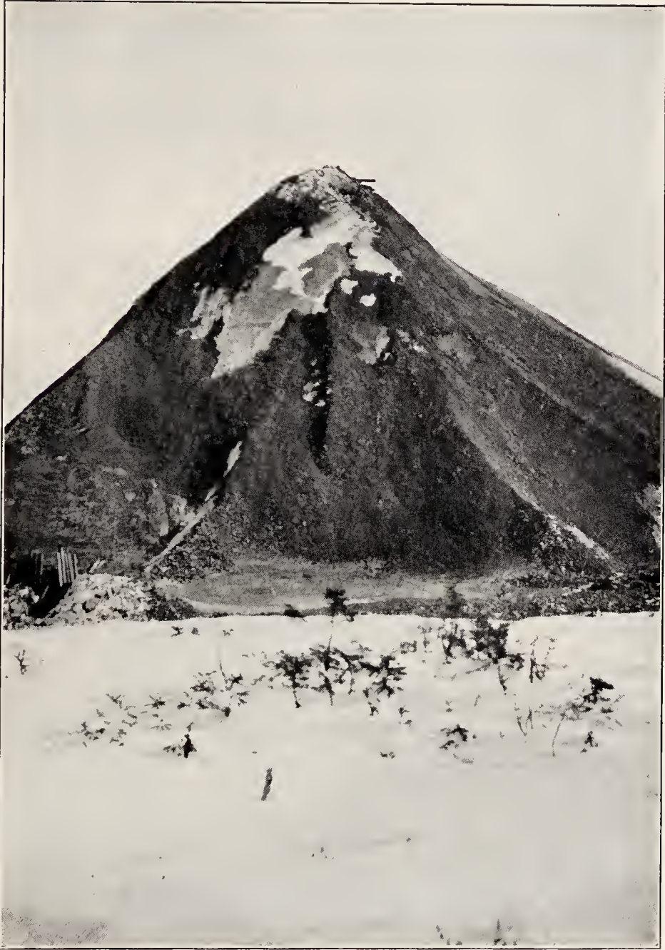
During the winter season the red iron ore from the Wabana mines is stored in huge piles. In the summer it is shipped by steamer to the company's steel mills in Nova Scotia.
