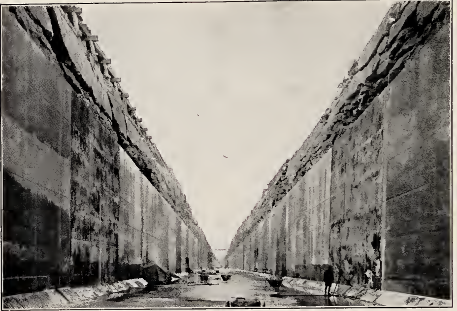
The big ditch that feeds the giant power station was cut through solid rock for miles and carries a stream of water thirty-nine feet deep and fifty feet wide, or more than the flow of a river.
