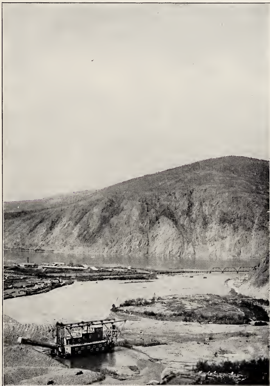
Although the earth contains only a few cents' worth of gold to the ton, the use of giant dredges to scoop up the gravel from the beds of the Klondike and Yukon rivers enables the mining companies to operate at a profit.
