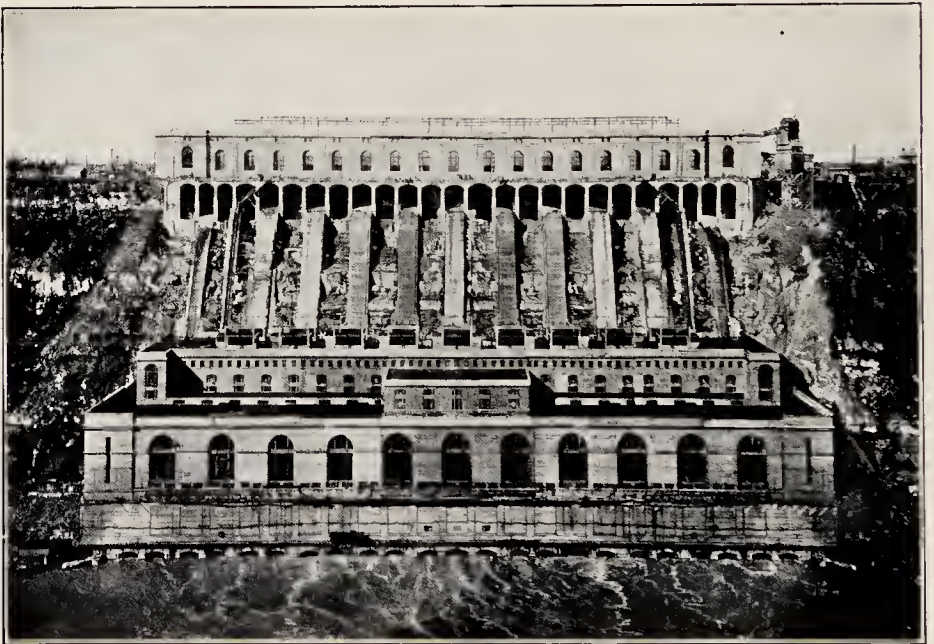
A bucket of water dropped down this cliff to the Niagara River would strike with the force of thirty horse-power. Imagine 20,000 buckets dropped every second and you have the capacity of this 600,000 horse-power station.
