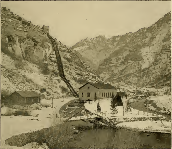
THE LOGAN POWER HOUSE
