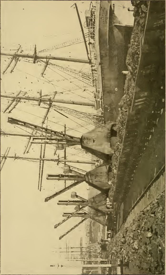
TRAVELLING HYDRAULIC CRANES FOR HANDLING COAL CARGOES ON THE DYKE. BUILT BY SIR W. G. ARMSTRONG, WHITWORTH & CO., LTD., NEWCASTLE-ON-TYNE, ENG.
