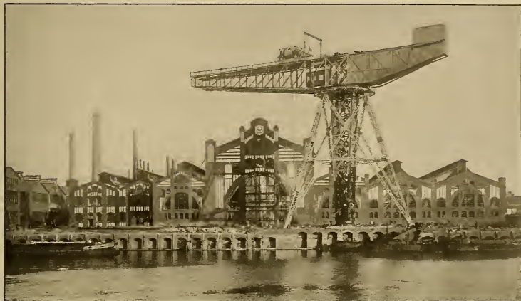
THE 150-TON CRANE AT THE GERMANIA WORKS ¶ ¶
