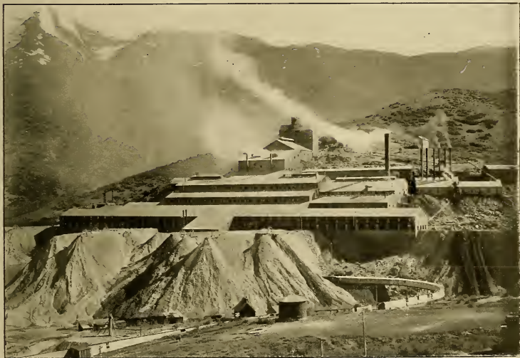
THE MERCUR MILL, SUPPLIED WITH POWER FROM THE PROVO, UTAH, STATION, SHOWN ON PAGES 192 AND 193. THE FIRST INDUSTRY OPERATED BY 40,000-VOLT POWER
