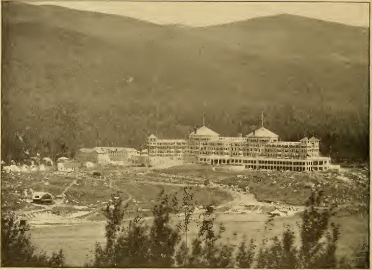
FIG. 9.—HOTEL MT. WASHINGTON, IN THE WHITE MOUNTAINS, AFFORDS A GOOD EXAMPLE OF COMPLETE WATER SUPPLY AND FIRE PROTECTION. SEE PAGE 497
