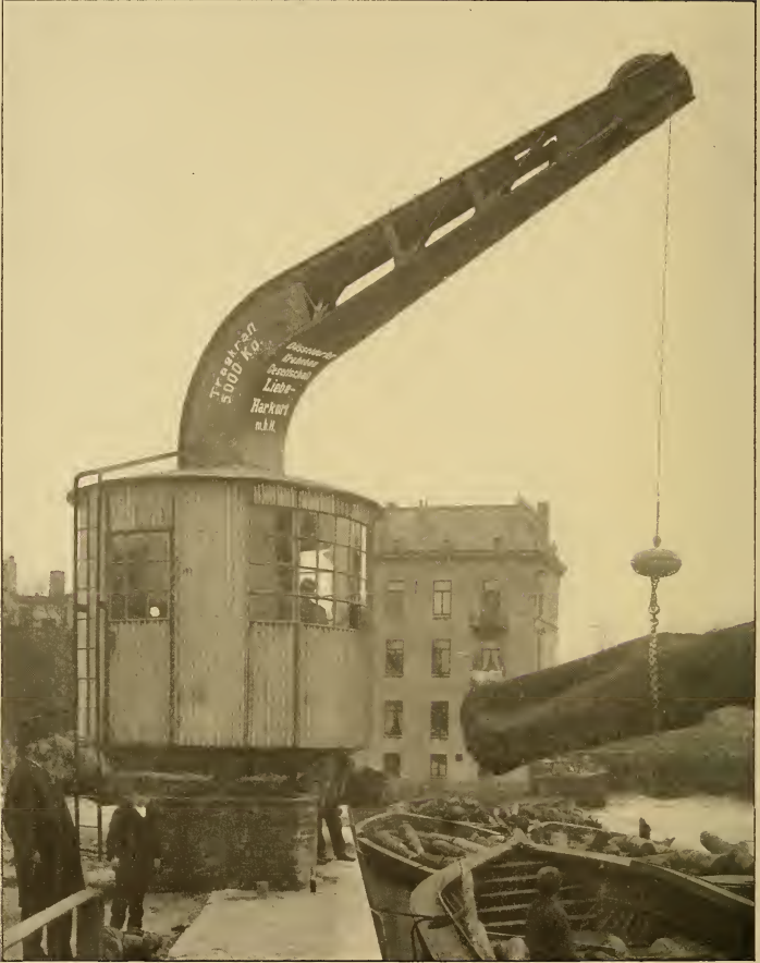
FIG. 14.—A 5-TON ELECTRIC REVOLVING CRANE BUILT BY THE DUESSELDORFER KRAHNBAU-GESELLSCHAFT LIEBE-HARKORT, M. B. H., DUESSELDORF-OBERKASSEL, GERMANY
