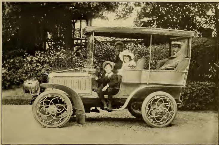
FIG. 2.—AUTOMOBILE EQUIPPED WITH ROUSSEL ELASTIC SPOKE WHEELS MADE BY MM. CADIGNAN & CIE., PARIS
