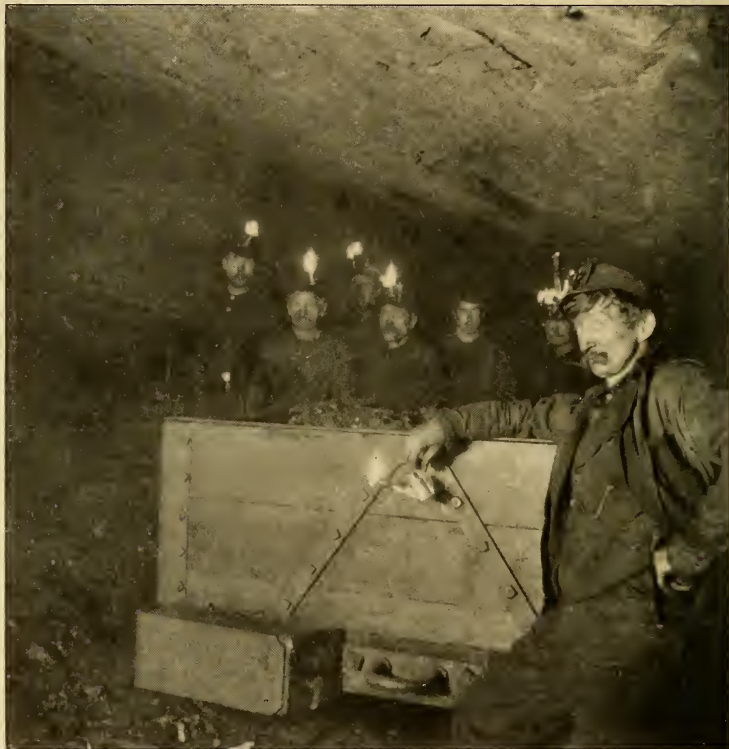
ENTRY IN MERRIMAC MINE
