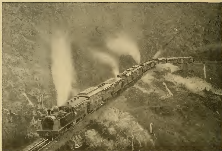
FIG. 1.—AN EXCURSION TRAIN DRAWN BY FOUR FELL ENGINES ON THE RIMUTAKA INCLINE. GRADE, 1 IN 15; WEIGHT OF TRAIN, 174 TONS; LENGTH OF TRAIN, 648 FEET
