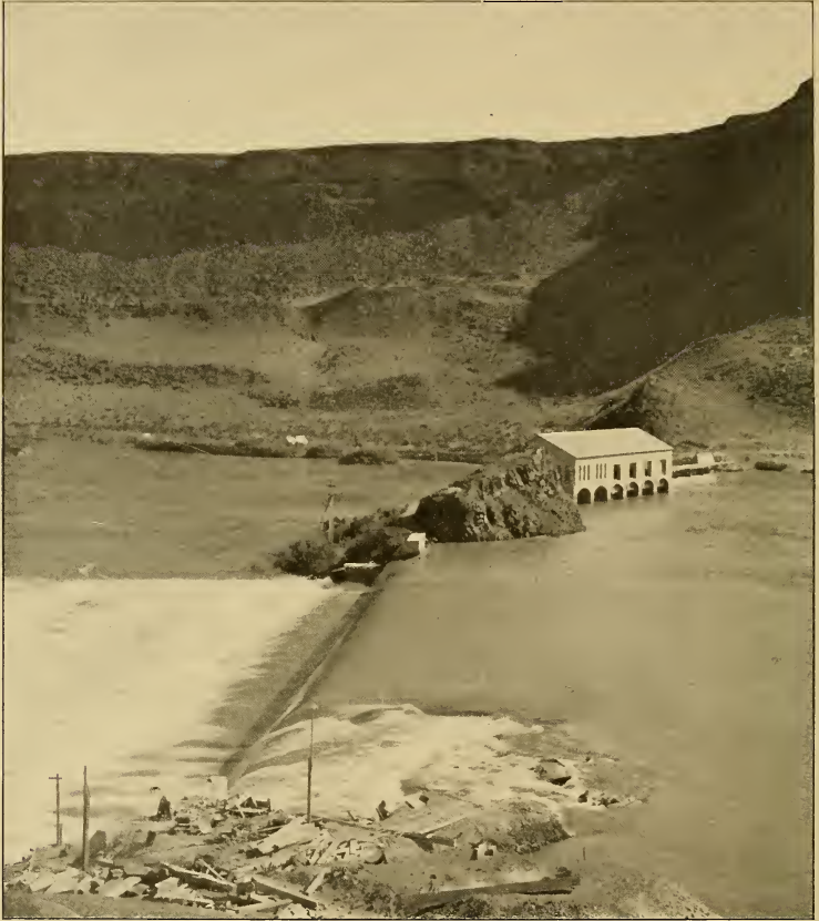
ANOTHER VIEW OF THE POWER HOUSE
