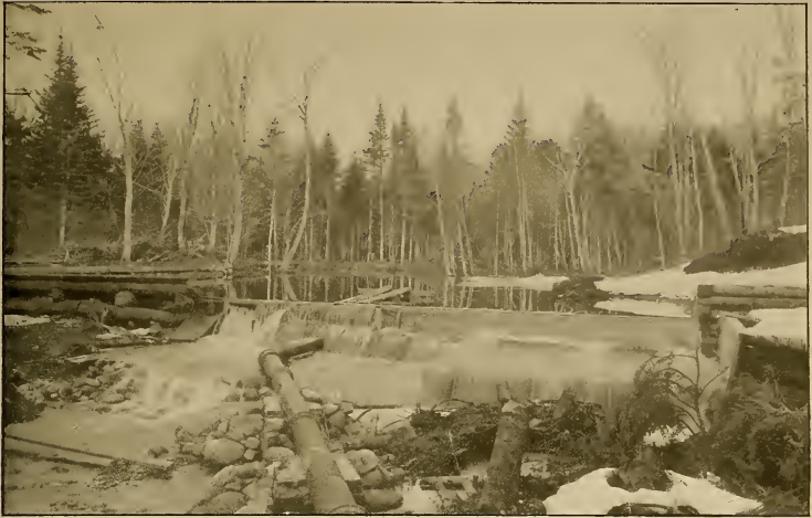
FIG. 13.—THE DAM FOR THE GRAVITY SUPPLY SYSTEM OF HOTEL MT. WASHINGTON
