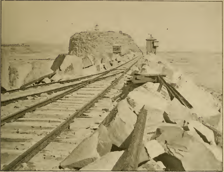
NOBBY'S, ORIGINALLY AN ISLAND AT THE ENTRANCE TO THE PORT OF NEWCASTLE, BUT NOW CONNECTED WITH THE MAINLAND BY A BREAKWATER, AS SHOWN
