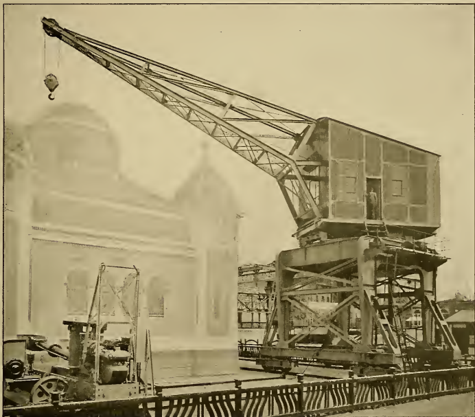
FIG. 6.—A 10-TON PORTAL WHARF CRANE, 49-FT. RADIUS, ELECTRICALLY DRIVEN. BUILT BY THE BEURATHER MASCHINENFABRIK, BEURATH, GERMANY
