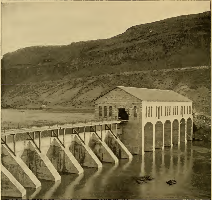
A VIEW OF THE POWER HOUSE AND SECTION OF THE DAM, LOOKING UP-STREAM
