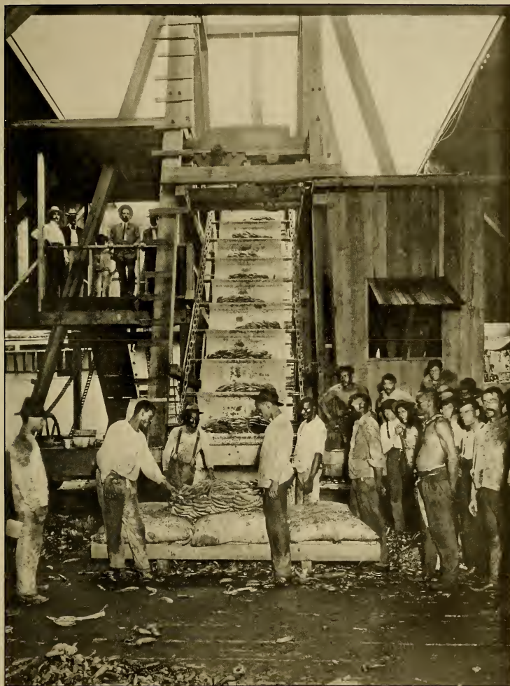
FIG. 3.—THE BANANA CONVEYOR SEEN FROM THE WHARF SIDE, SHOWING WHERE THE BANANAS ARE LANDED, TO BE PASSED INTO CARS FOR FURTHER TRANSPORT
