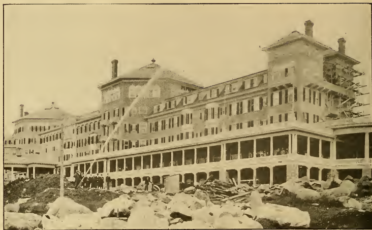
FIG. 14.—A FIRE STREAM IN OPERATION AT MT. WASHINGTON HOTEL
