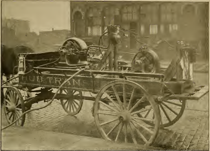
FIG. 4.—IN SOME TOWNS A PORTABLE MOTOR-DRIVEN GENERATOR OUTFIT IS USED IN PLACE OF WATER OR OTHER RHEOSTATS
