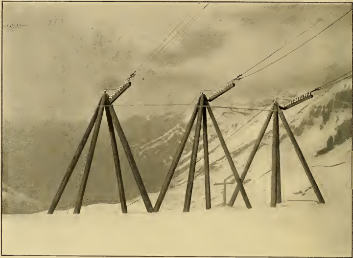
SPECIAL CONSTRUCTION FOR SEPARATION OF CONDUCTORS
