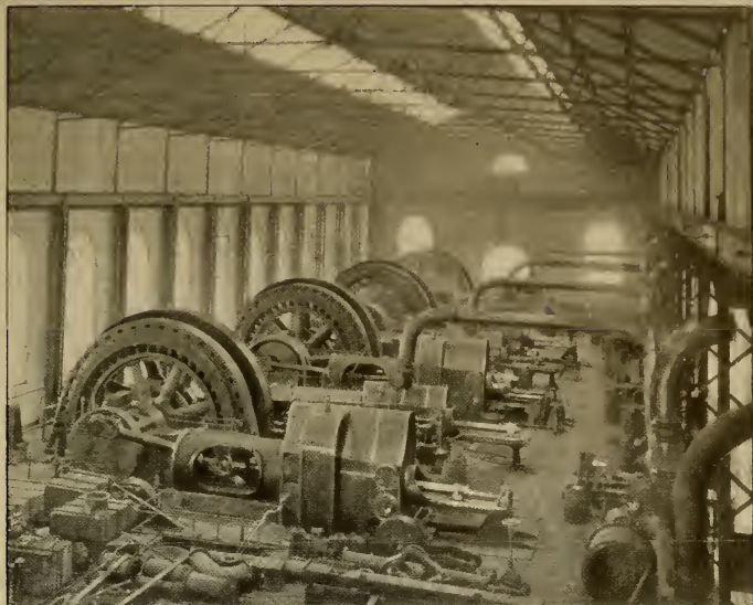
FIG. 3.—INTERIOR OF THE FORMBY POWER HOUSE OF THE LIVERPOOL & SOUTHPORT ELECTRIC RAILWAY, SHOWING CROSS-COMPOUND ENGINES BUILT BY MESSRS. YATES & THOM, BLACKBURN, LANCASHIRE
