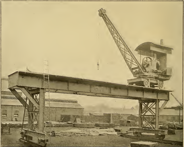
FIG. 1.—A 4-TON STEAM GANTRY CRANE, BUILT BY MESSRS. RANSOMES & RAPIER, LTD., IPSWICH
