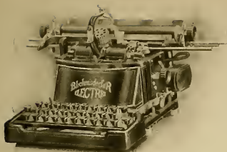
AN ELECTRIC TYPEWRITER MADE BY THE BLICKENSDERFER MANUFACTURING CO., STAMFORD, CONN.
