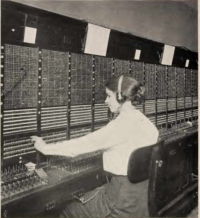
FIG. 52.—Switchboard for A operators
