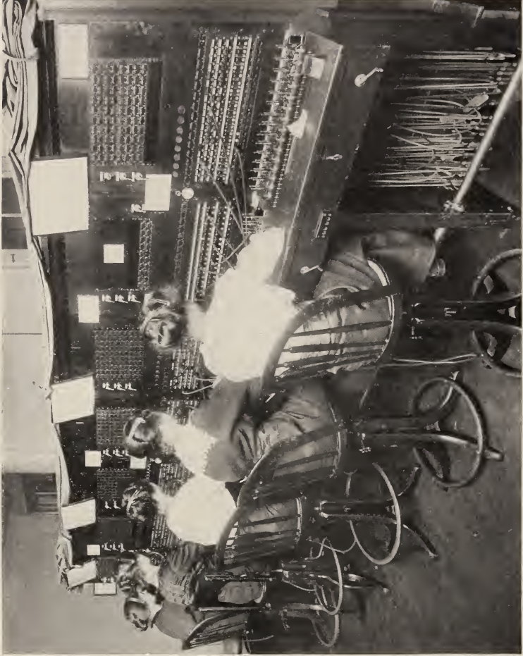
FIG. 18.—A magneto switchboard
