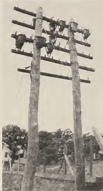
FIG. 10.—Loading coils on an aerial line
