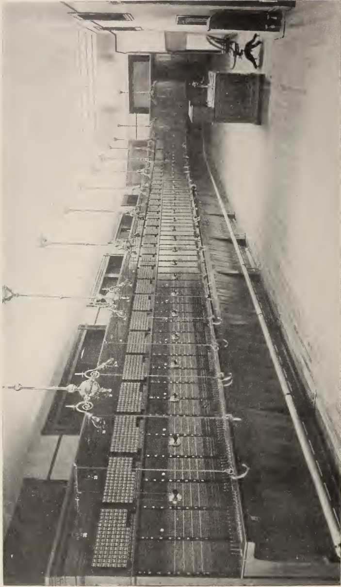
FIG. 4.—1 multiple switchboard—magneto type
