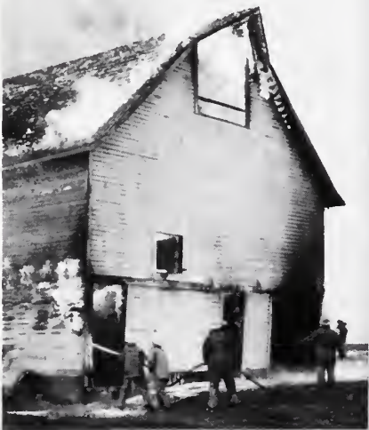
Figure 1—Initial attack on barn engulfed with fire.
