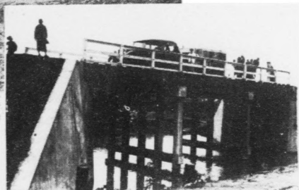
Above—Ta-Chiao Bridge with Concrete Abutments, Reinforced Concrete Bents and Timber Floor —Anhwei Section
