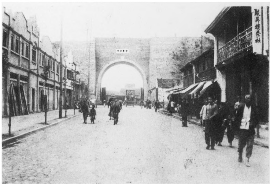
Above—East Gate of Chun-Hwa-Men, the Starting Point of the Nanking-Wuhu Highway-Nanking
