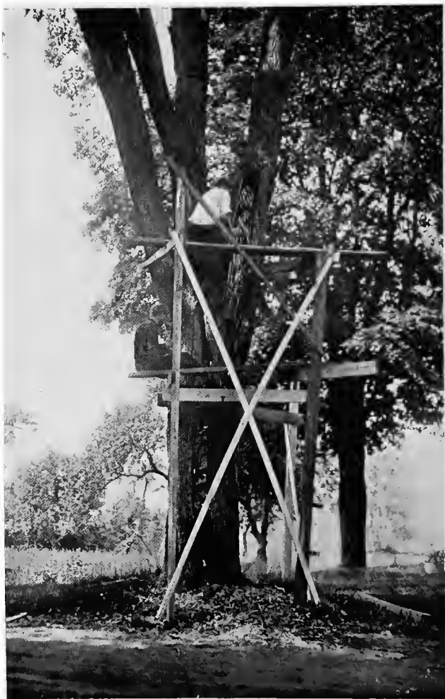
Excavating a large cavity
