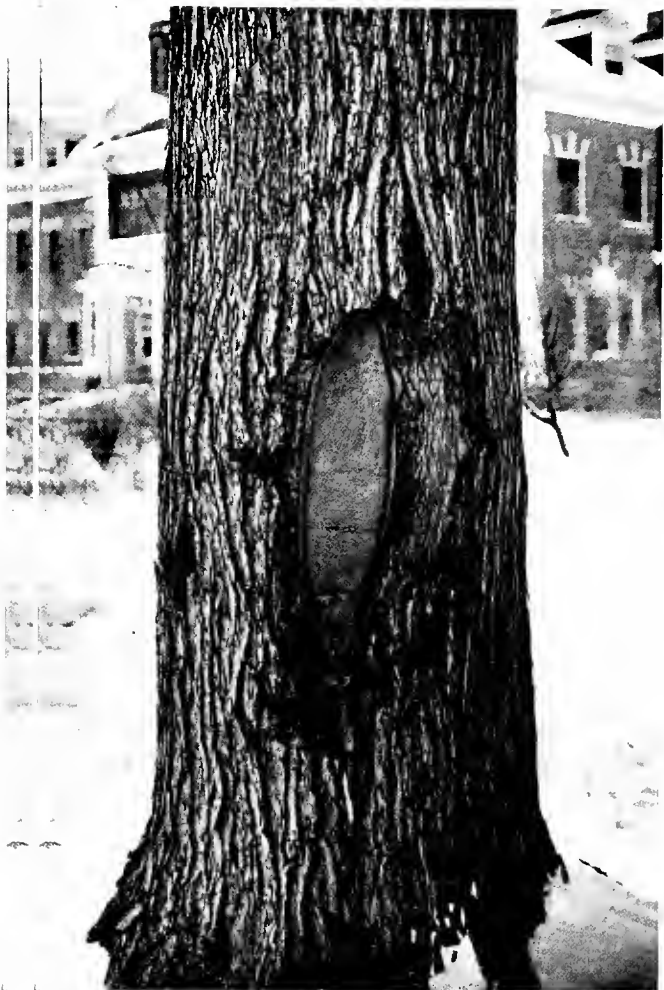
Small cavity in white oak correctly filled with concrete
