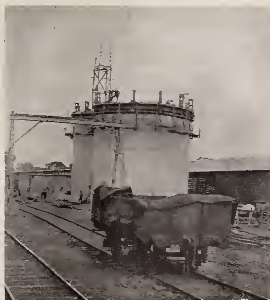
100,000 BUSHEL ELEVATOR UNDER CONSTRUCTION AT URANQUINTY
