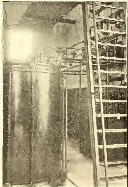
WATER-COOLED, OIL-INSULATED TRANSFORMERS AND OIL SWITCHES IN POWER STATION
