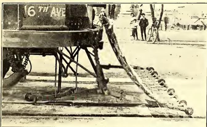
SWITCH BEING THROWN BY MOTORMAN ON CAR
