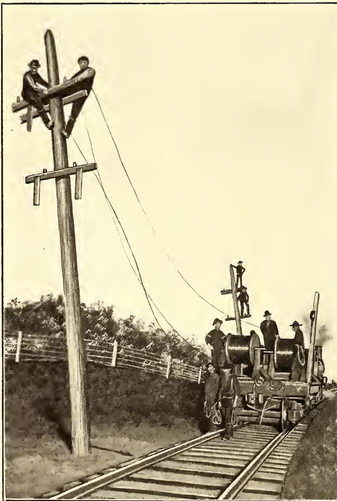
STRINGING HIGH-TENSION TRANSMISSION WIRES BY LOCOMOTIVE
