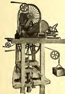
Allis Telescopic Double-Cutting Band Mill
