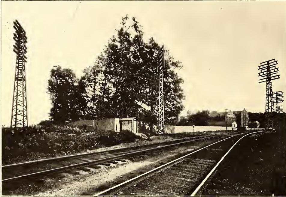
THE TYPE OF STRAIN POLES USED AT TRANSMISSION CROSSINGS
