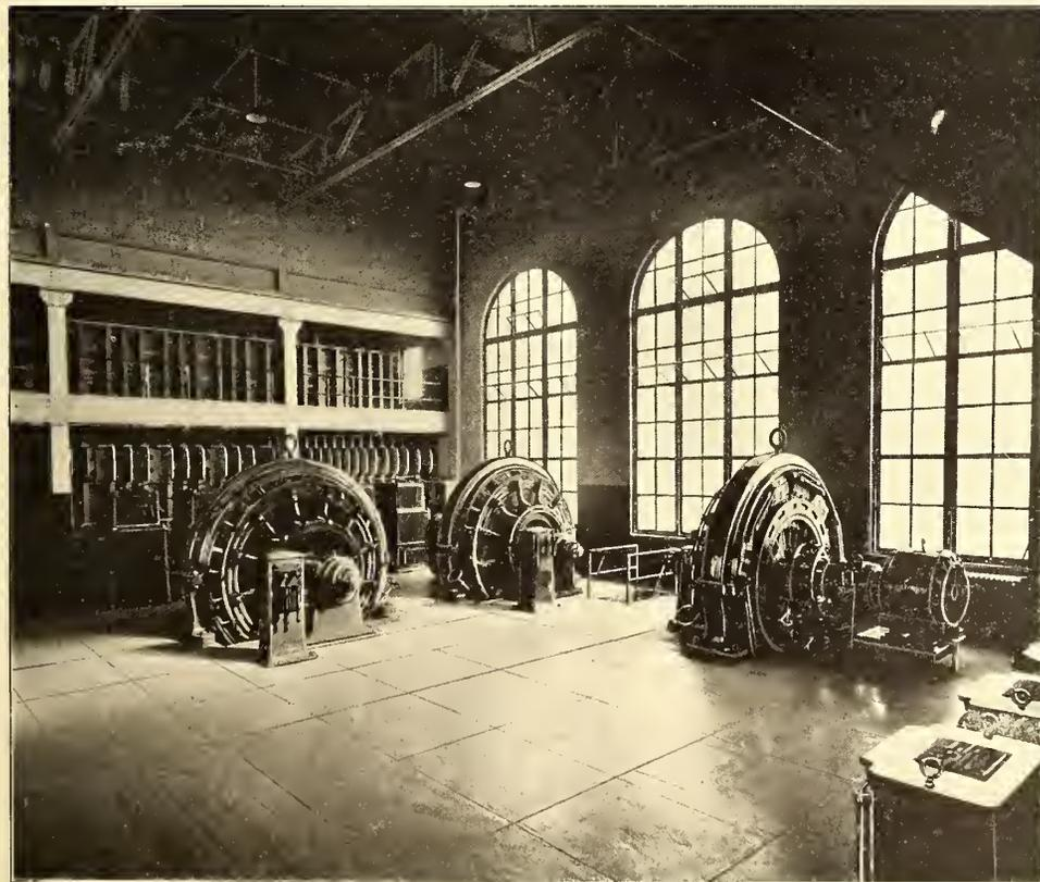
INTERIOR VIEW OF EAST NEW YORK SUB-STATION, SHOWING ARRANGEMENT OF ROTARIES, TRANSFORMERS AND SWITCHING GALLERIES
