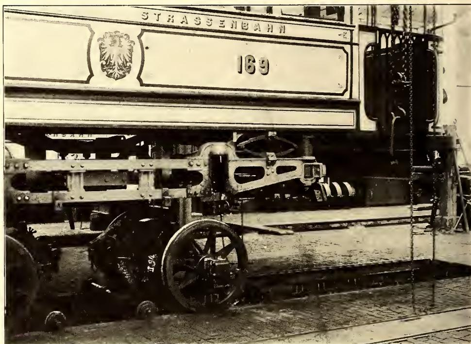
VIEW SHOWING METHOD OF HOISTING CAR-BODY AND TRUCKS, LEAVING THE WHEELS AND MOTORS TO BE REMOVED ELSEWHERE
