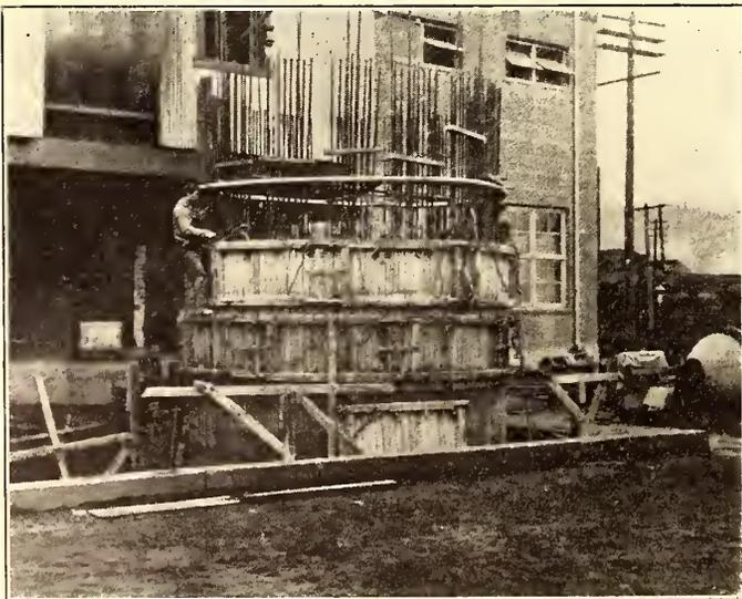
FIG. 1.—VIEW OF CONCRETE CHIMNEY IN COURSE OF CONSTRUCTION
