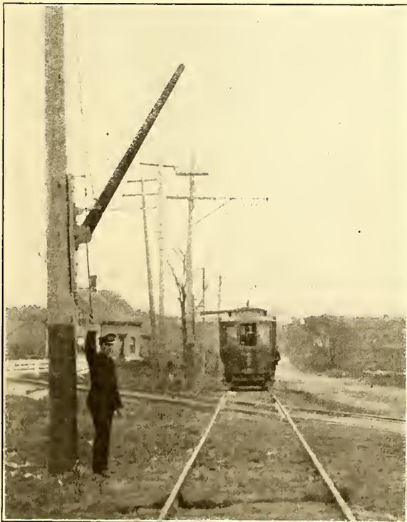
FIG. 1.—CONDUCTOR RAISING THE STOP-GATE
