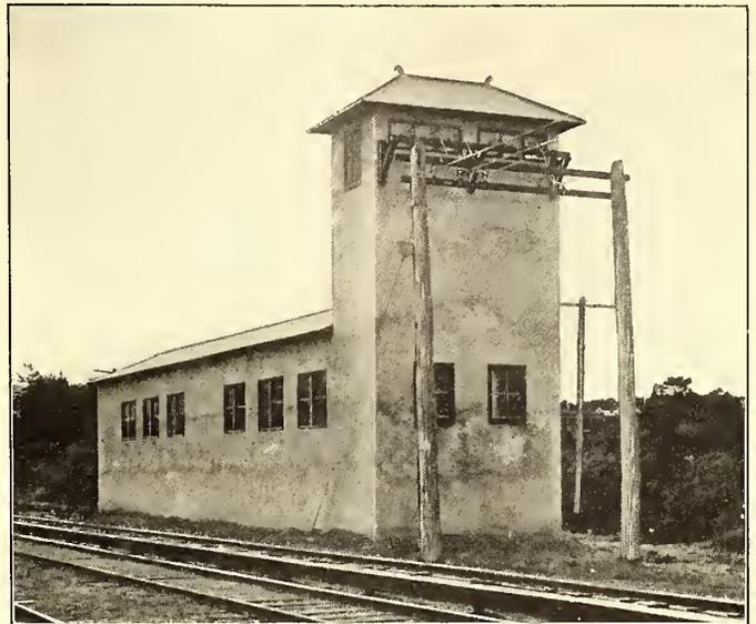
THE STEEL-CONCRETE HOUSE AT BELMONT PARK, USED FOR HOUSING TWO PORTABLE SUB-STATIONS
