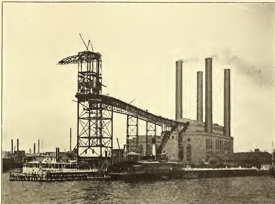
EXTERIOR VIEW OF THE LONG ISLAND CITY POWER STATION ON THE EAST RIVER, SHOWING ALSO THE COAL-HANDLING APPARATUS AND TRESTLE
