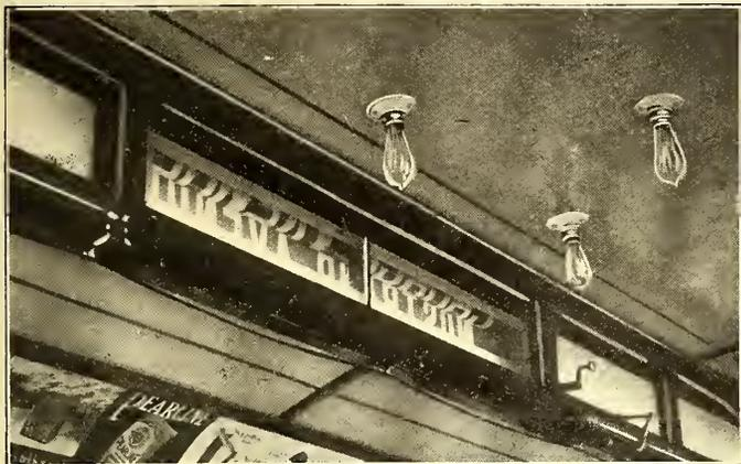
FIG. 20.—SIGN, SHOWING POSITION OF LAMPS BEHIND IT
