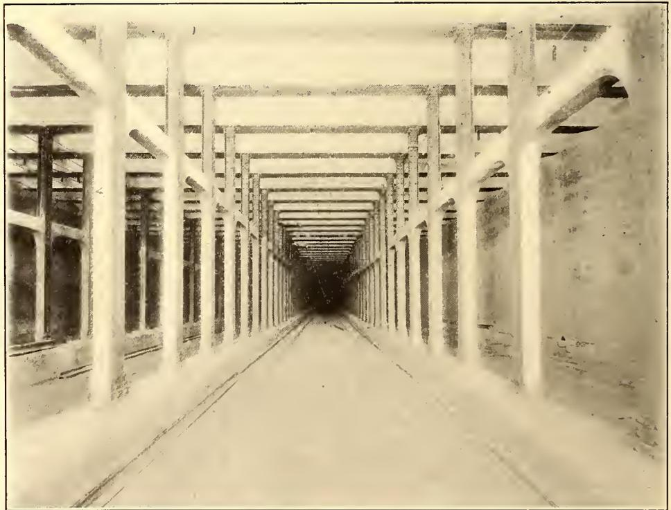
VIEW TAKEN SEPT. 26, 1905, BEFORE TRACKS WERE LAID, SHOWING REINFORCED CONCRETE STRUTS BETWEEN COLUMNS
