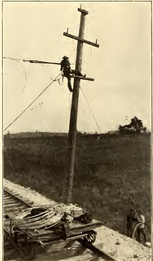
FASTENING GUY ANCHORS AND PULLING UP SPAN WIRE
