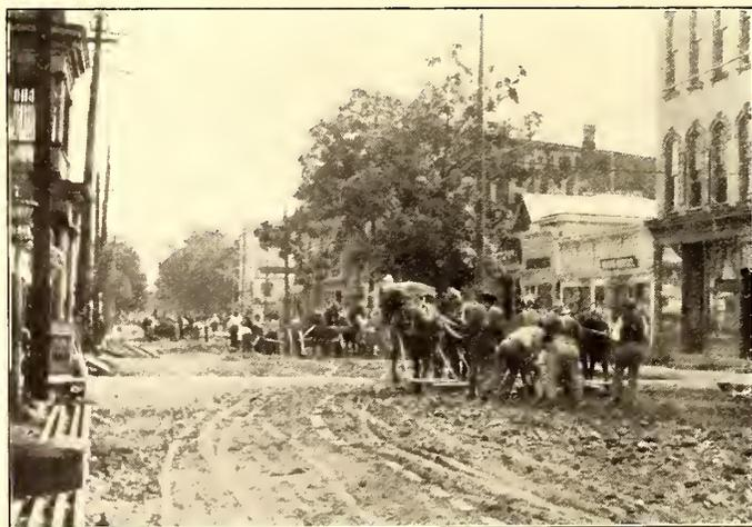
TEARING UP STREET SURFACE WITH ROOTER PLOWS
