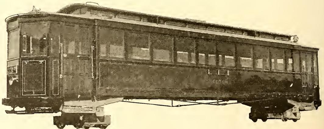
ONE OF THE NEW PITTSBURG CARS BEFORE BEING MOUNTED ON ITS TRUCKS
