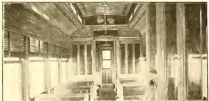
INTERIOR VIEW OF ANTIOQUIA CAR, SHOWING SLAT SEATS IN SECOND-CLASS COMPARTMENT AND CANE SEATS IN THE FIRST-CLASS COMPARTMENT
