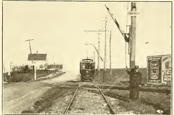
FIG. 2.—CONDUCTOR HOLDING THE STOP-GATE UP
