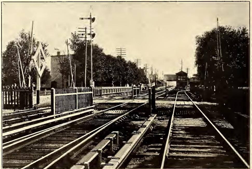
THIRD-RAIL LAYOUT AT HIGHWAY CROSSING NEAR WOODHAVEN JUNCTION, SHOWING ALSO SIGNALS, CATTLE GUARDS, GATES, ETC.
