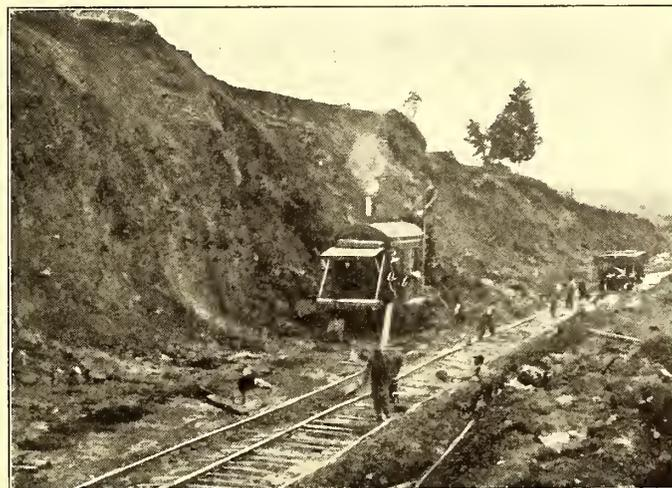
EXCAVATING IN 54,000-CU. YD. CUT NEAR PALMYRA
