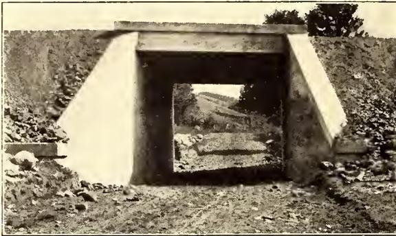
20-FT. SPAN CONCRETE STRUCTURE. DECK OF I-BEAMS IN CONCRETE. SIDE WINGS ARE ARRANGED TO AVOID FORMING A BLIND CURVE
