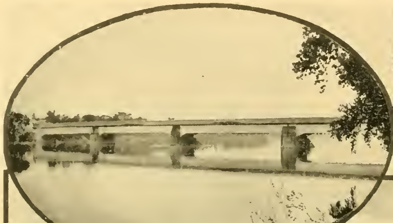
OLD WATERFORD BRIDGE
