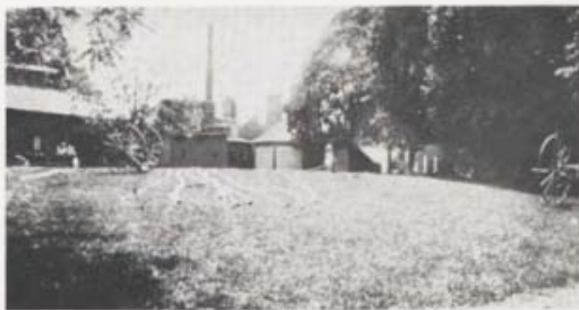
AFTER THE FIRE
