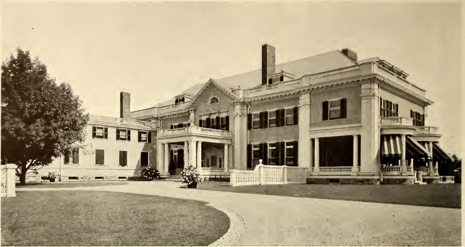
The Principal Characteristic of the Exterior are the Pilasters, which are Finished with Ionic Capitals
