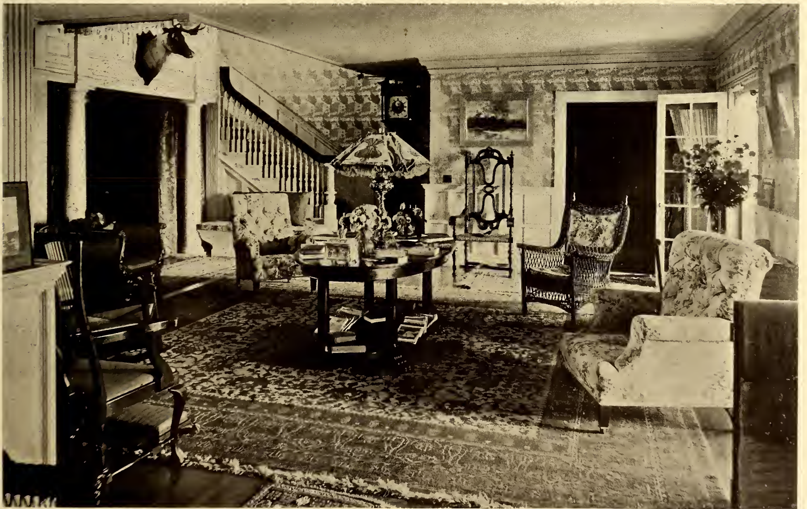
"Heim Mere"—The Hall and Staircase
