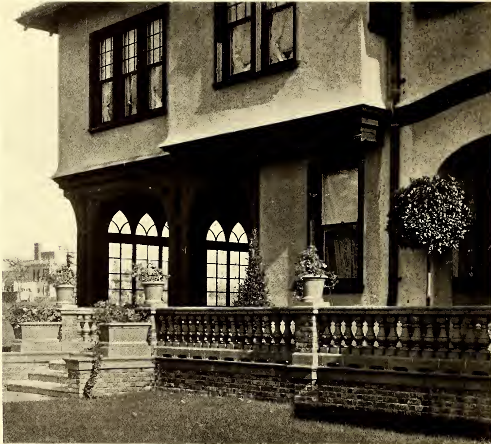
The Entrance Porch and Porte-Cochère
