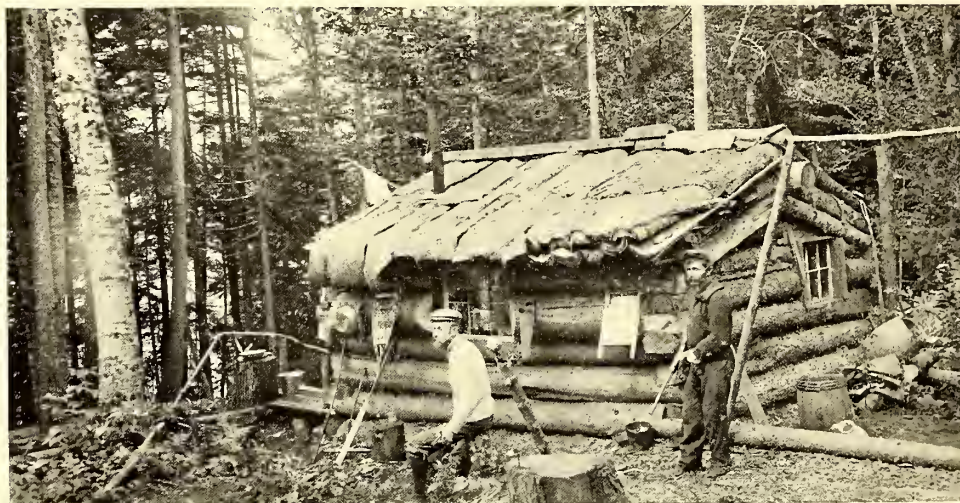
A Useful Device in Roof Construction, Showing How the Logs have been Hollowed Out and Laid in the Manner of a Tile Roof
