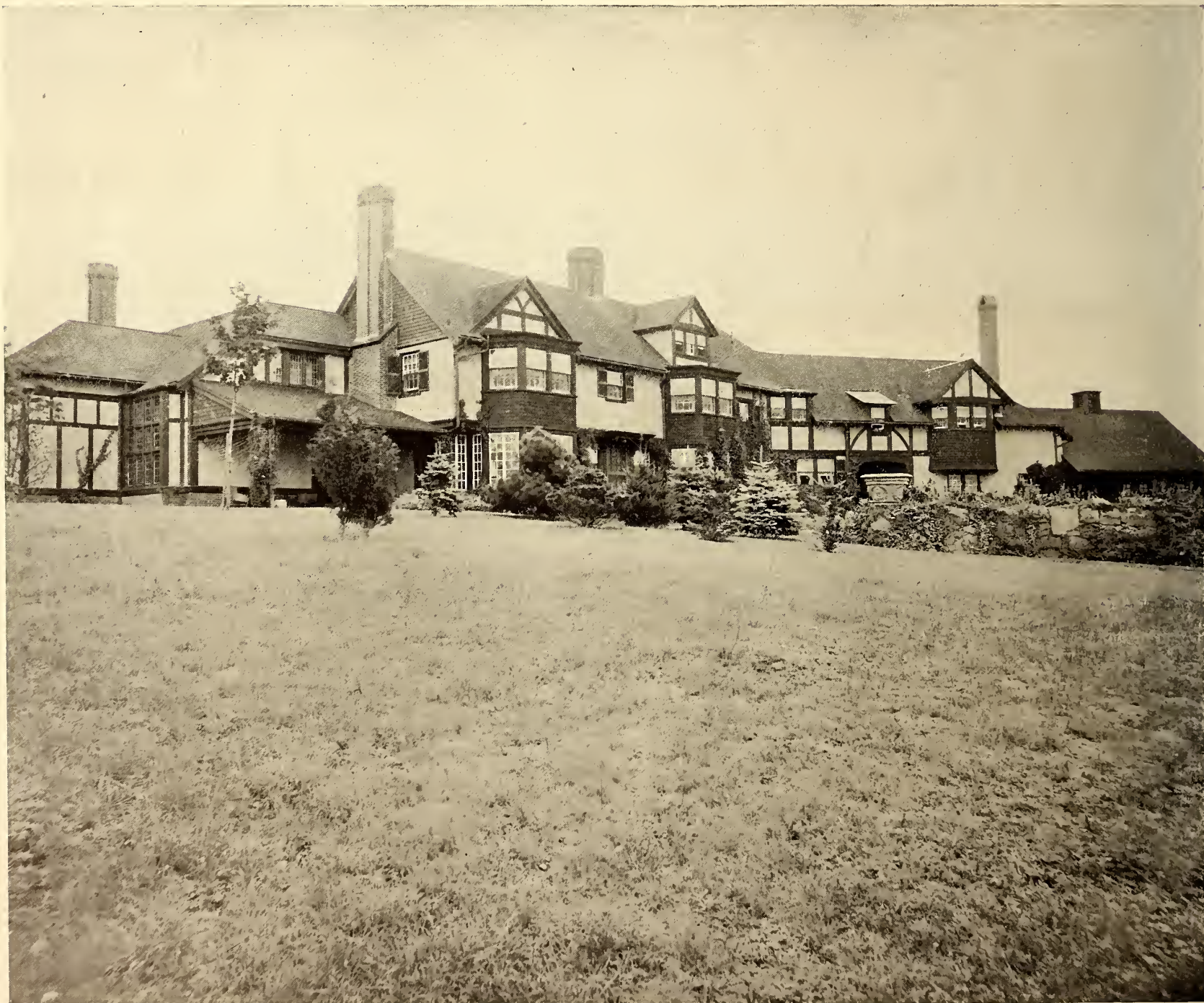
“Craigston”—The Entrance Front
