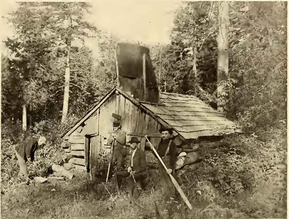
The Use of Boards and Shingles Greatly Simplifies the Work of Construction, But They Are Not Always to Be Obtained
