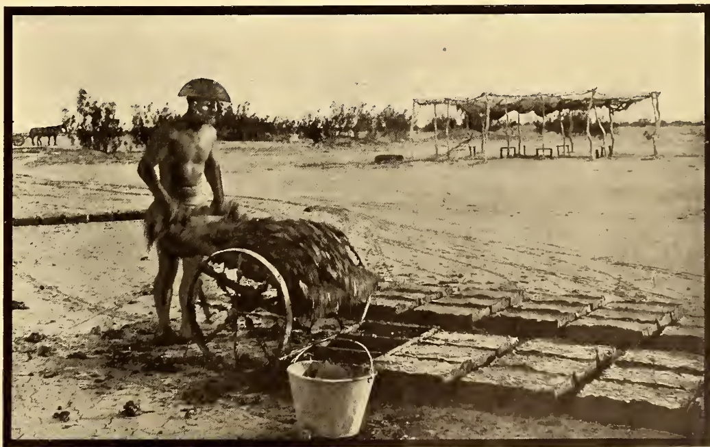
A Minister Making Adobe Brick Sun-Dried at a Temperature of 130 Degrees, with which to Build a Church. The Present Church is Seen in the Background, and is Called "Grace and Glory Land"
