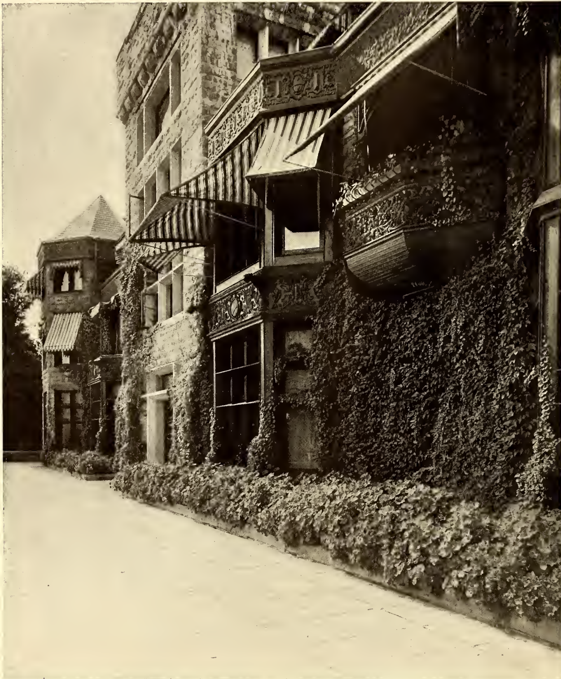
A Glimpse of the Façade and the Terrace. The Outer Wall is Tapestried with Vines; Flower Beds Flank the Walk
