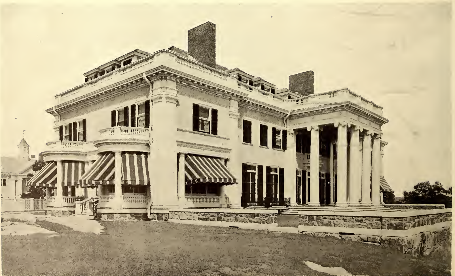
A House Designed in the Colonial Style and Built of Stucco Left in its Natural Silvery Gray Color
