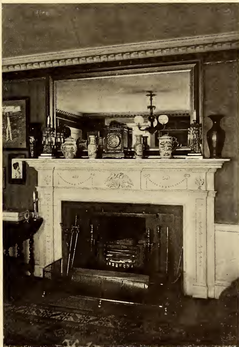
Fig. 6—A Colonial Mantel, Showing the First Hob Grate Introduced into Salem
