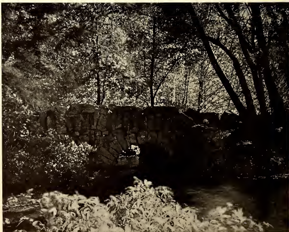
An Arch of Massive Stones Connects Two of the Small Lakes
