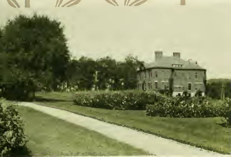
Wilson Hall from rear
