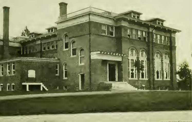
Kitchen and Dining Hall
