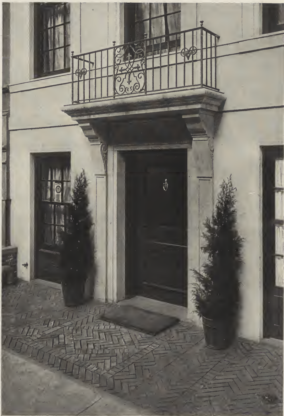
RESIDENCE OF GRENVILLE T. EMMET, ESQ., NEW YORK. MOTT B. SCHMIDT, ARCHITECT.
