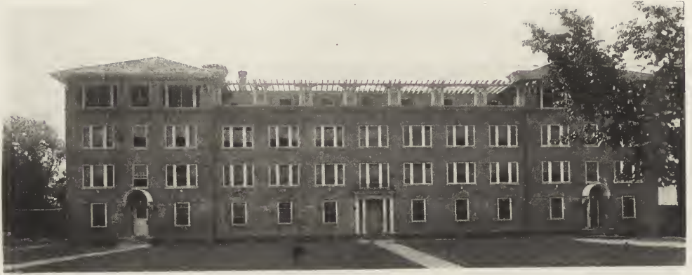
BOYS' DORMITORY (JAMES HALL), HAMPTON NORMAL AND AGRICULTURAL INSTITUTE, HAMPTON, VA. Ludlow & Peabody, Architects.
