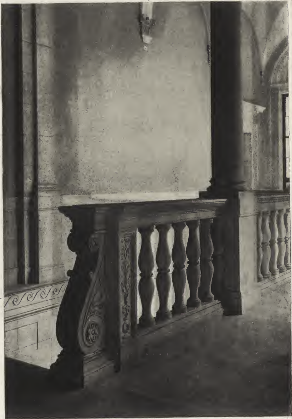
DETAIL OF BALUSTRADE—RESIDENCE OF OTTO H. KAHN, ESQ., NEW YORK. J. ARMSTRONG STENHOUSE, ARCHITECT.
