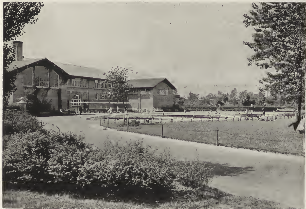
FIELD HOUSE—HAMILTON PARK, CHICAGO. D. H. Burnham & Co. (Graham, Anderson, Probst & White), Architects.
