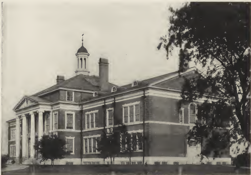
NORTH AND WEST FRONTS—HIGH SCHOOL, SOUTHAMPTON, L. I. William Lawrence Bottomley, Architect.
