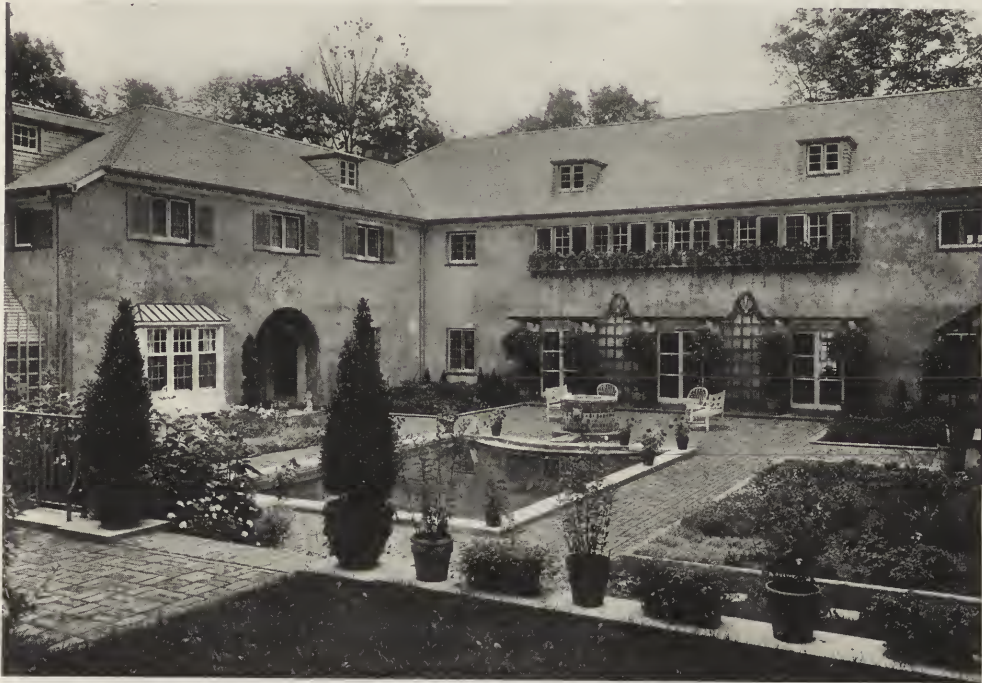
FIG. 13B. COURT—RESIDENCE OF C. A. BARTLETT, ESQ., LAKE GENEVA, WIS. Howard Shaw, Architect.
