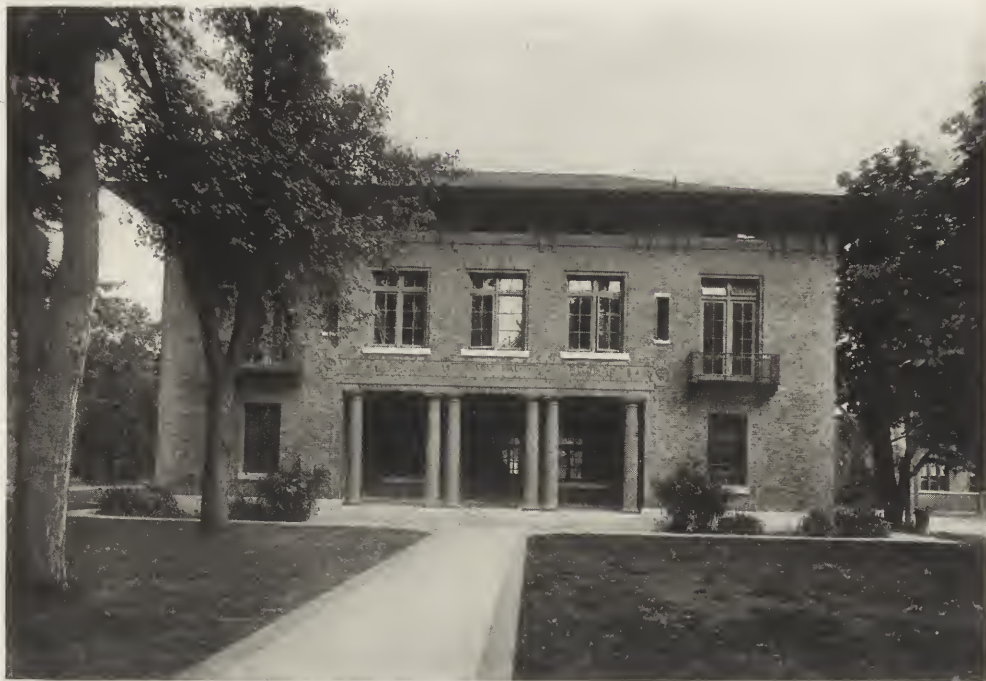
RECREATION BUILDING (CLARKE HALL), HAMPTON NORMAL AND AGRICULTURAL INSTITUTE, HAMPTON, VA. Ludlow & Peabody, Architects.
