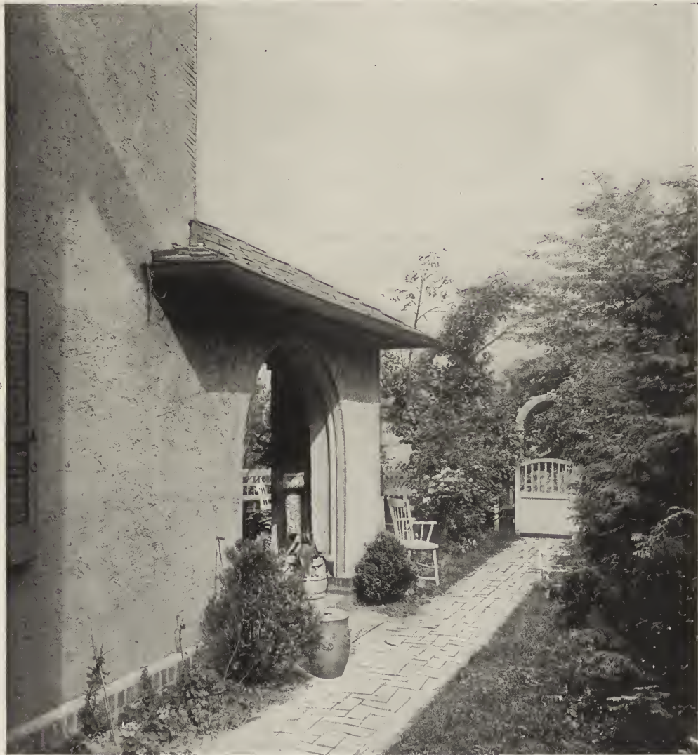
GARDEN GATE—HOUSE OF E. DIGBY BALTZELL, ESQ., ST. MARTIN'S, CHESTNUT HILL, PHILA- DELPHIA. EDMUND B. GILCHRIST, ARCHITECT.
