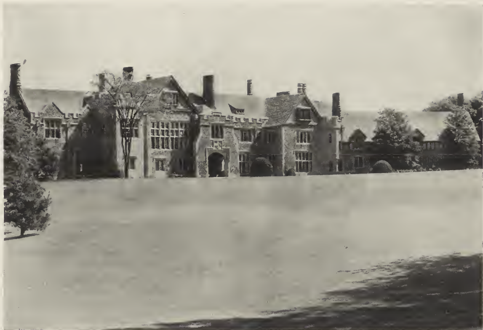
FIG. 5. VIEW FROM THE SOUTH—RESIDENCE OF STEWART DUNCAN, ESQ., NEWPORT, R. I. John Russell Pope, Architect.
