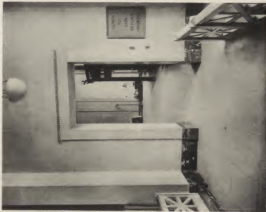
DOORWAY OF ELEVATOR LOBBY—COMMERCIAL NATIONAL BANK BUILDING, WASHINGTON, D. C. WADDY B. WOOD, ARCHITECT.
