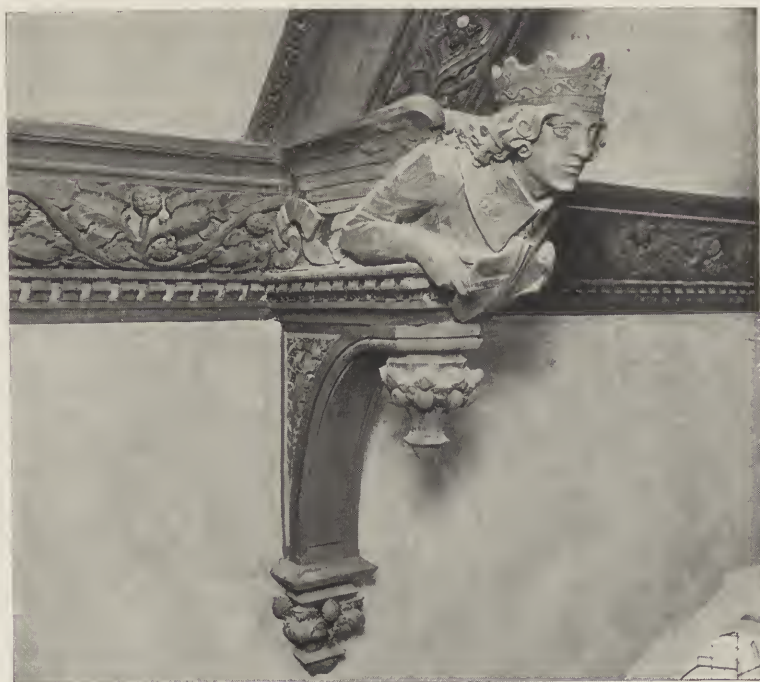
FIGURE CORBEL UNDER CEILING BEAMS — LAKE AVENUE BAPTIST CHURCH, ROCHESTER, N. Y. FOOTE, HEADLEY & CARPENTER, ARCHITECTS.
