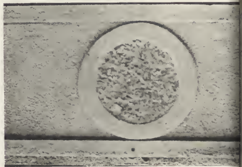
Interior of Circle Is Pebble Dash; Rim of Circle Troweled and Body Surface Sand-Floated.
