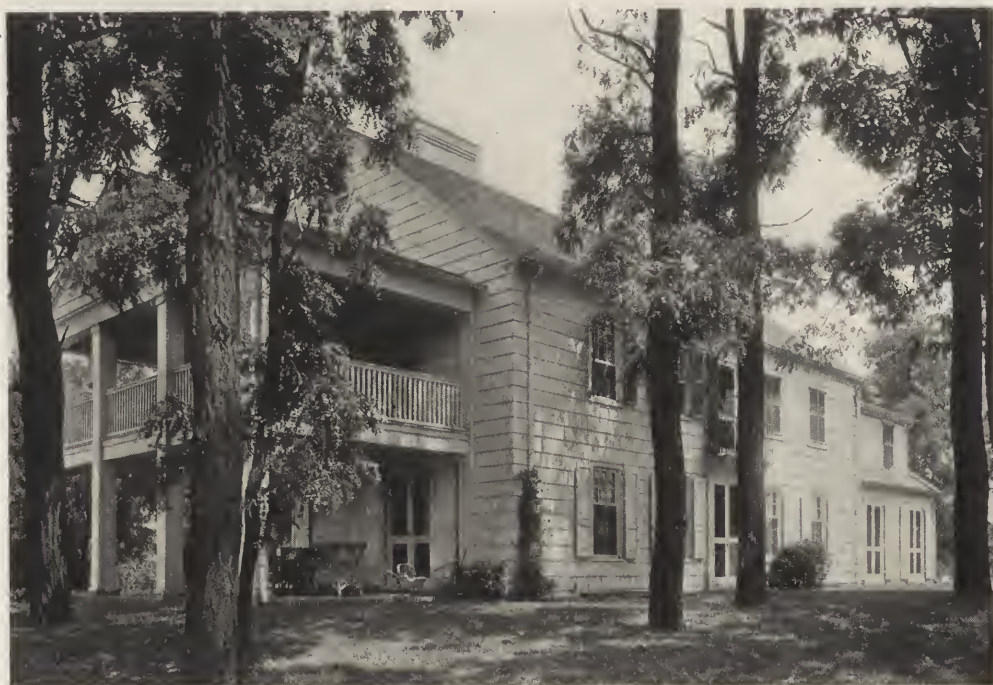
FIG. 39. WEST AND SOUTH FRONTS—RESIDENCE OF H. P. WHITNEY, ESQ., GLEN COVE, L. I. Charles Willing of Furness, Evans & Co., Architect.
