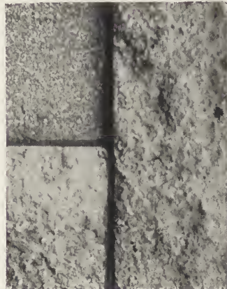
Corner Blocks Are Finished in the Same Way That Stones Are Quarry Faced. The Others Are Finished With the Pointer.
