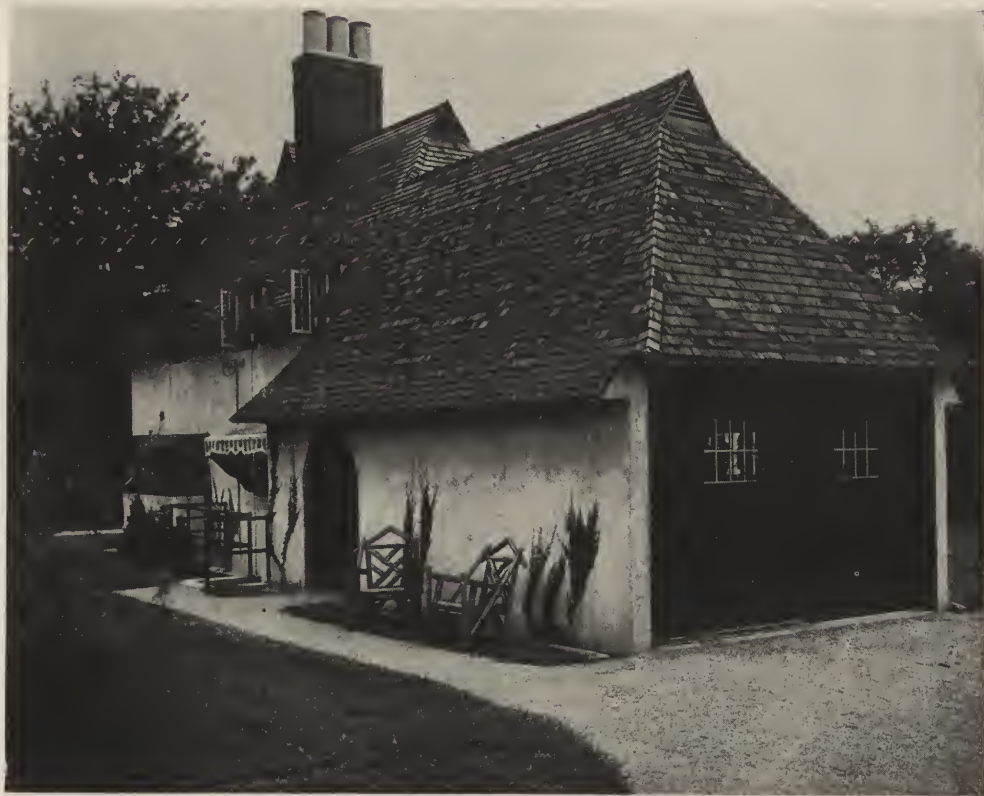
GARAGE — RESIDENCE OF WALTER B. WALKER, ESQ., ARDSLEY, N. Y. Frank J. Forster, Architect.
