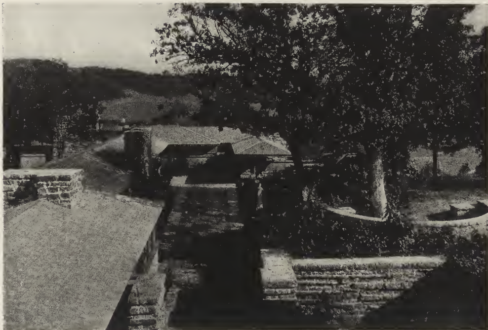
FIG. 15. GENERAL VIEW OF FORECOURT AS SEEN FROM THE GRANARY—ESTATE OF FRANK LLOYD WRIGHT, SPRING GREEN, WIS. Frank Lloyd Wright, Architect.
