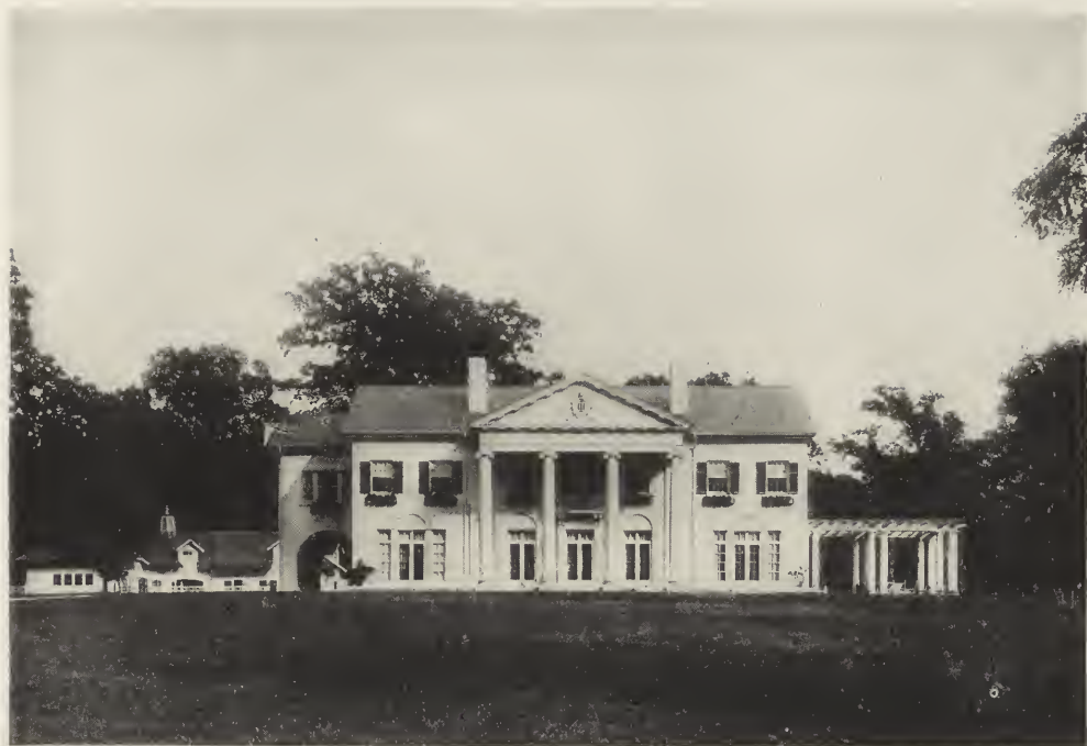
FIG. 103. RESIDENCE OF J. A. HITCHCOCK, ESQ., NASHVILLE, TENN. Dougherty & Gardner, Architects.
