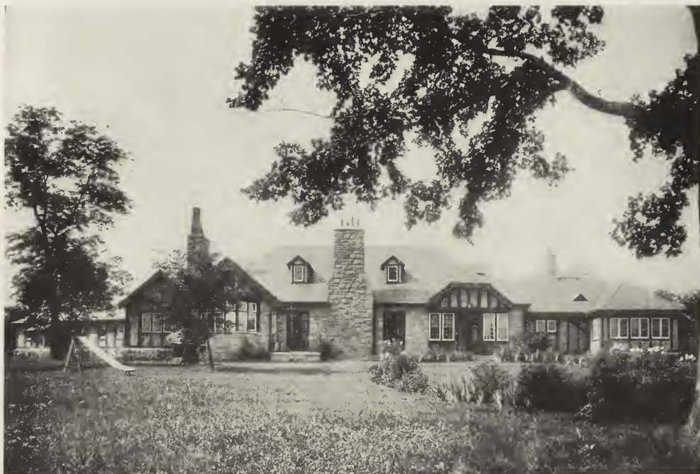
FIG. 86. GARDEN FRONT—RESIDENCE OF DR. W. D. HAGGARD, NASHVILLE, TENN. Dougherty & Gardner, Architects.
