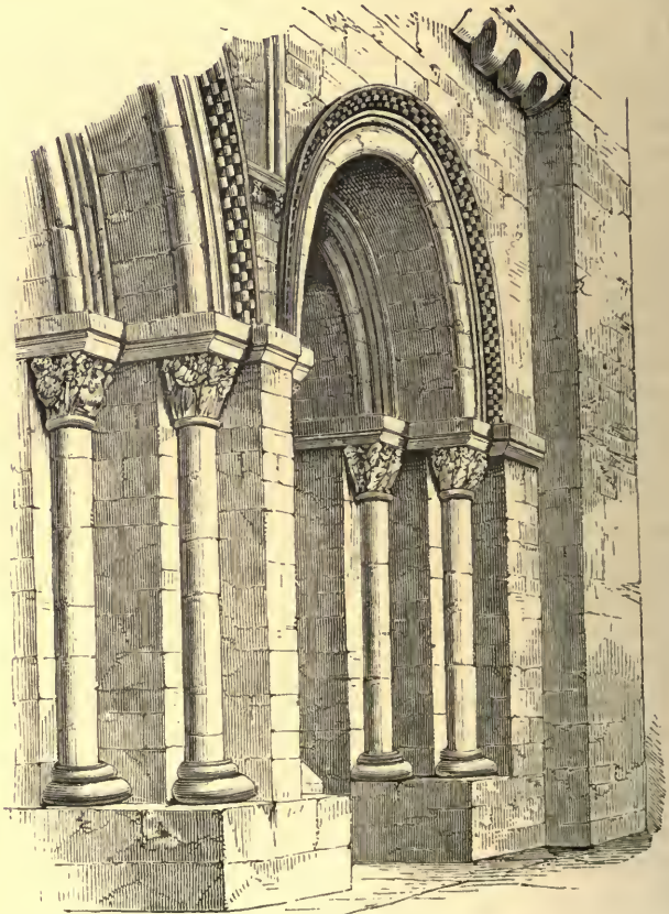
FIG. 171.—ARCHES IN RECEDING PLANES AT ST. SERVIN, TOULOUSE.
