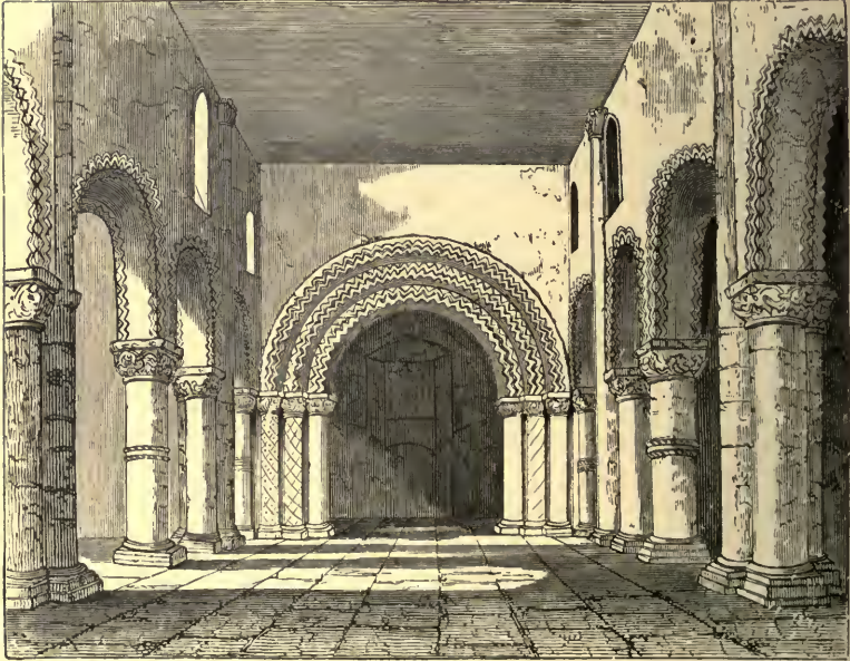
FIG. 172.—NORMAN ARCHES IN ST. PETER'S CHURCH, NORTHAMPTON.
