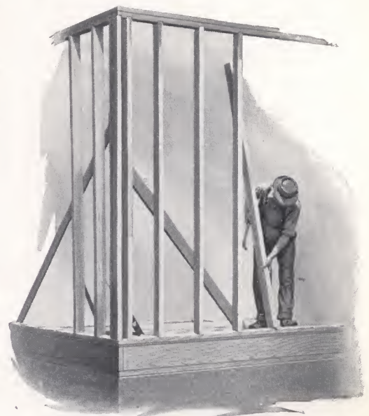
Notches Make Assembling Easy
