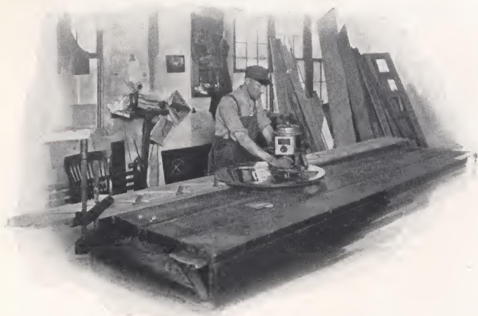
A Better-Built idea—routing (instead of cleating) stair-stringers for fine workmanship, and accurate fit.
