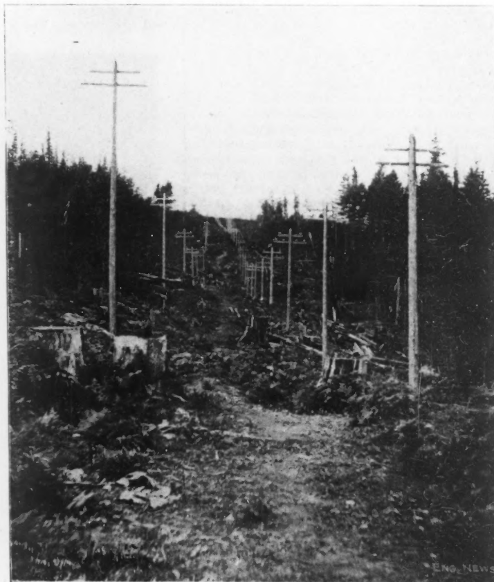
FIG. 12.—VIEW ON TRANSMISSION LINE.
