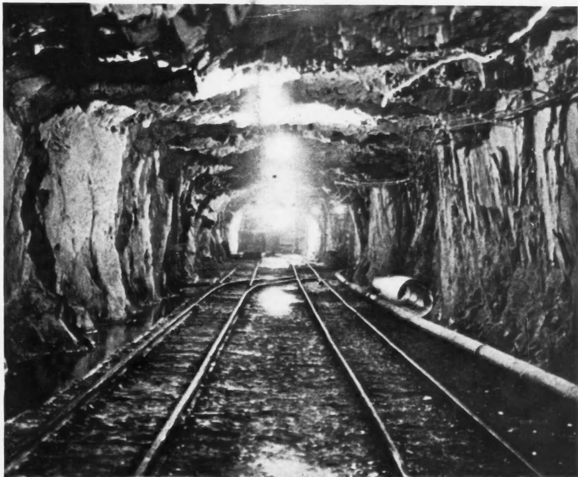
The Star Crosscut, in the Coeur d'Alene district, Idaho, which will connect the Hecla Mine with the Morning, about 8,000 ft. away, and facilitate the working of the Star ground
