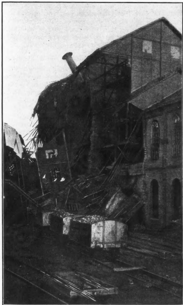
COAL-WASHING PLANT IN FRENCH COAL FIELD AFTER DESTRUCTION BY GERMANS
