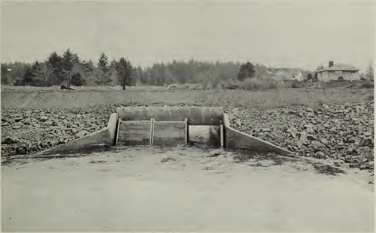
Photo 38.--These flood gates on the Skipanon River are part of the P. L. 566 project near Warrenton. SCS photo
