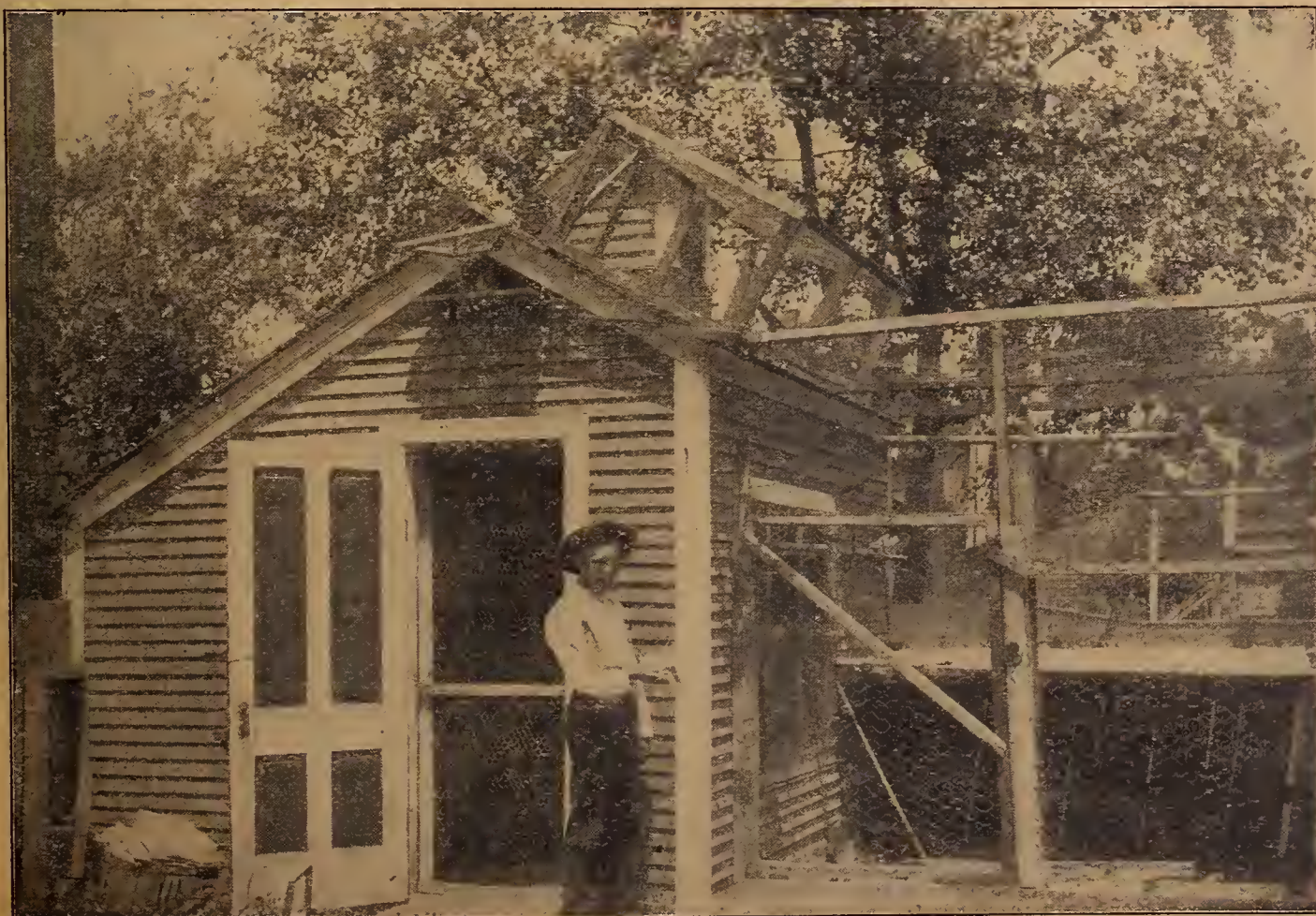
MASTER HOMER WINCH'S SQUAB HOUSE
