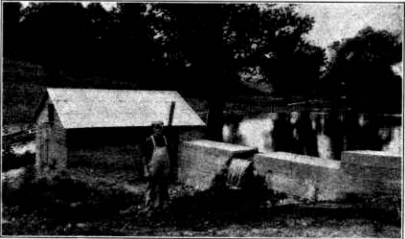
FIGURE 3.—Hydroelectric plant built in Pennsylvania in 1925. Drainage area 2.4 square miles, head 6.9 feet, steel overshot wheel 6 by 2½ feet, generator one-half kilowatt, power house 13 by 15 feet. Cost of machinery $385, materials $325, labor $356, wire $64, miscellaneous $128, total $1,258. Estimated cost of current, including interest, depreciation, taxes, insurance, attention, and repairs, $174 per year
