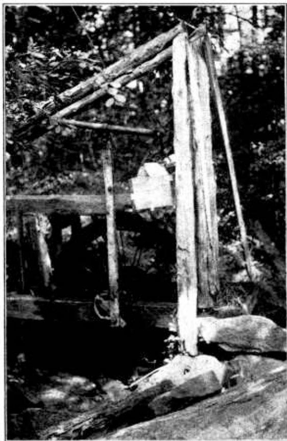
FIGURE 1.—Inexpensive overshot wheel and homemade counterweight rocker arm with draft wire for transmitting the power. Virginia
