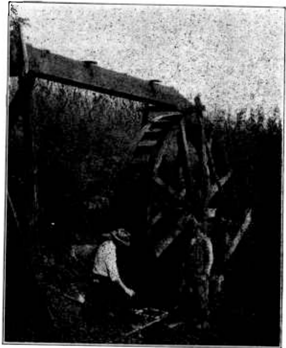
FIGURE 2.—Simple wooden flume and overshot wheel with chain drive to a pump lifting spring water to a mountain home. North Carolina
