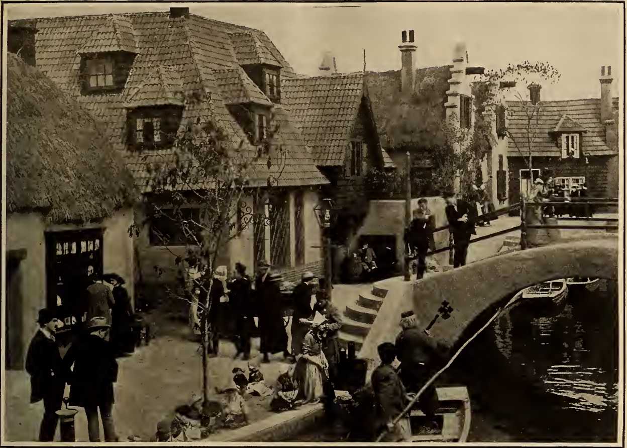
TRIANGLE This elaborate Dutch village was constructed at Culver City, Cal., for the production of "Wooden Shoes," in which Bessie Barriscale was the star. Its cost would have been prohibitive, even for a movie set, were it not that such a structure is convertible.
