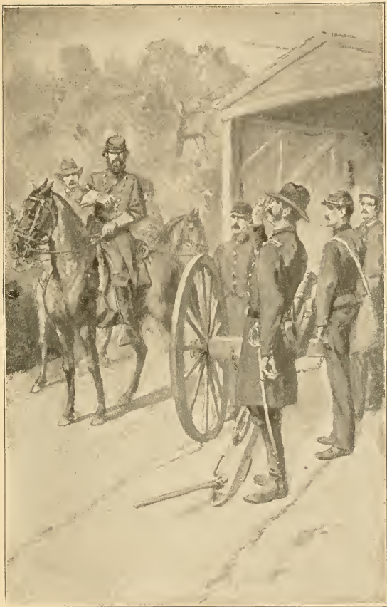
JACKSON AT PORT REPUBLIC BRIDGE
