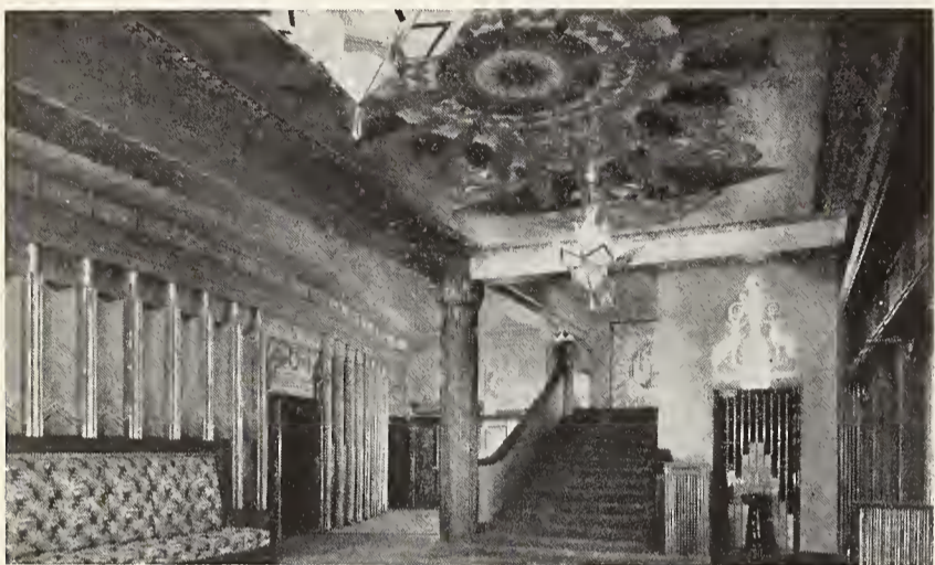
Figure 2.—Same lobby as in Figure 1 after remodeling.
