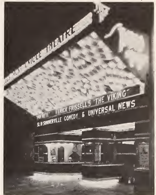
Figure 5.—As remodeled—cost today, $1,500.
