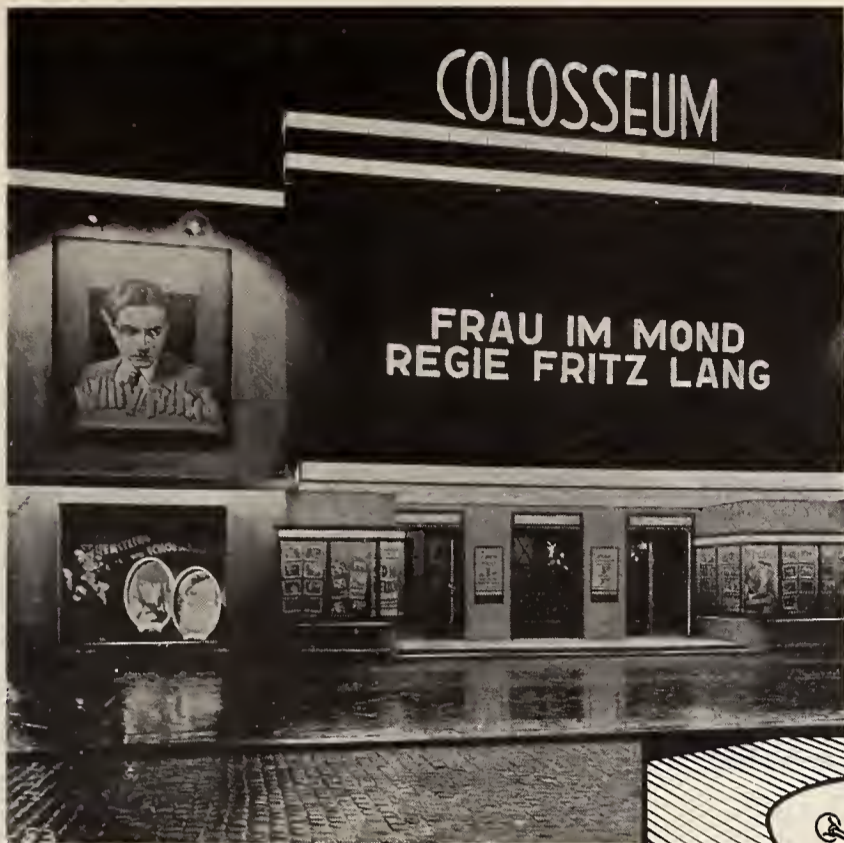
The Colosseum theatre in Berlin and how it sells itself with light. In addition to luminous panels and a glass-faced block letter sign is a marquee completely of diffusing glass. Posters are a feature of the theatre front rather than an afterthought.
