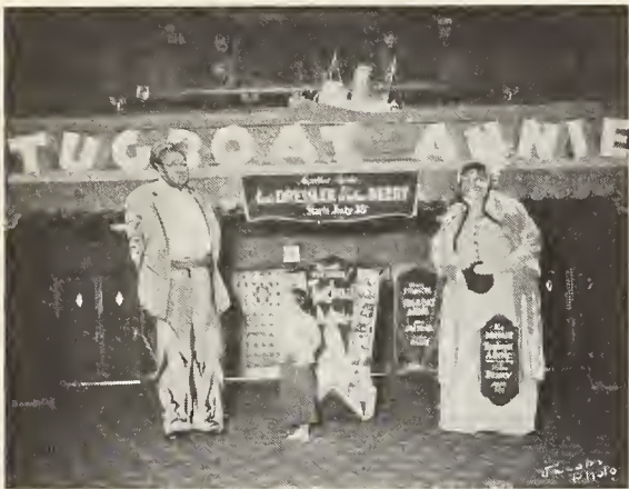
Enlarged Lobby Cutouts
