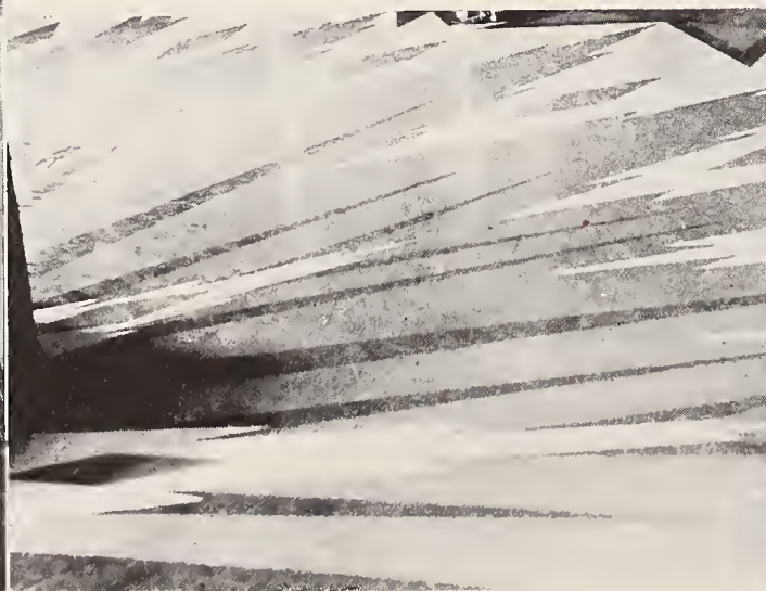
Figure 9.—Terrazzo floor of marble chips in cement.
