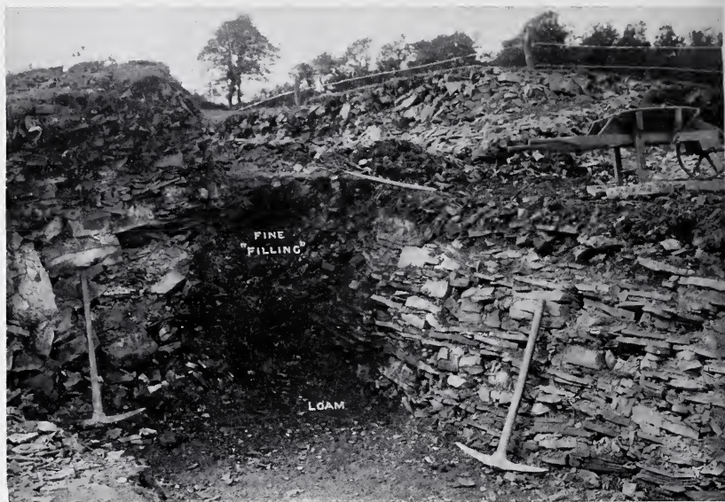
FIG. 1.—View from the S.E., showing the “fine filling,” consisting of mould and small thin pieces of lias, placed against the wall for protection.
