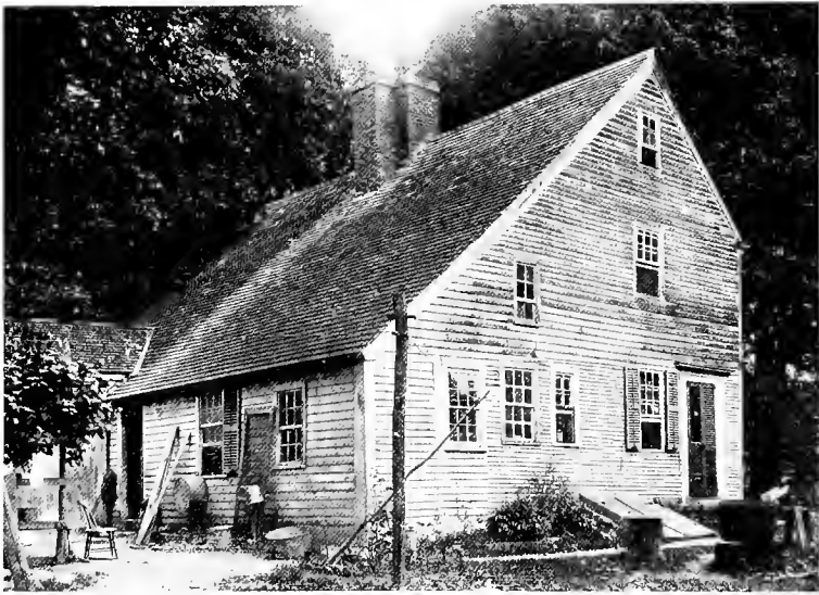
An old "B" plan house showing a "stack of chimneys." In the old times, "chimney" meant flue, and in the topping out each flue was apt to show as a unit
