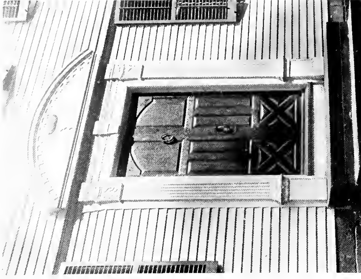
This is essentially a craftsman doorway, which has employed certain unarchitectural inventions in the caps and pediment. Note the braced double door
