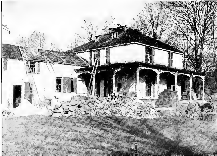
Before alteration, this "gem" of a piazza nearly girdled the house, cutting out direct sunlight from all the lower rooms. Otherwise the block of the structure had not been tampered with to any extent
