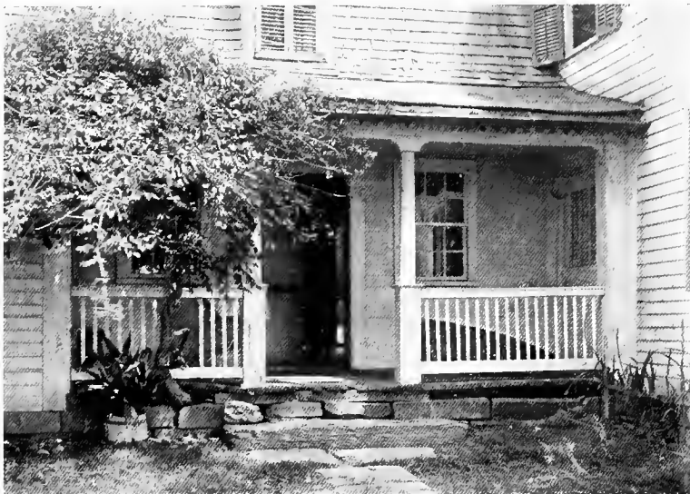
A rear piazza in the Connecticut valley, with the "kicked" roof. The problem is one of framing and was solved without the aid of the turned column
