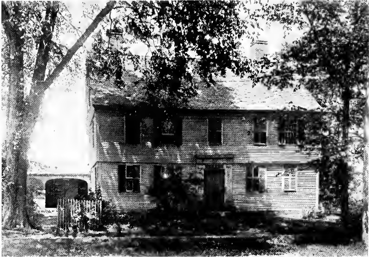
One of the Ellsworth houses at Windsor, Vt. (about 1750). This preserves the tradition of the Pre-Georgian overhang on each story. Modified "I" plan
