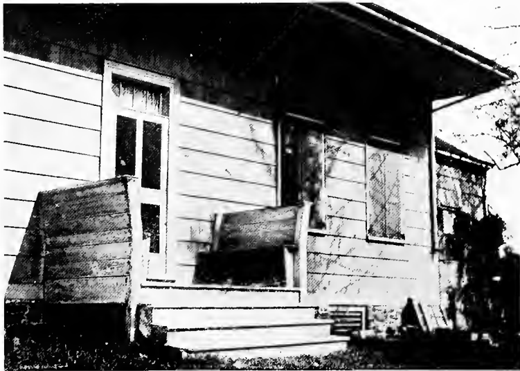
The "stoep" of a Dutch house on Long Island, N. Y. This is a good and simple treatment, with excellent constructional qualities
