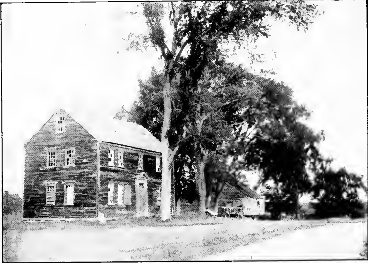
If the house sets true and straight and the roof has no sag to it, it is well worth the time and trouble of examination, regardless of outside covering
