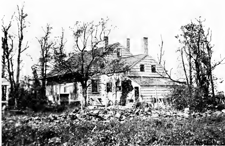
Old Dutch house on Long Island, N. Y. This has the usual overhang and "kick," with typical "stoeps" on either side. Modified "J" plan
