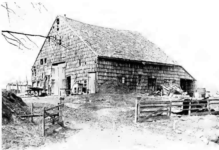
An old Long Island barn which follows the Saxon tradition in having the end door. The design as it stands is good and also effective with the long shingles
