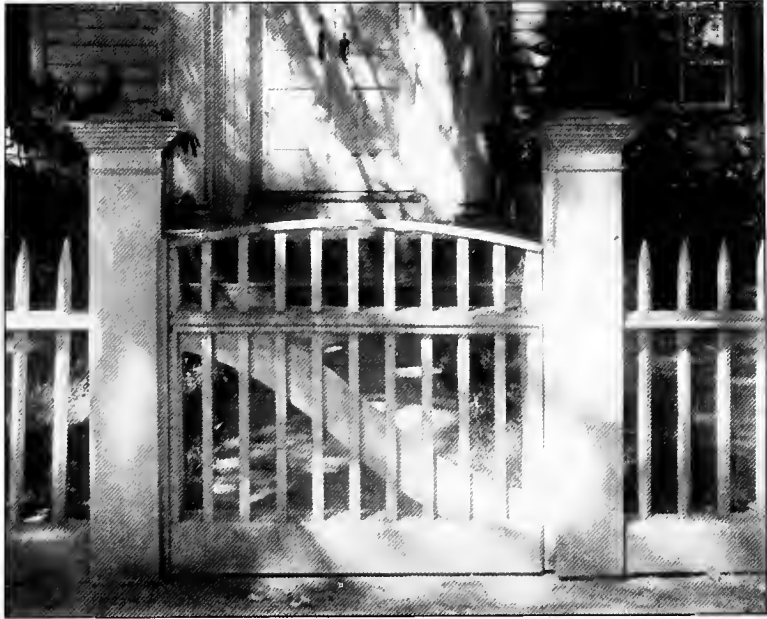
A new gate in an old fence, which anticipates the possible breaking of pickets by a cap and likely sagging by the introduction of a brace
