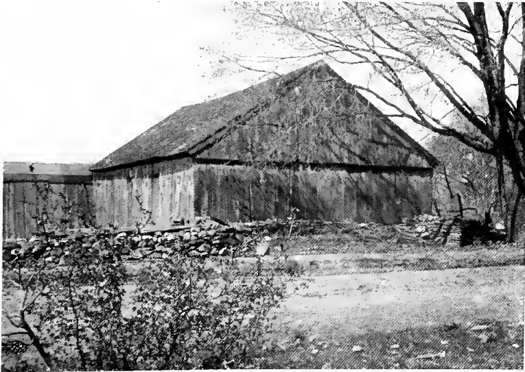
A Connecticut barn which follows the tradition of the Pre-Georgian type. It is boarded vertically and the aisle is from side to side after the English fashion
