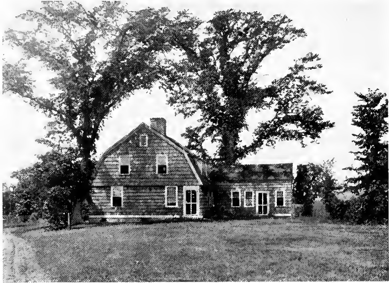
An old Connecticut house of the gambrel type which retains the tradition of the overhang of the Pre Georgian style. (C. L.)
