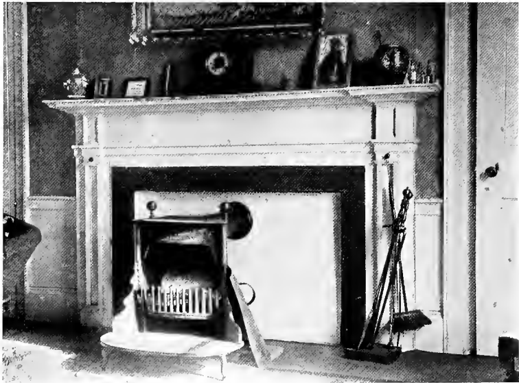
A New England mantel of simple but interesting design. The dado and door trim is also good. The Franklin stove is worth while as a chamber heater
