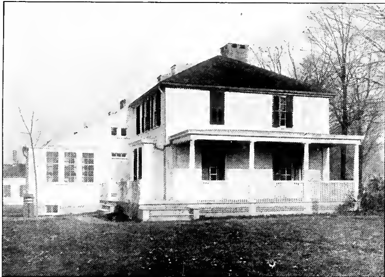
The substitute for the old piazza was a bit more in keeping with the period of the house. The "kick" to the roof of the "outdoor" room is a localism probably borrowed from the Dutch
