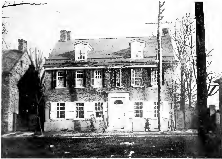
"Grumblethorp," Germantown, Pa. Showing a slight modification of central door arrangement. Variation of the "F" plan
