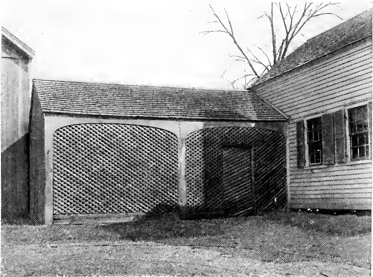
The screened woodshed has some practical advantages, but the lattice should fall back of the outer wall face several inches to give the best results
