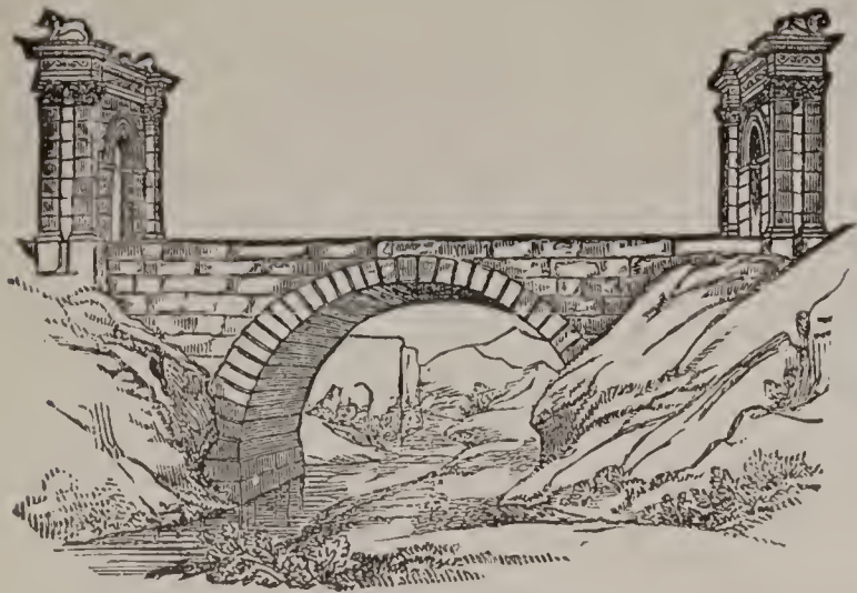
FIG. 6.—Bridge at St. Chamas.
