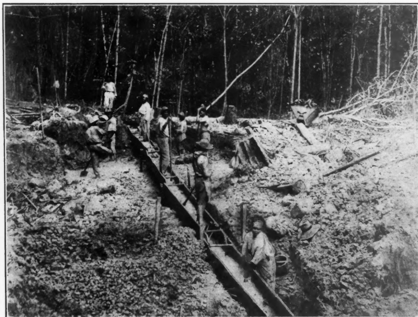
SLUICING PLANT ON THE ELYSEE PLACER
