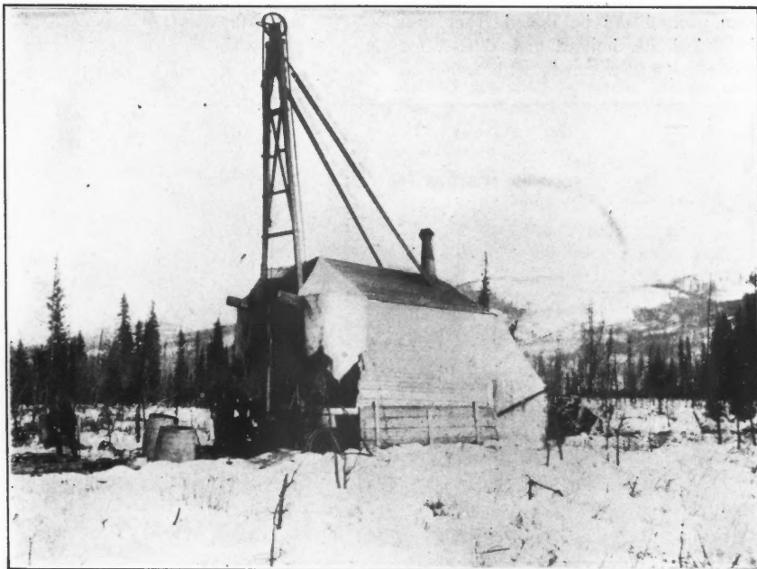
DRILLING IN WINTER, INDIAN RIVER
