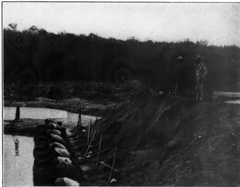
WASHING DIAMOND GRAVEL AT AGUA FRIAS
