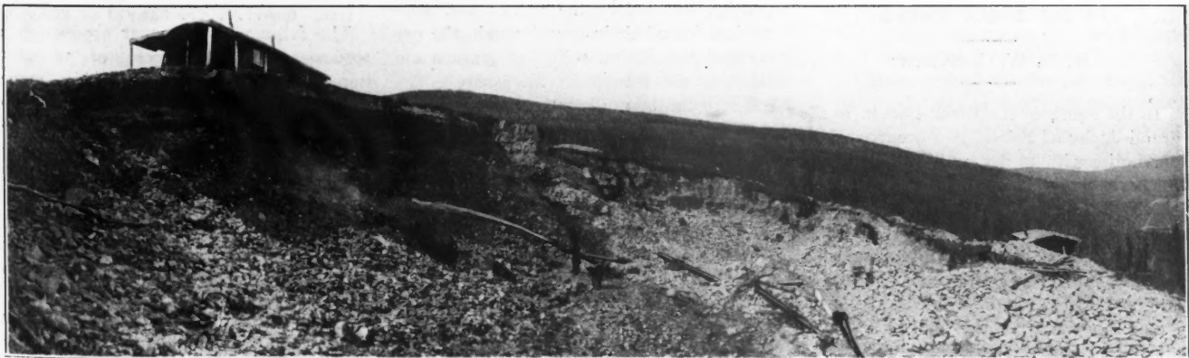
A SMALL HYDRAULIC INSTALLATION
