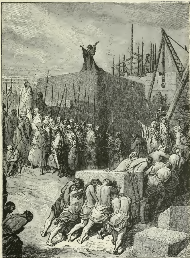
THE REBUILDING OF THE TEMPLE.
