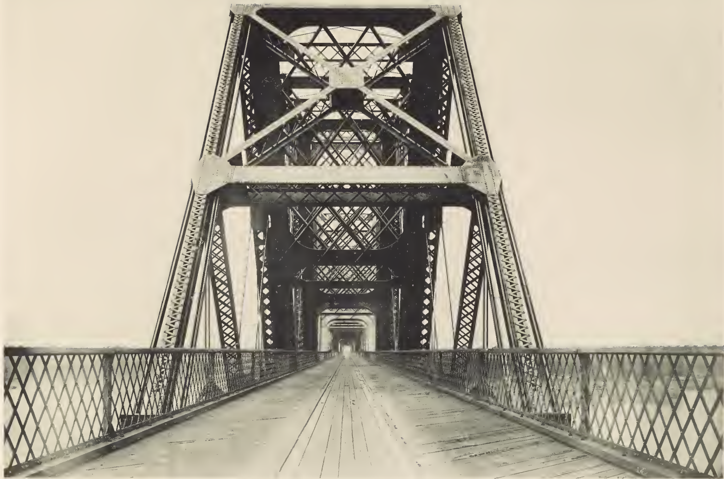
THE MEMPHIS BRIDGE
