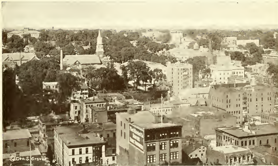
View over busy Main Street at Court Square, looking to Armory Hill and United States Arsenal. Prominent in this view can be seen the City Library, St. Michaels Church, Wesson Hospital, and many other important buildings in the educational and religious center. State Street leading on to Boston is in the center of this view.
