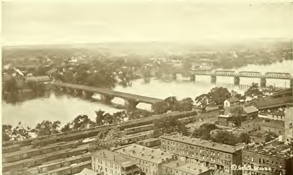
View to West Springfield across the Connecticut River showing the Old Toll Bridge, built in 1816, and Boston & Albany Railroad Bridge. Beyond West Springfield is the beautiful hill country ending in the noted Berkshire Mountains.
