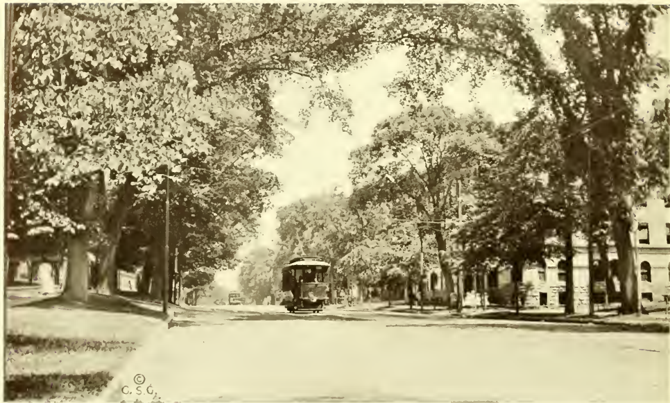
VIEW UP STATE STREET, AT CORNER OF BYERS STREET.
