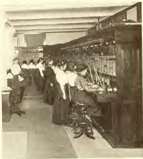
PART OF OPERATING ROOM.
