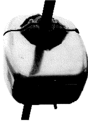
Figure 5-10 Conductor temperature sensors installed on a steel-reinforced aluminum cable (ACSR) conductor. The sensor communicates using a cell phone modem.
