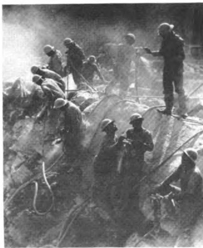
Wet drilling should be used in many stone-cutting operations to protect the workers from harmful dusts. Cold weather and inaccessible water supplies make it very difficult at times.
