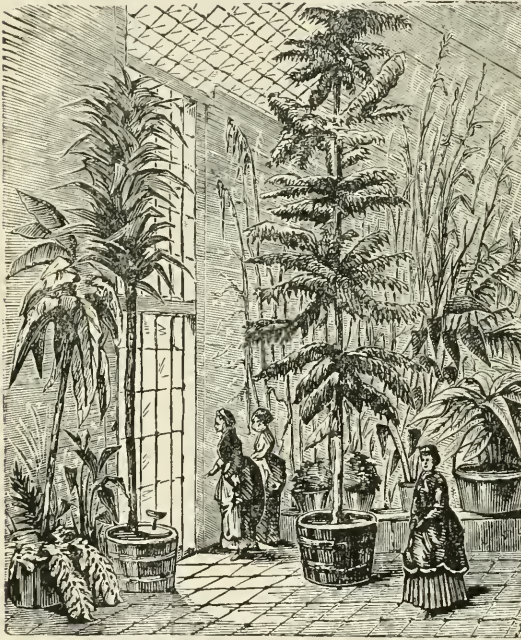
INTERIOR OF PLANT HOUSE.
