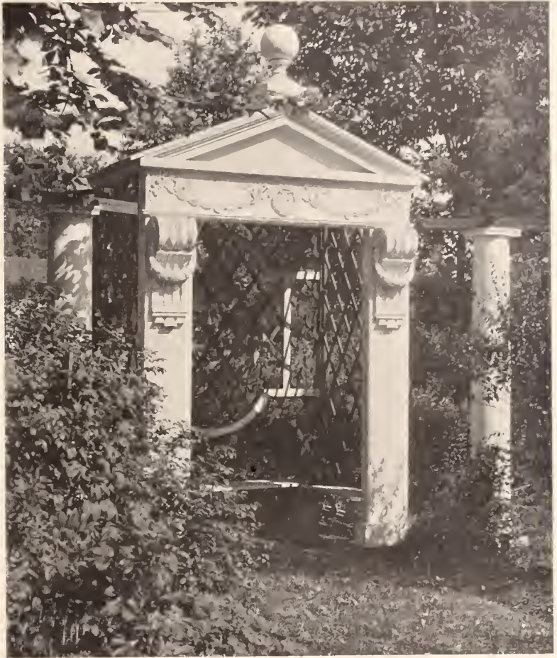
The Summer House at the Terminal of the Walk has a Stately Entrance with Massive Pilasters at Either Side, Supporting a Pediment
