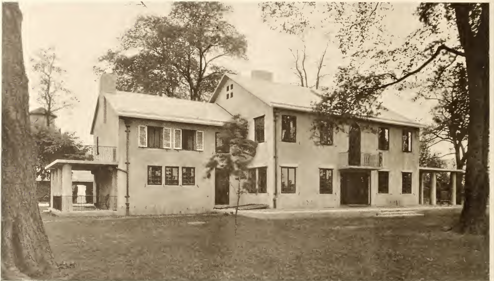
4—The House, Showing the Roof of Reinforced Concrete. The Kitchen Extension and the Servants' Porch are Excellent Features of the House
