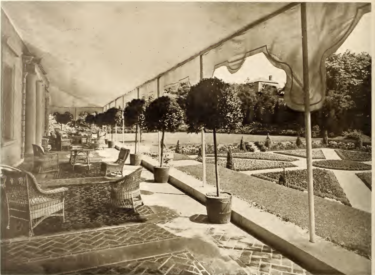
The Terrace Overlooking the Garden is Paved with Brick and Shaded by an Awning
