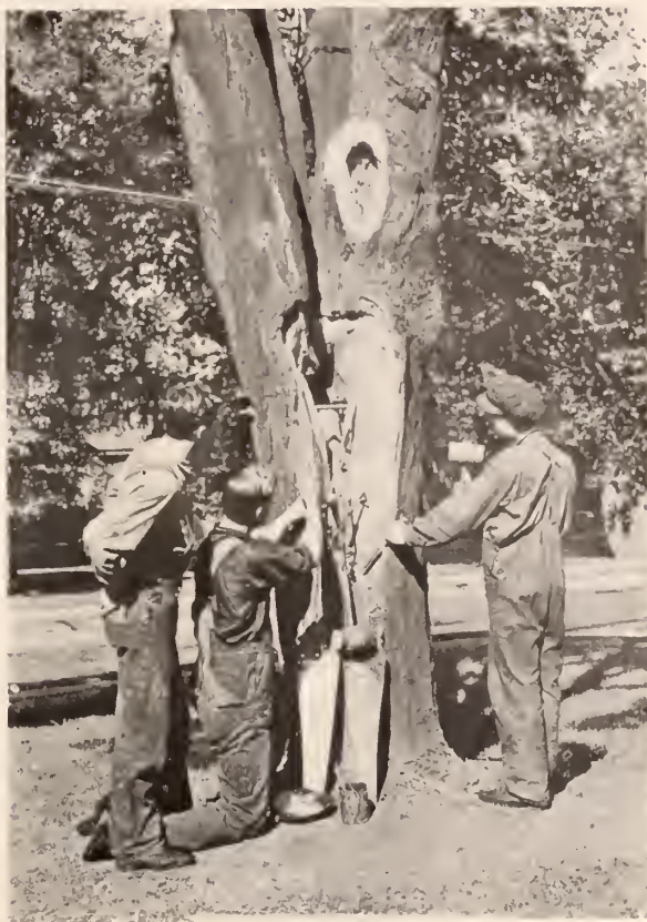
Splitting Means Decay
