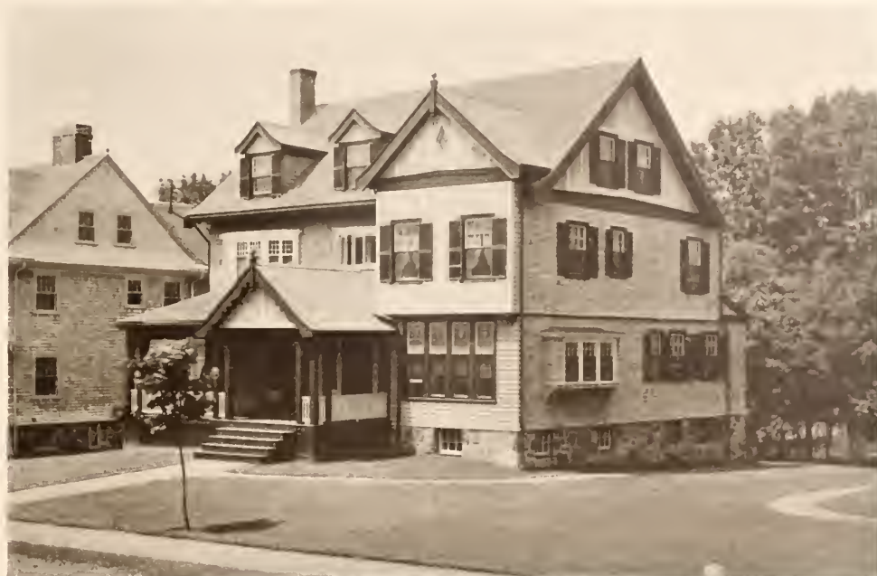
1—A House of Good Style with Shingled Sides, and Half-Timbered Gable Ends
