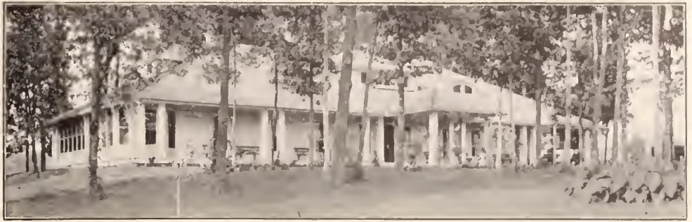
Country Home of Rev. J. Wilbur Chapman, Winona Lake, Ind. Supplied with water by the Kewanee Water Supply System
