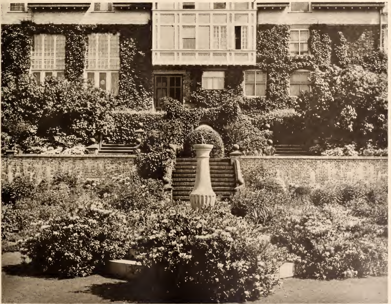
The House Rises as a Screen, with the Terraces Below. The Vine-Clad Walls Harmonize Finely with the Rich Vegetation of Garden
