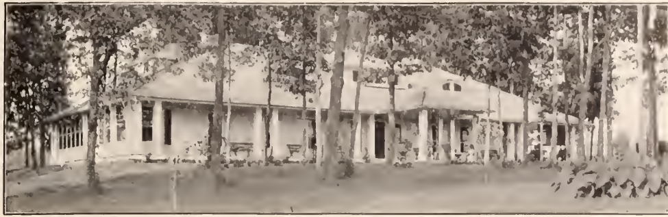
Country Home of Rev. J. Wilbur Chapman, Winona Lake, Ind. Supplied with water by the Kewanee Water Supply System
