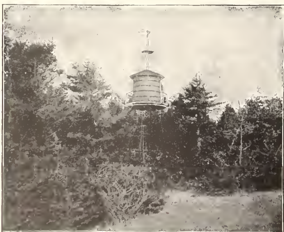
27 ft. Tower, 3,000 gal. Tank, furnished Mr. J. F. Perkins, Portland, Maine
