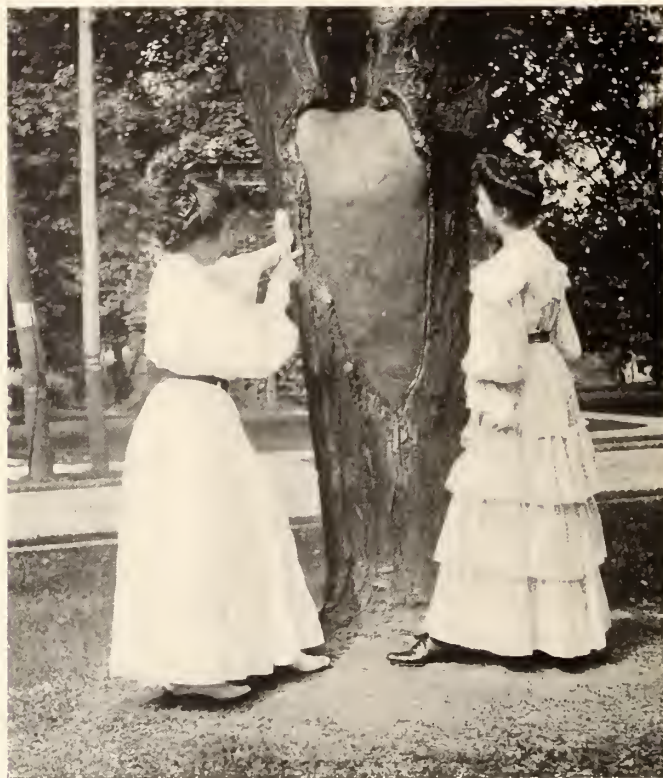
A Shell Filled with Cement to Preserve Life
