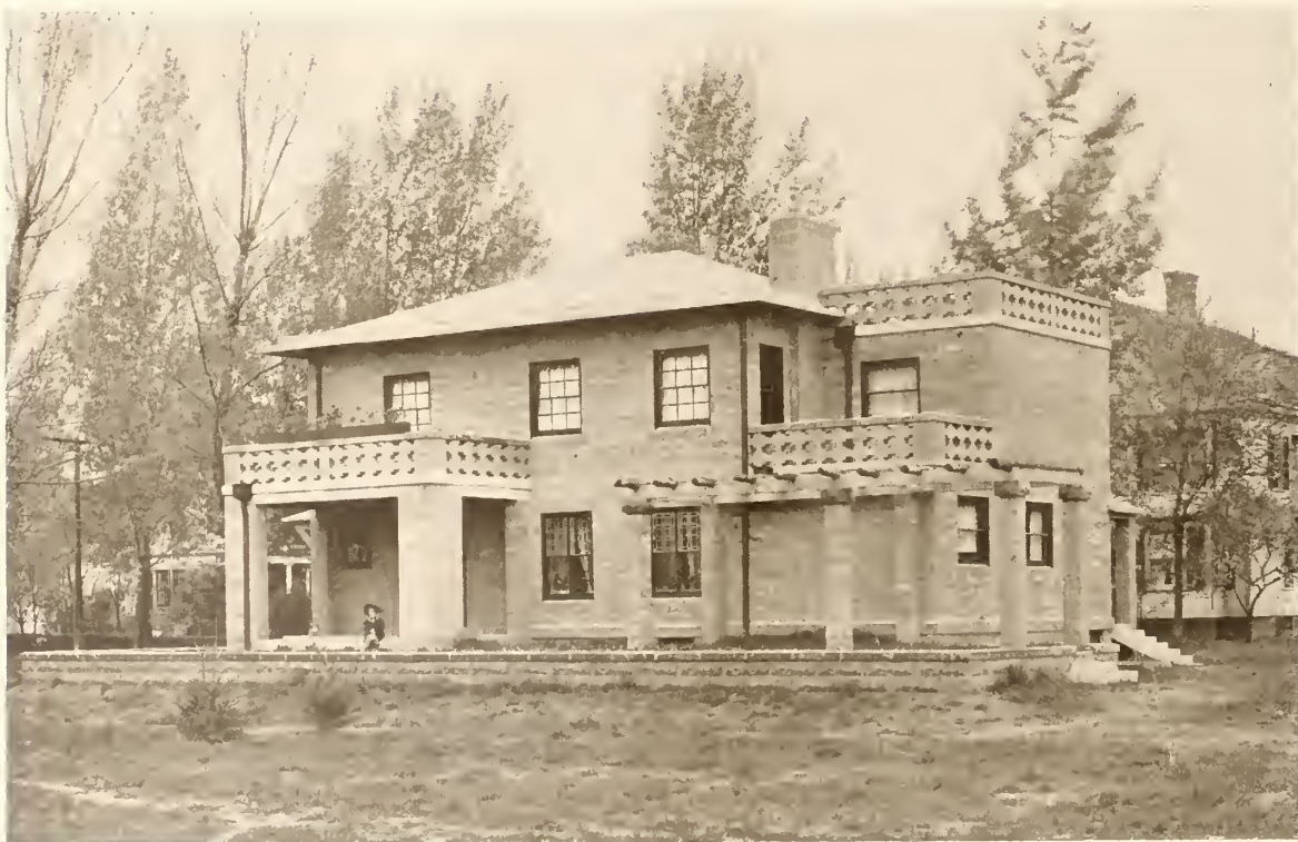
14—Skilled Labor is Not Required to Make the Hollow Concrete Block of Which the House is Built
