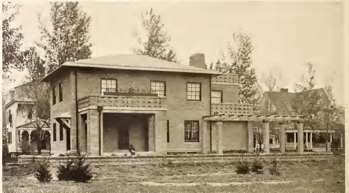
12—House of Mr. W. J. Steel, at New Dorp, Staten Island, is Constructed with Hollow Block Walls and Reinforced Concrete Roof and Floors
