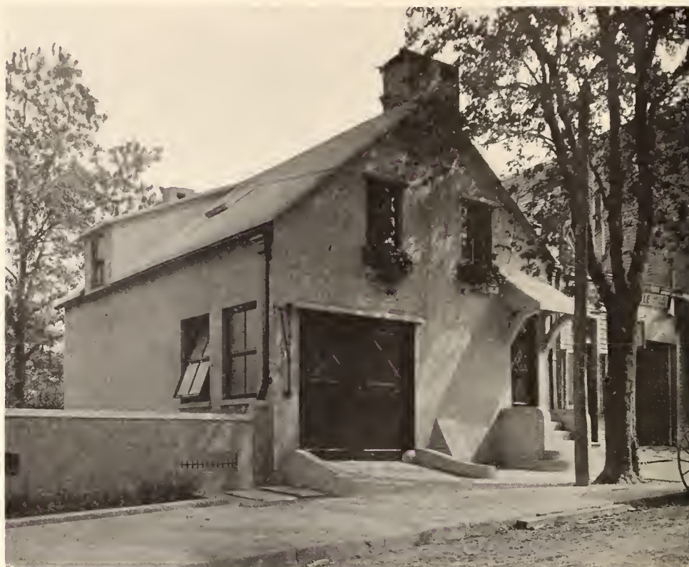
A Garage Constructed of Reinforced Concrete throughout Walls, Floors and Roof
