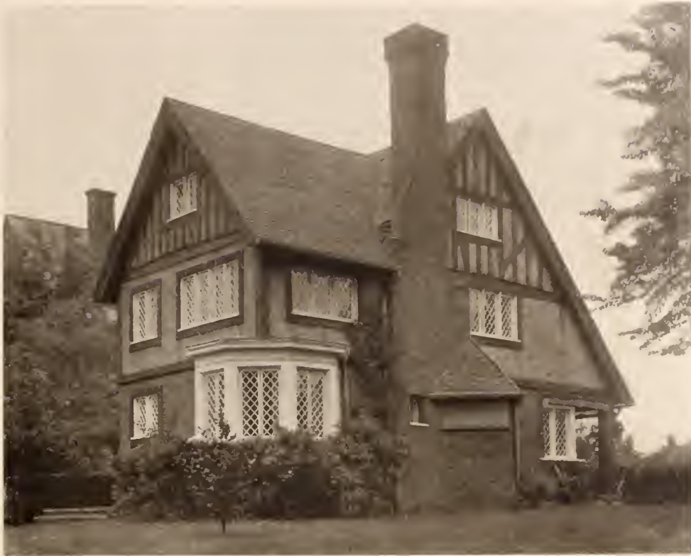
The Brick Chimney and the Lean-to Roof are the Architectural Features of the Side of the House
