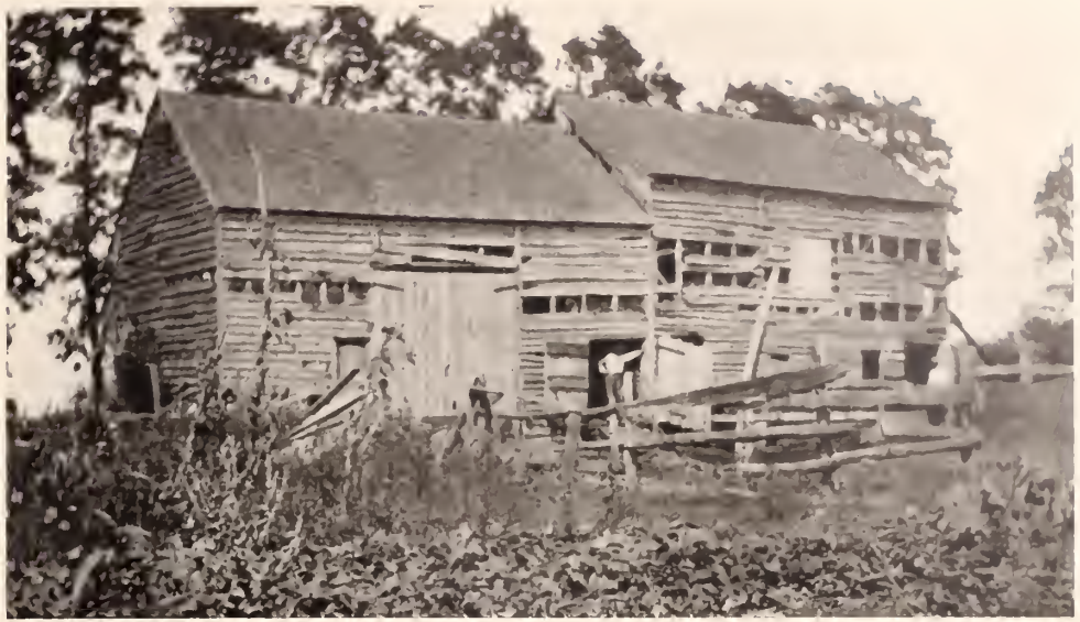
Another View of the Barn
