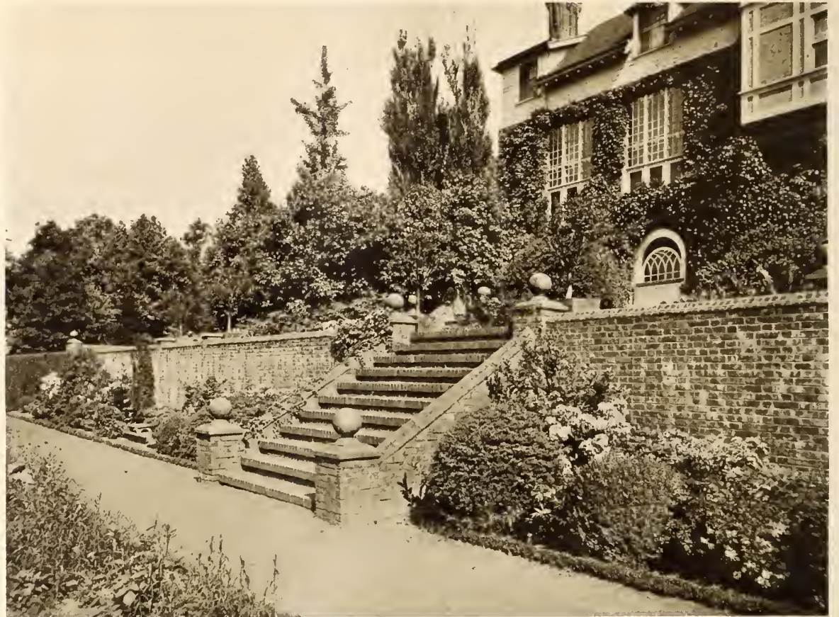
Brick Steps Descend to the Lower Terrace; Above is a Vine-Covered Archway with Steps on Either Side
