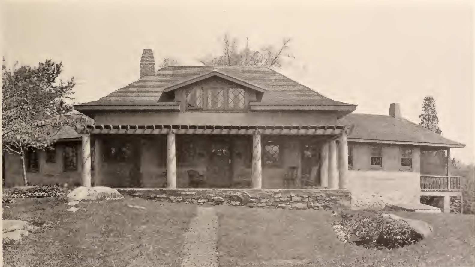
21—The House of Mr. Bassett Jones at Bryn Mawr Park, New York, has Reinforced Concrete Walls Finished with a Pebble Dash, and a Shingled Roof Stained a Moss Green with Good Effect
