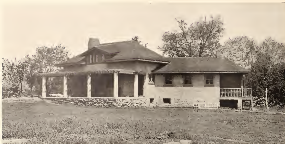
22—An Annexed Extension Isolates the Servants' Quarters from the Main Living Quarters
