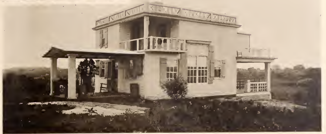
7—Mr. Edward B. Stratton's Italian Bungalow at Clifton Heights, Massachusetts Before and After Its Restoration
