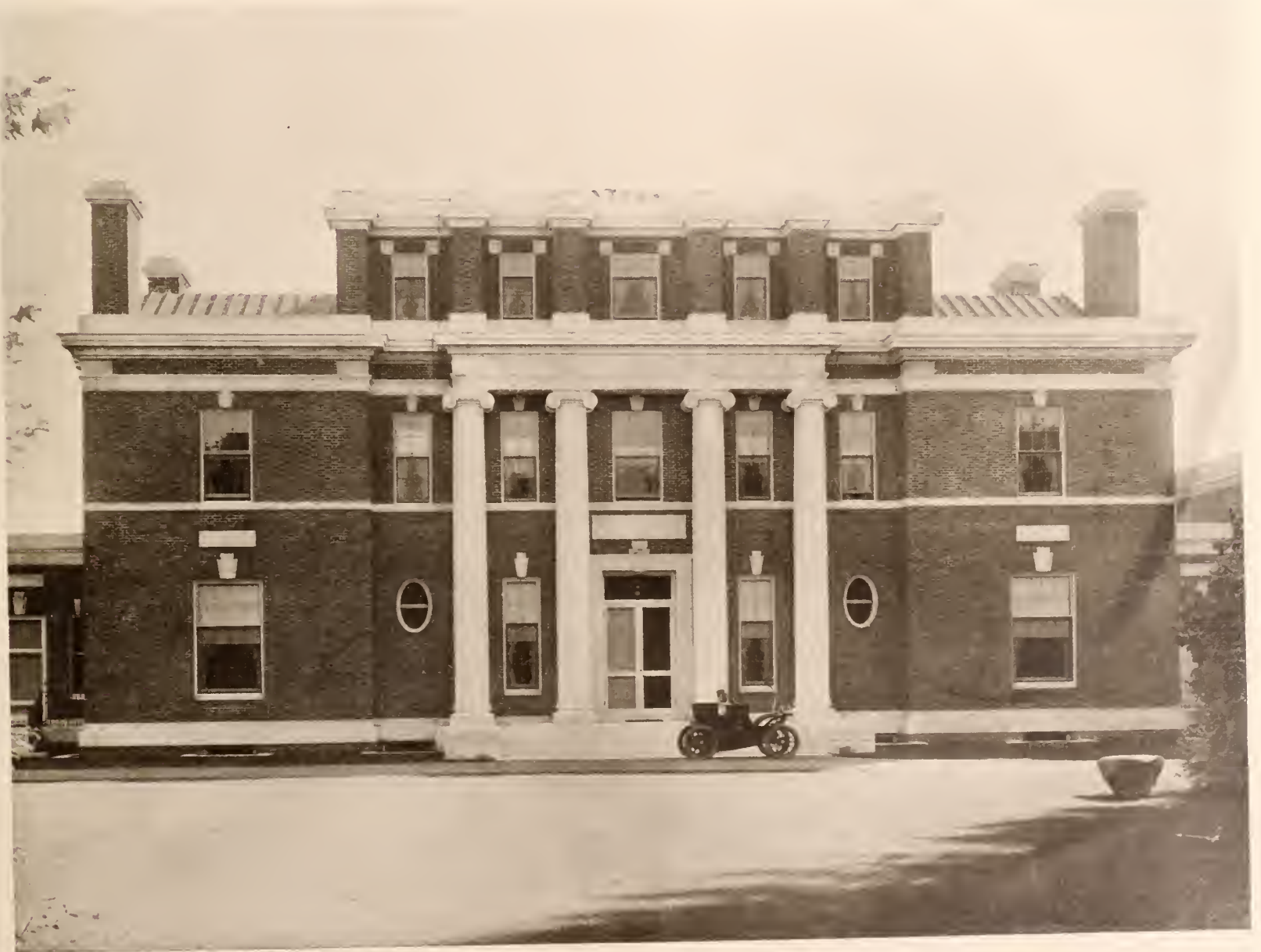
The Entrance-front of the Seaside Home of Mr. T. Jefferson Coolidge, Jr., Manchester, Massachusetts
