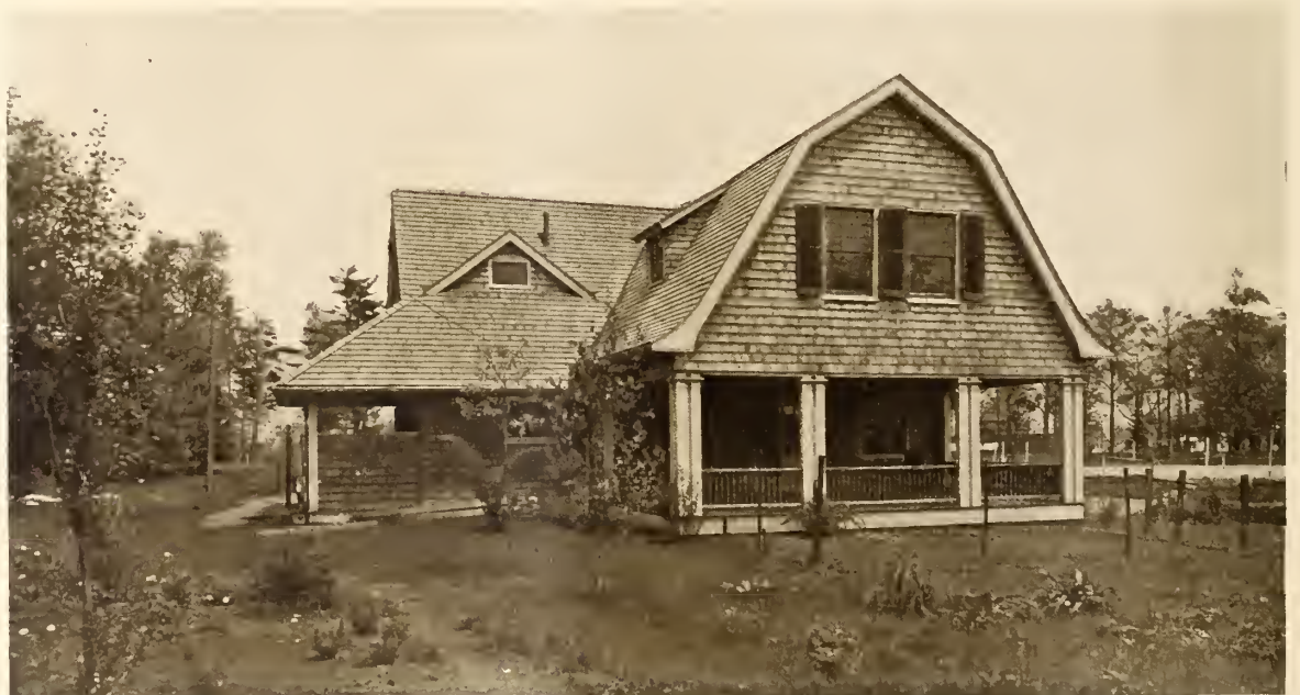
12—A Feature of the Exterior is the Long Gambrel Roof, and the Piazza, which in Winter is Inclosed with Glass
