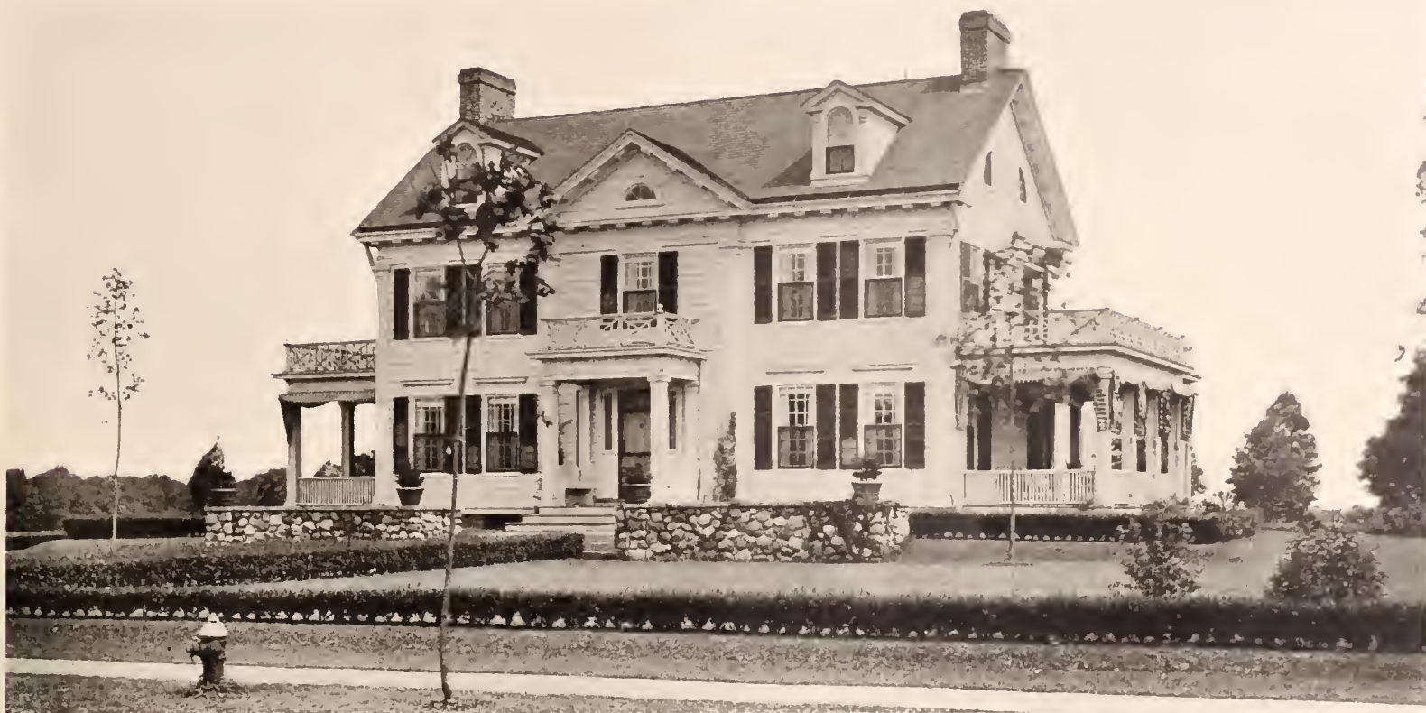
10—A Colonial House of Good Type, with a Central Hall and Rooms on Either Side, Beyond which the Living-porches are Placed
