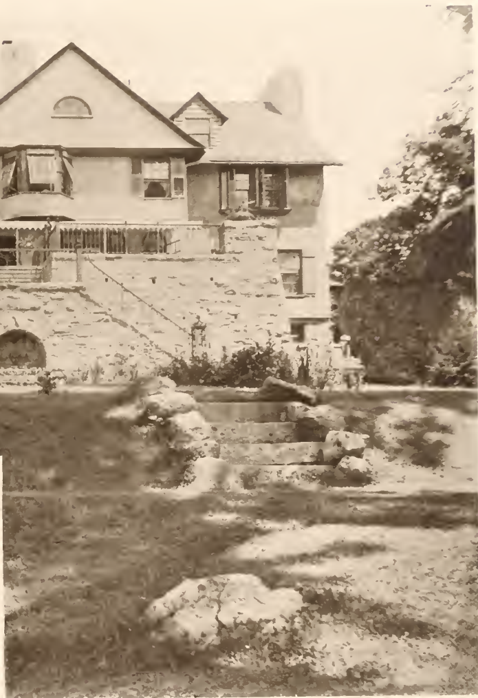
The Terrace Front and its Massive Stone Base
