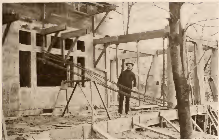
6—The Construction of the Columns to the Piazza
