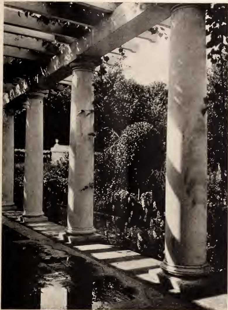
Looking Through the Pergola
