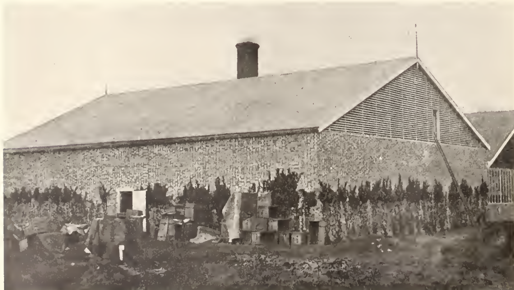
A Cold Storage Building in Which Plants are Retarded. In this Building Five Million Lily-of-the-Valley Plants Were Retarded in a Single Year
