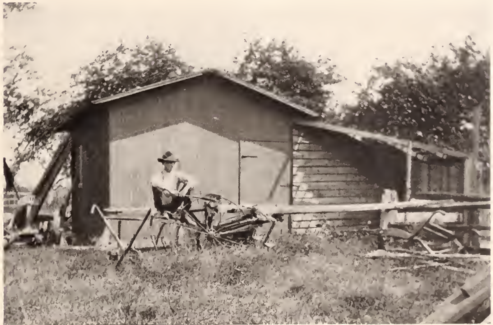
The New Outbuildings Completed the Second Year
