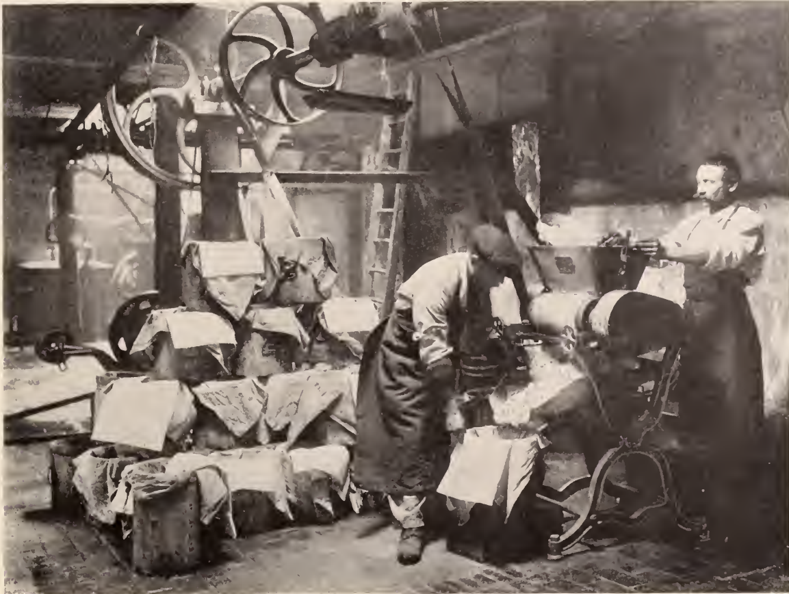
4—Kneading the Mass with a Roller-kneading Machine
