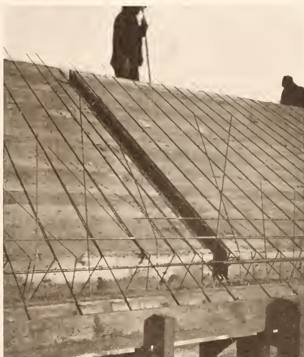
7—The Forms for the Roof, Showing the Reinforcement Rods in Position Ready for the Concrete
