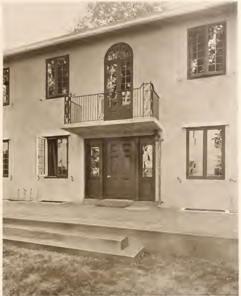
1—A Broad Doorway with Windows on Either Side, and a Balcony Inclosed with an Iron Railing
