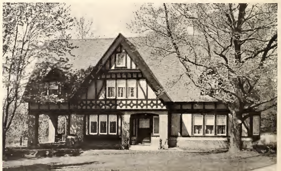
9—Harvard Brick, Beams and Stucco are the Materials Used for the Exterior of the House
