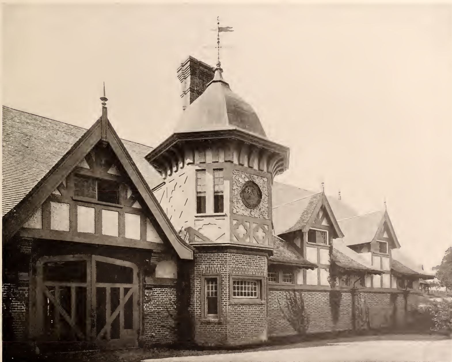
The Stable of James H. Proctor, Esq., at Hamilton, Massachusetts, Has a Picturesque Tower Rising amid the Half-timber Gables
