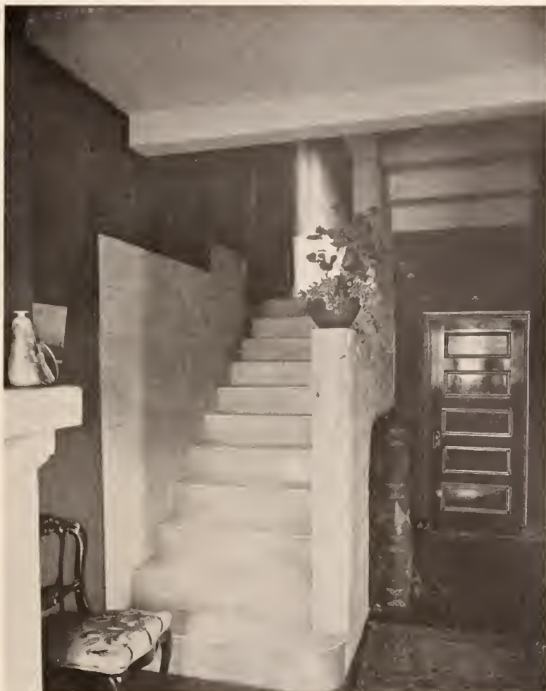
20—The Stairs and Hand-Rail are Built of Reinforced Concrete Treated with a Cement Tint
