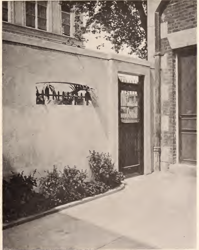
The Gateway from the Street to the Court, and the Wall Built of Reinforced Concrete
