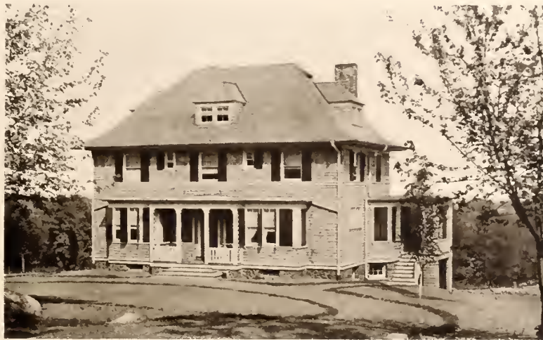
7—This Square-Rigged House Provides Ample Rooms of Good Size It Has a Rubble Stone Foundation with Shingled Walls and Roof. Contains Ten Rooms and Bath
