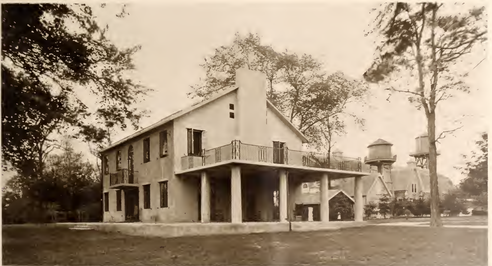
2—The Reinforced Concrete House of Alexander Smith Cochrane, Esq., at East View, New York, Showing the Walls, the Terrace and Finished Columns to the Piazza
