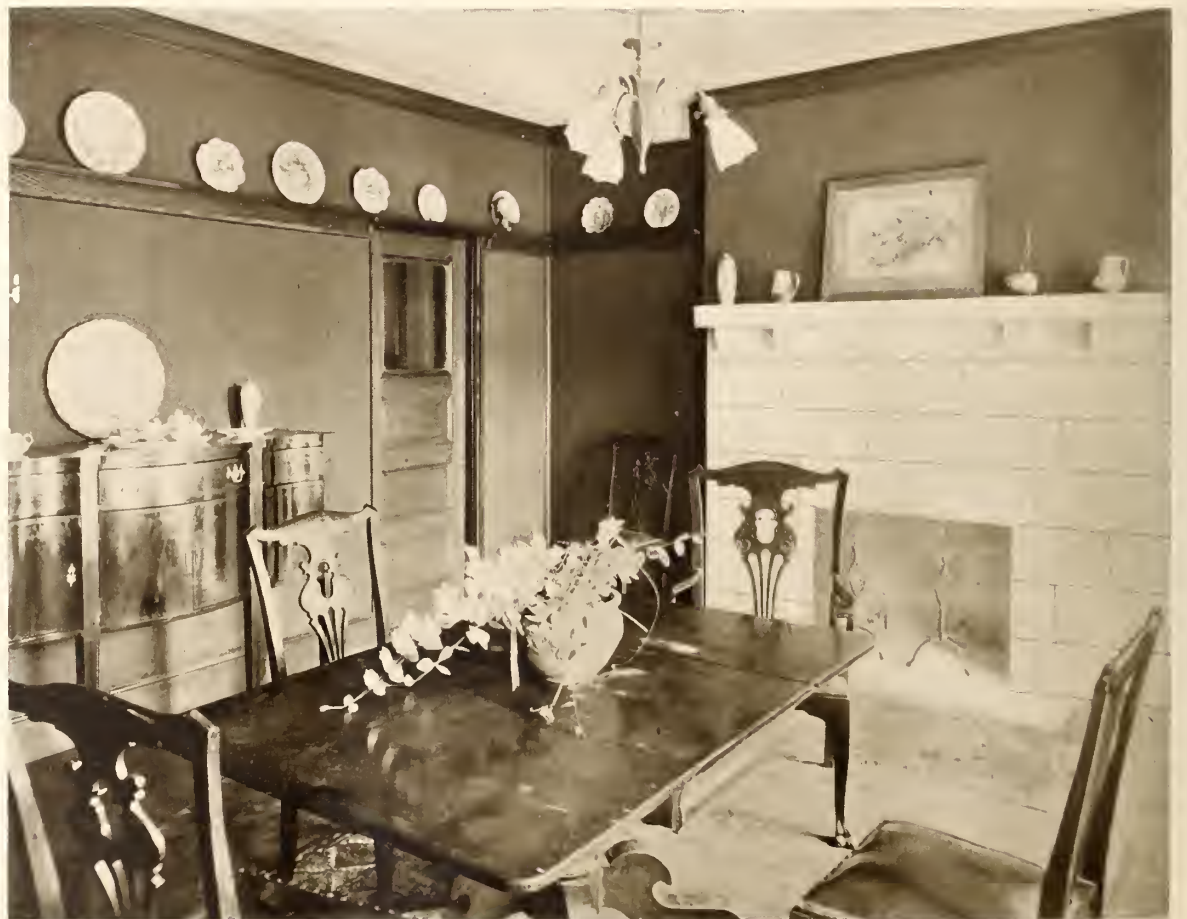
19—The Dining-Room has Wall Covered with Green Burlap, and a Fireplace and Mantel of Concrete
