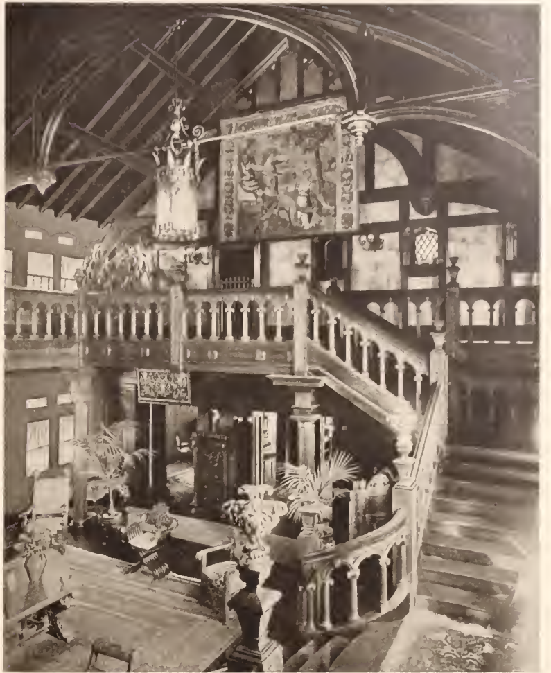
The Hall Has an Open Timber Roof
