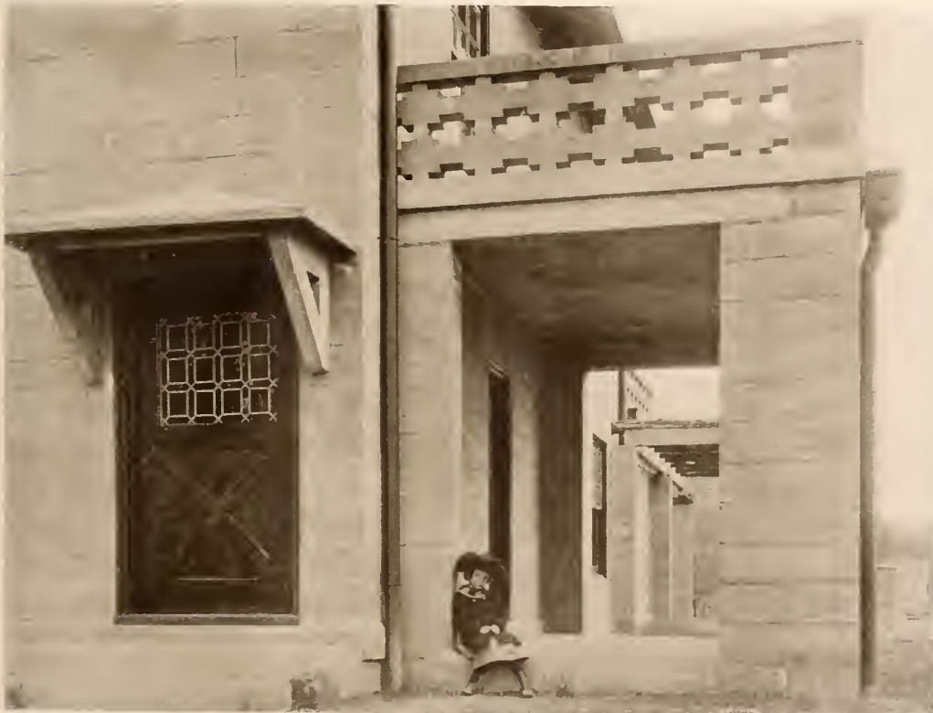
16—The Hood Over the Entrance-Way, and the Columns to the Porch are Made of Reinforced Concrete
