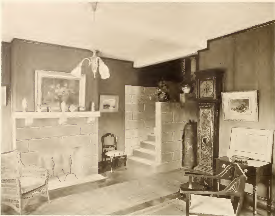
18—The Mantel and Shelf Supported on Corbeled Brackets is Built of Concrete. The Walls are Covered with Crimson Burlap. View Shows Reinforced Beams in Ceiling Which Carries the Floor Above
