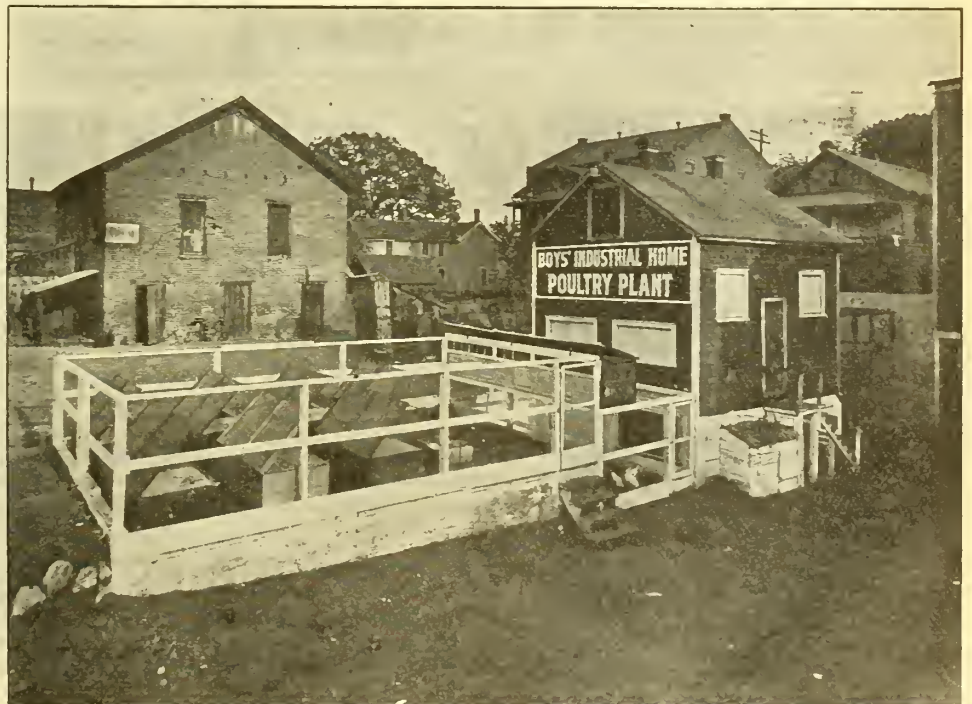
A photographic view of a small successful poultry plant operated by the Philo System
