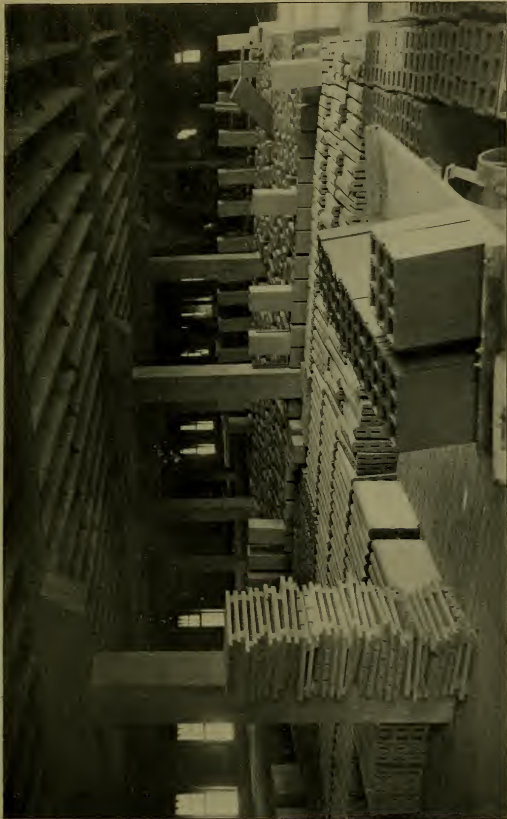
Drying floor for sewer pipe and hollow brick. J. Lyth & Sons, Angola.
