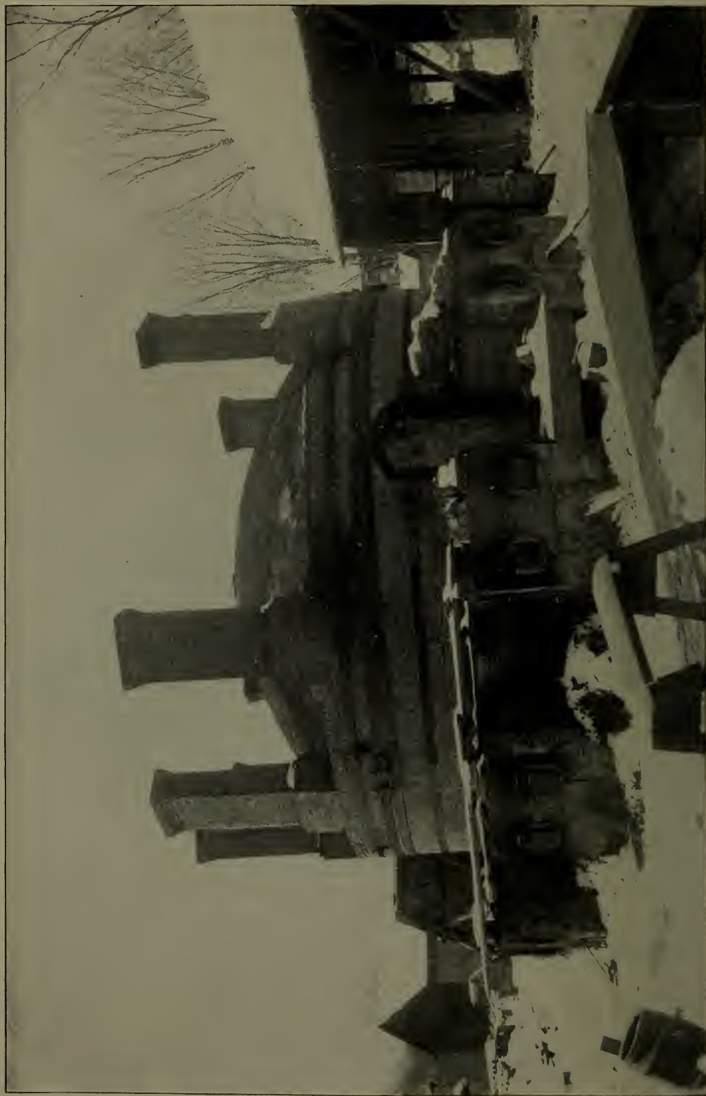
Grath coking furnace used for burning roofing tile. Celadon terra cotta co., Alfred Center.
