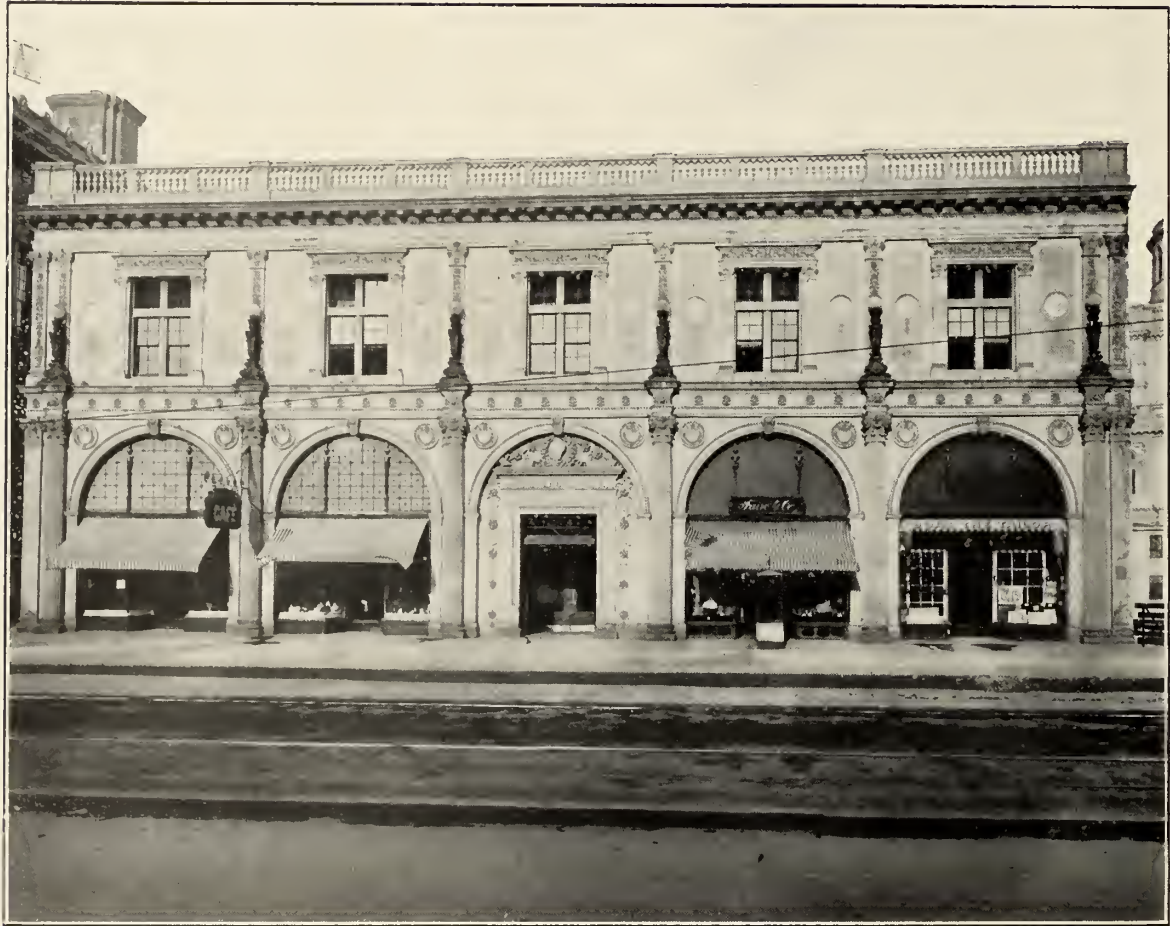
EXTERIOR OF EMERSON COLLEGE
