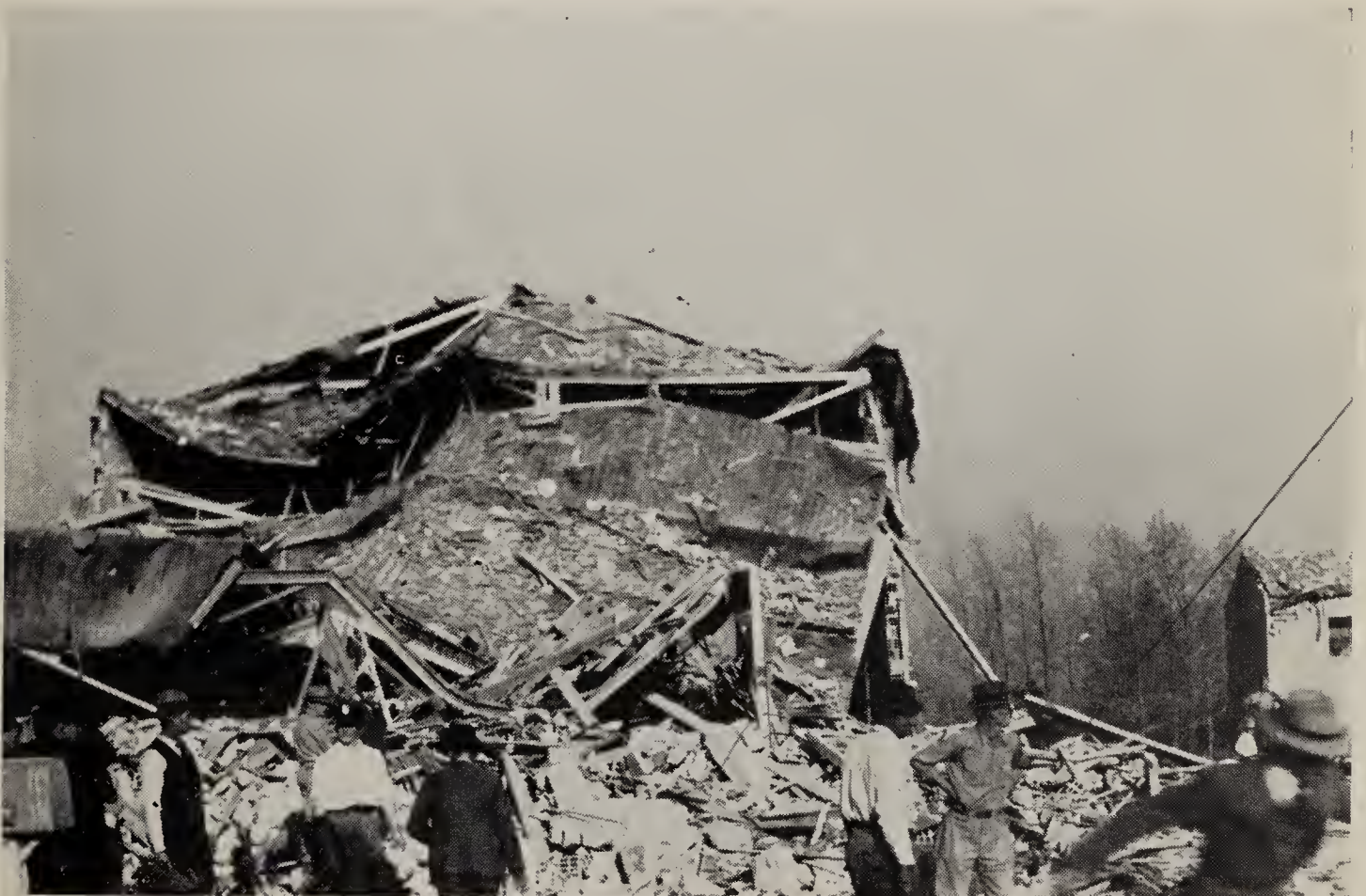
Close-up view showing debris from wrecked auditorium. Note steel girders, brick, and tile.
