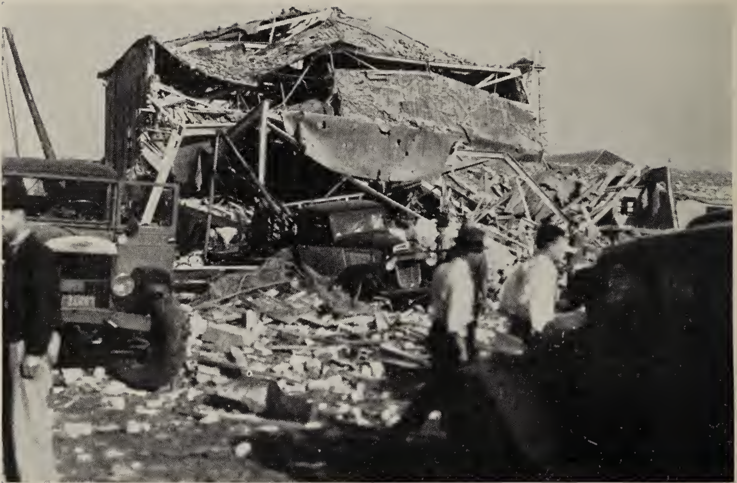
Another view of auditorium while recovery work was in progress. Many bodies were buried in the debris.
