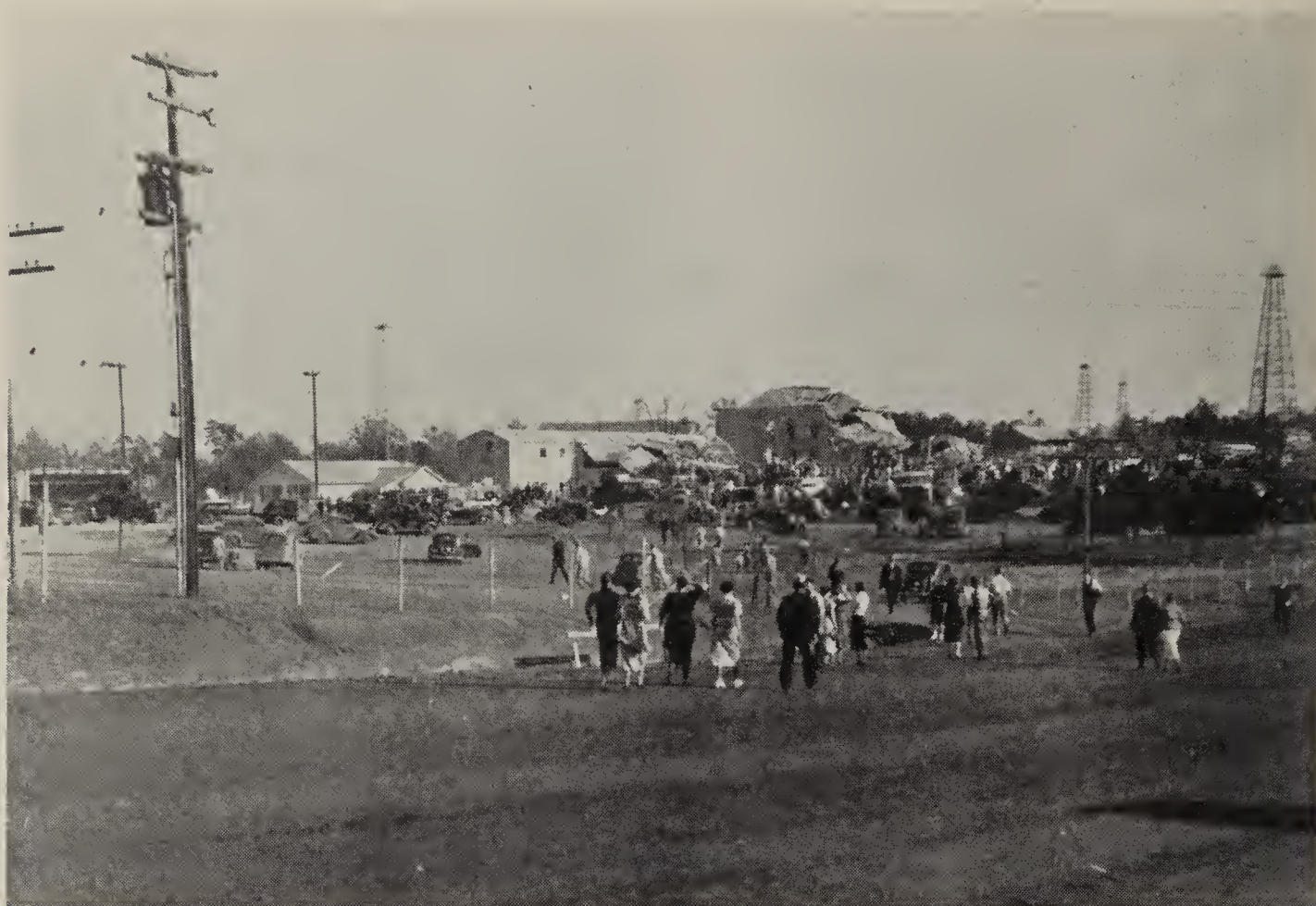
General view approaching school property. Wrecked high-school building on left, auditorium in center, graded school at right. Note oil and gas wells adjoining school property.
