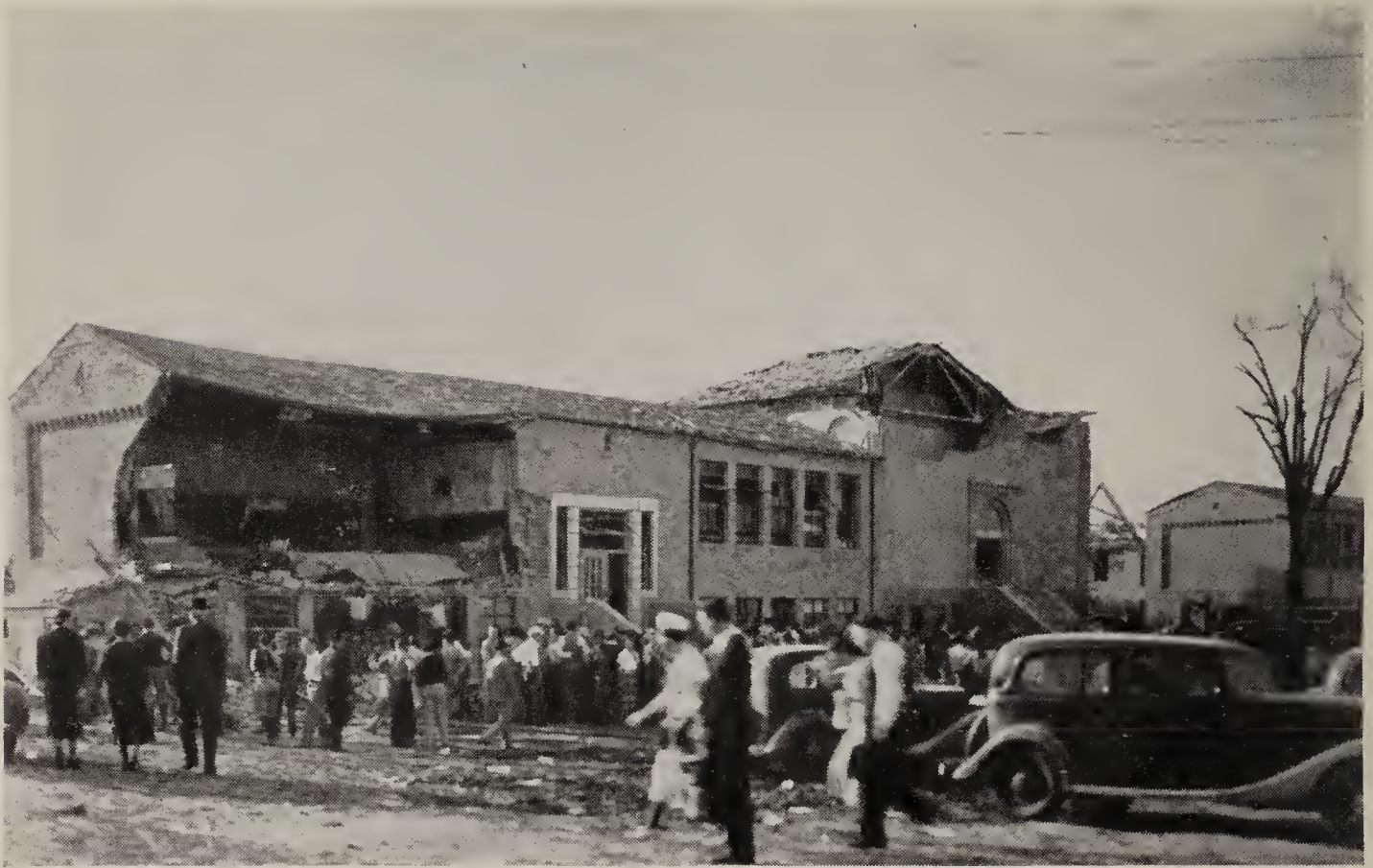
View of graded school and auditorium after explosion on March 18, 1937; approximately 300 children were killed in this section of the building.
