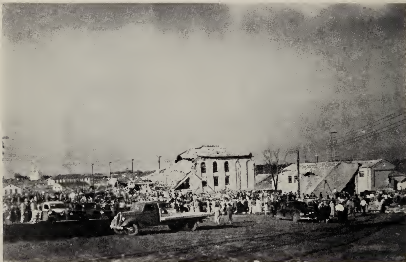
View showing damage to auditorium in center and graded school on right. Note near-by oil and gas wells and athletic-field stadium back of auditorium.
