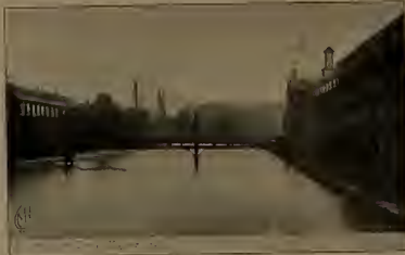
THIRD LEVEL CANAL.
