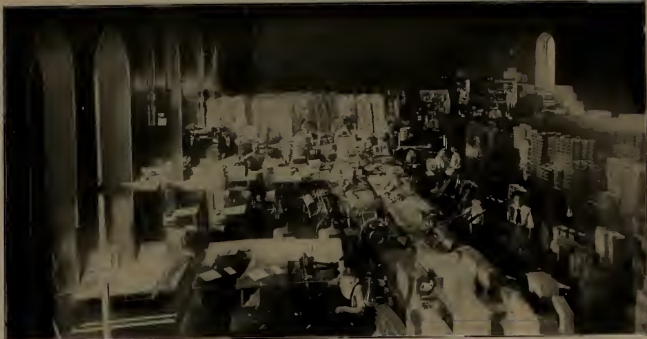
INTERIOR VIEW WHITE PAPER BOX COMPANY
