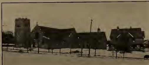
St. Paul's Episcopal Church, Parish House and Rectory.
