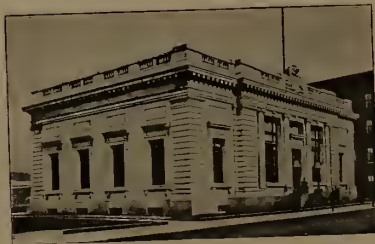
HOLYOKE POST OFFICE.
