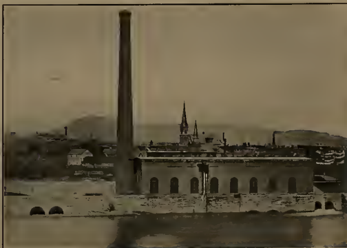
HOLYOKE WATER POWER COMPANY'S ELECTRIC PLANT
