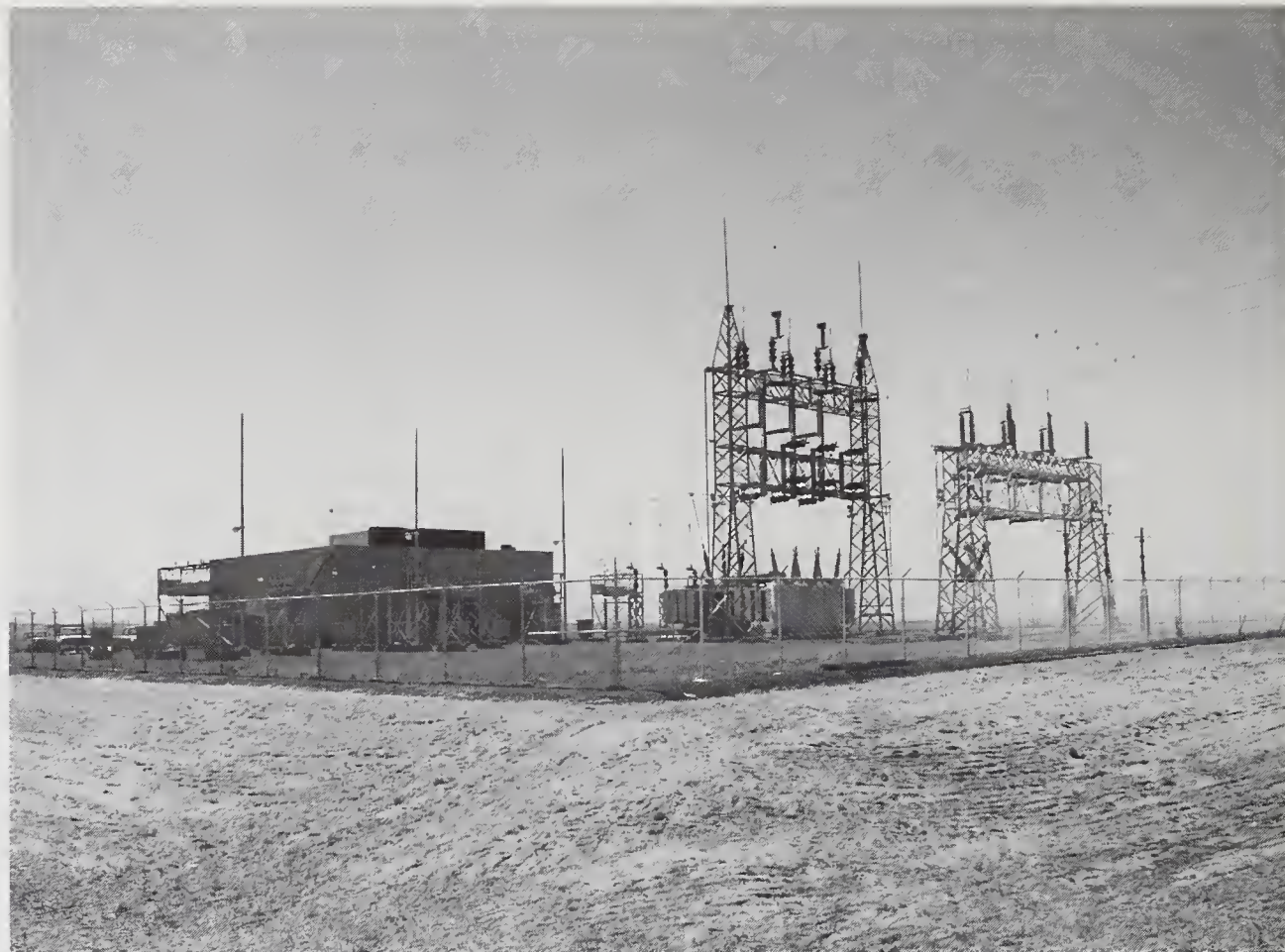
A report on energy use management explores a variety of methods for reducing peak demand and energy costs for rail transit systems.
