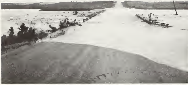
Road and Bridge Flooding
