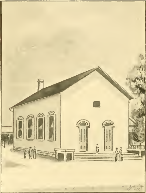
NEW GERMAN BAPTIST CHURCH, SPENCER TOWNSHIP, LUCAS COUNTY, OHIO.
