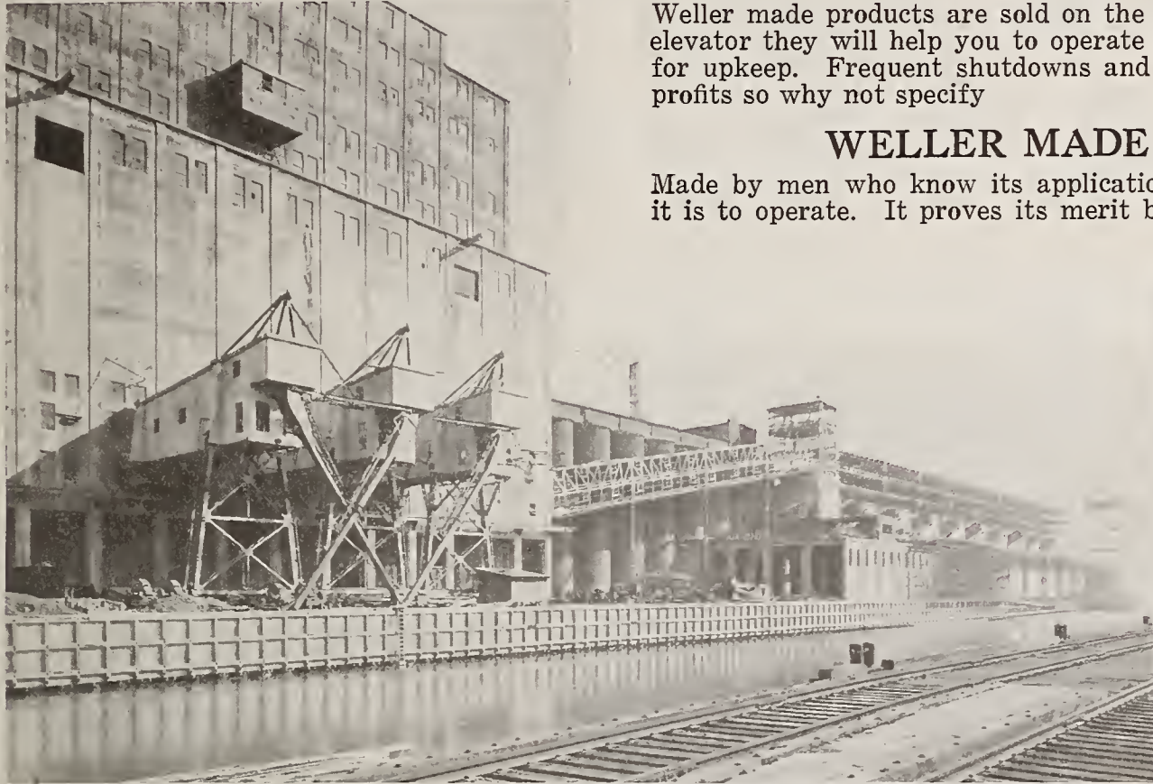
NORTHERN CENTRAL ELEVATOR, BALTIMORE, MD.
