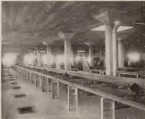
VIEW OF THE GALLERY OVER STORAGE BINS
