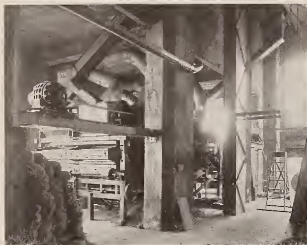
EAST BAY OF MAIN FLOOR WITH CLEANERS
