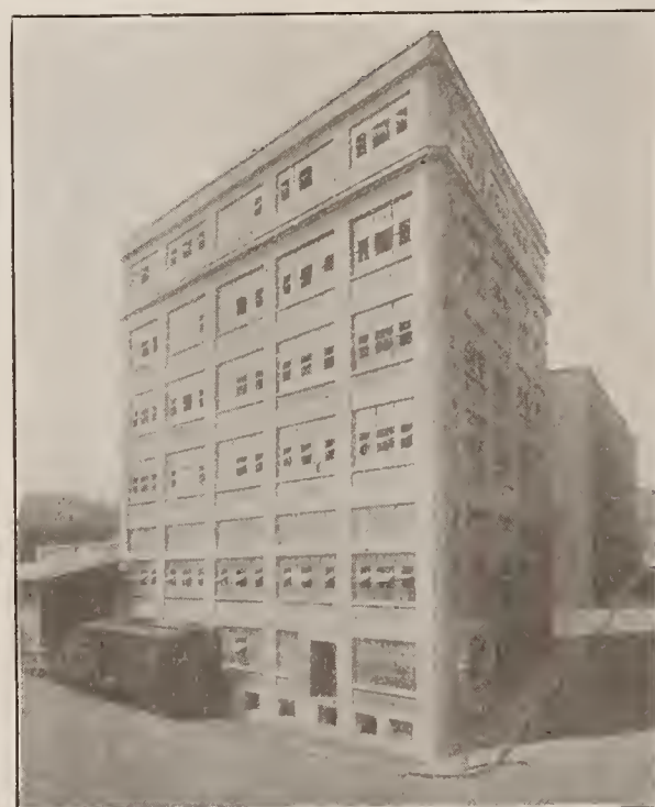
Reinforced Concrete Flour Mill with 50,000 bu. Grain Storage erected for the Wilkins Rogers Milling Co., Washington, D. C.
