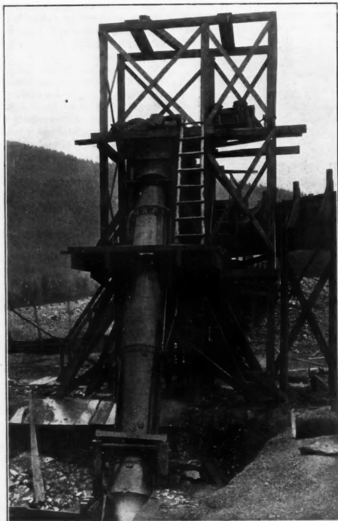
HYDRAULIC ELEVATOR ON AN OREGON MINE.
