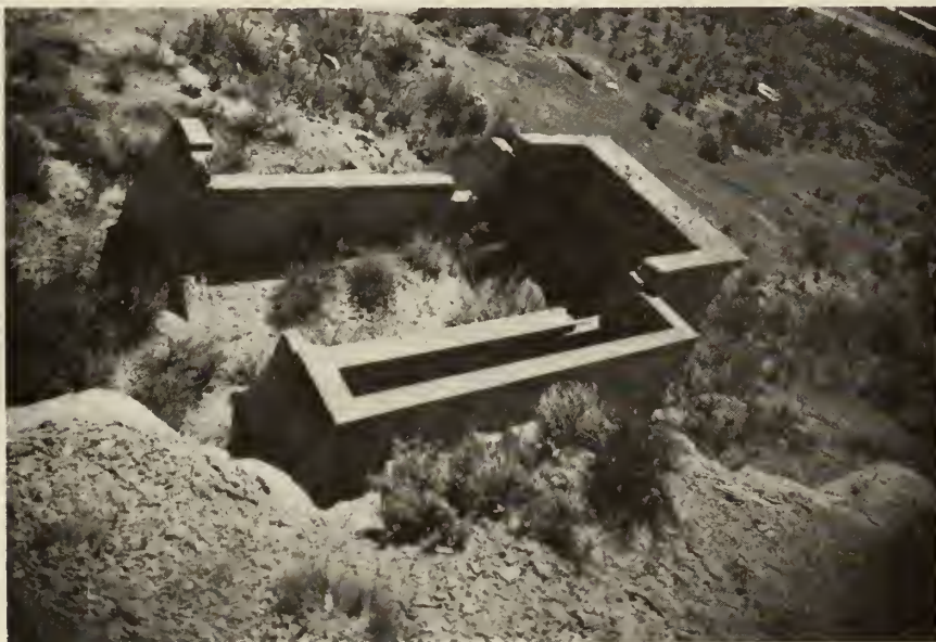
The Forebay structure of the Havemeyer-Willcox Canal is what remains today. Historic American Engineering Record Photo by F.J. Athearn
