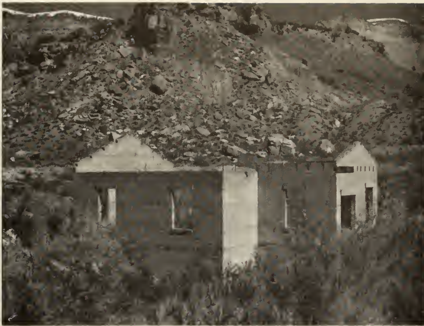
The Havermeyer-Willcox Canal was one of the boldest ventures in the state for providing water to beet fields. In 1980 all that remained was this pumphouse. Historic American Engineering Record Photo by F. J. Athearn
